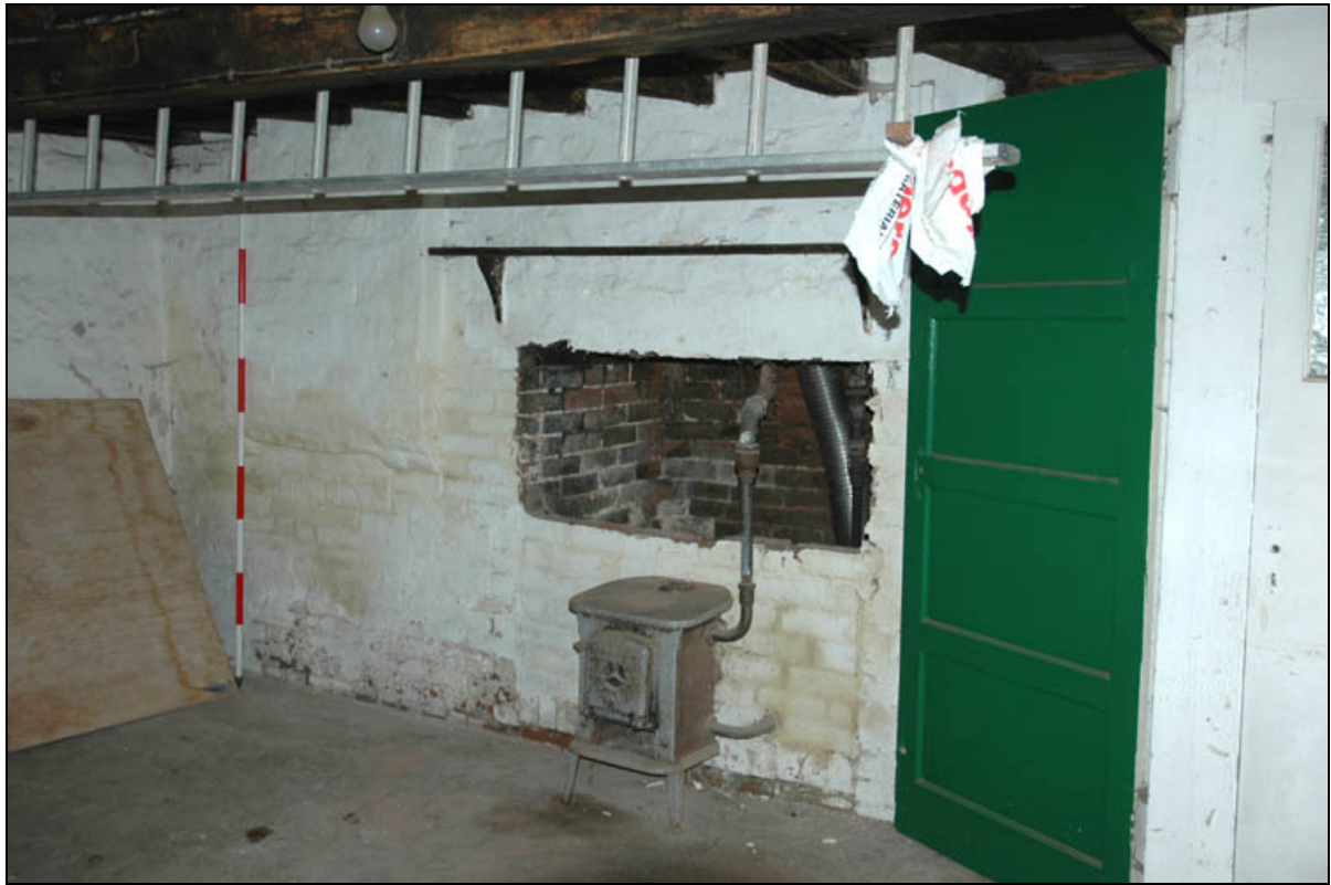
Plate 20: Fireplace in 18 th century extension with bread oven to immediate right of scale
