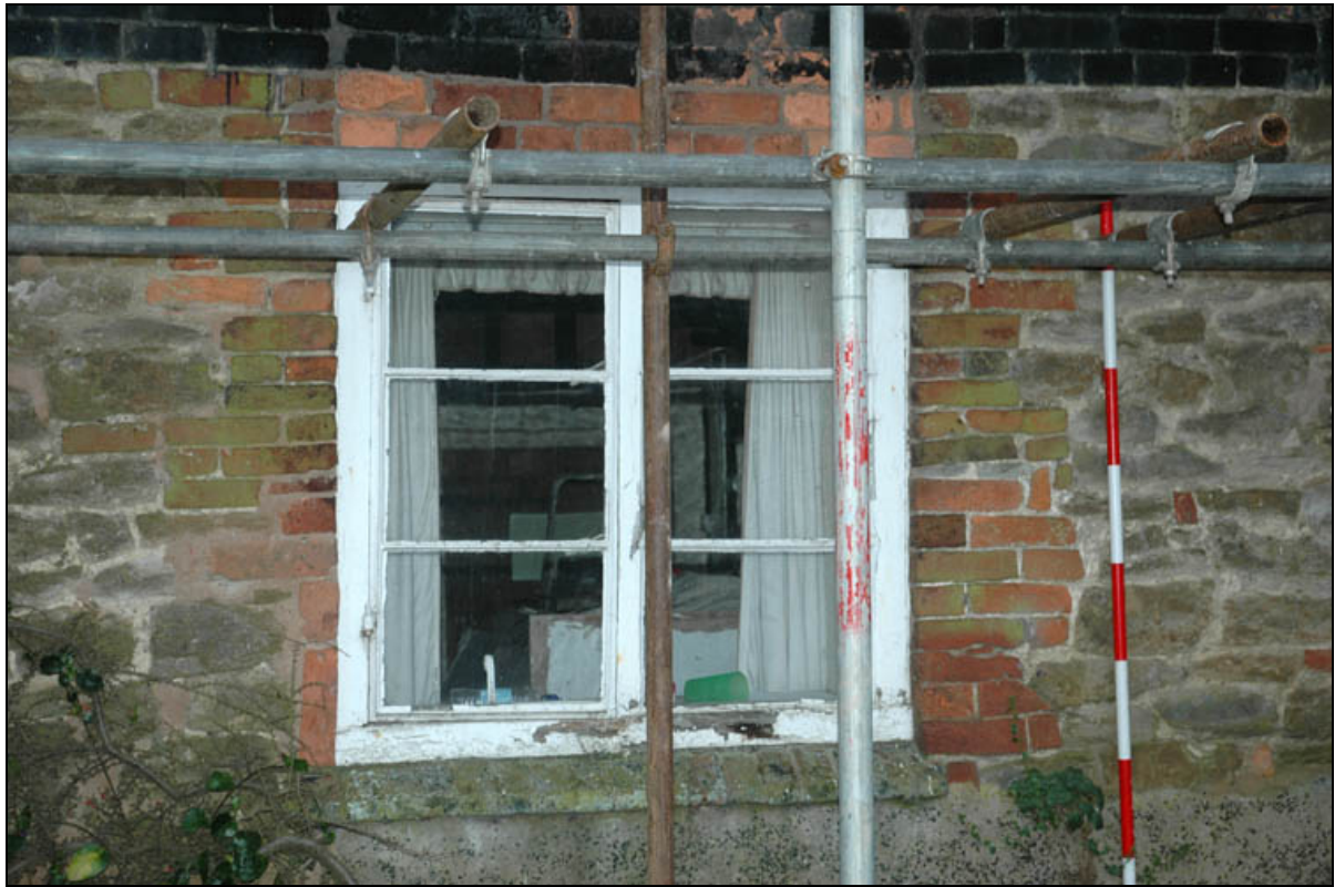
Plate 16: Blocking of hall window
