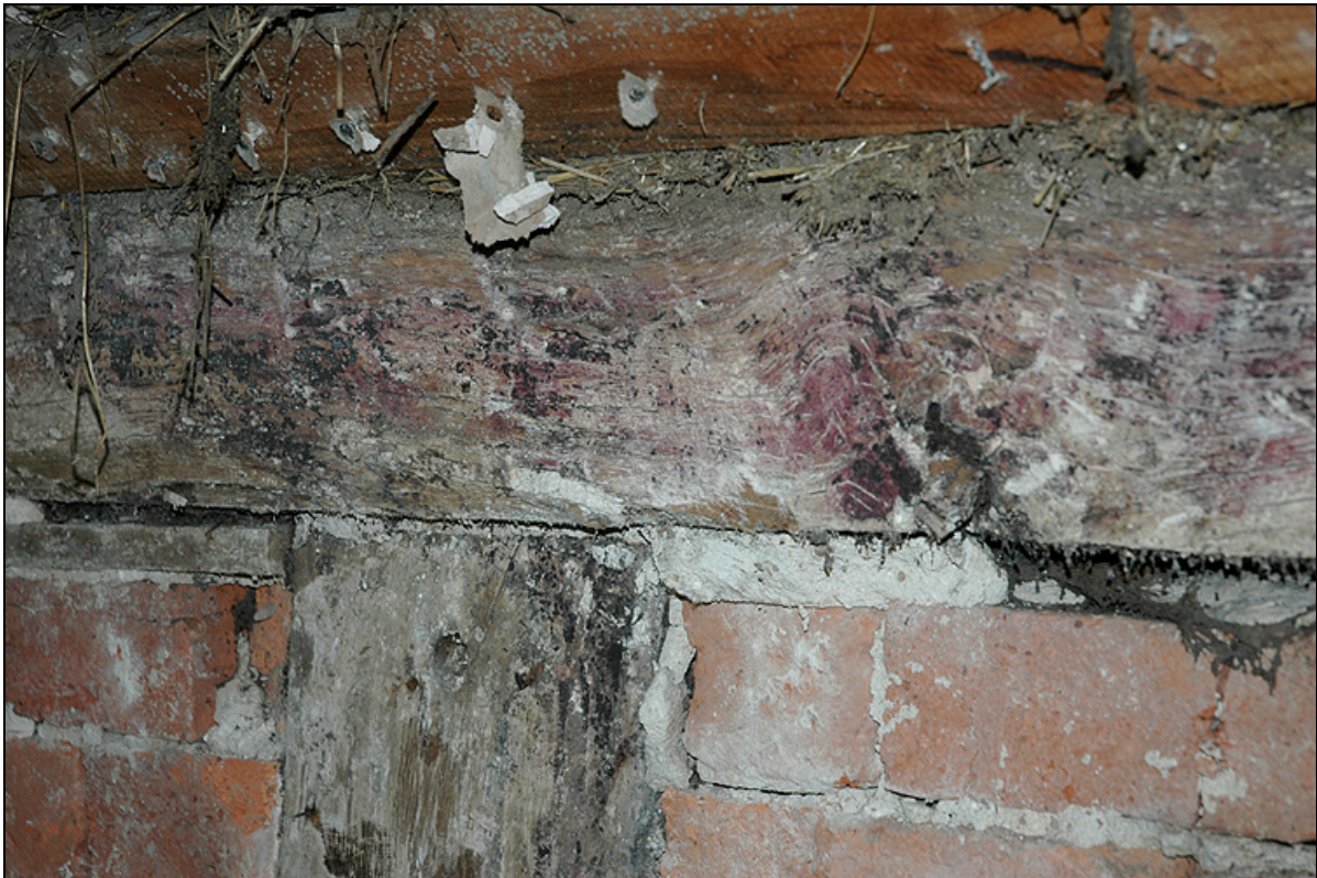
Plate 9: Magenta paint on timbers in room F8
