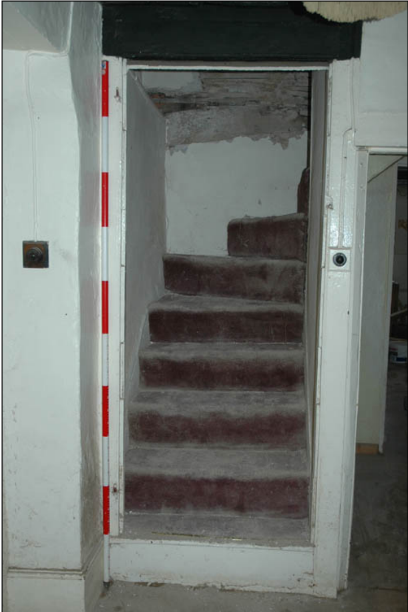
Plate 15: Straight flight with winder staircase inserted in to cross passage
