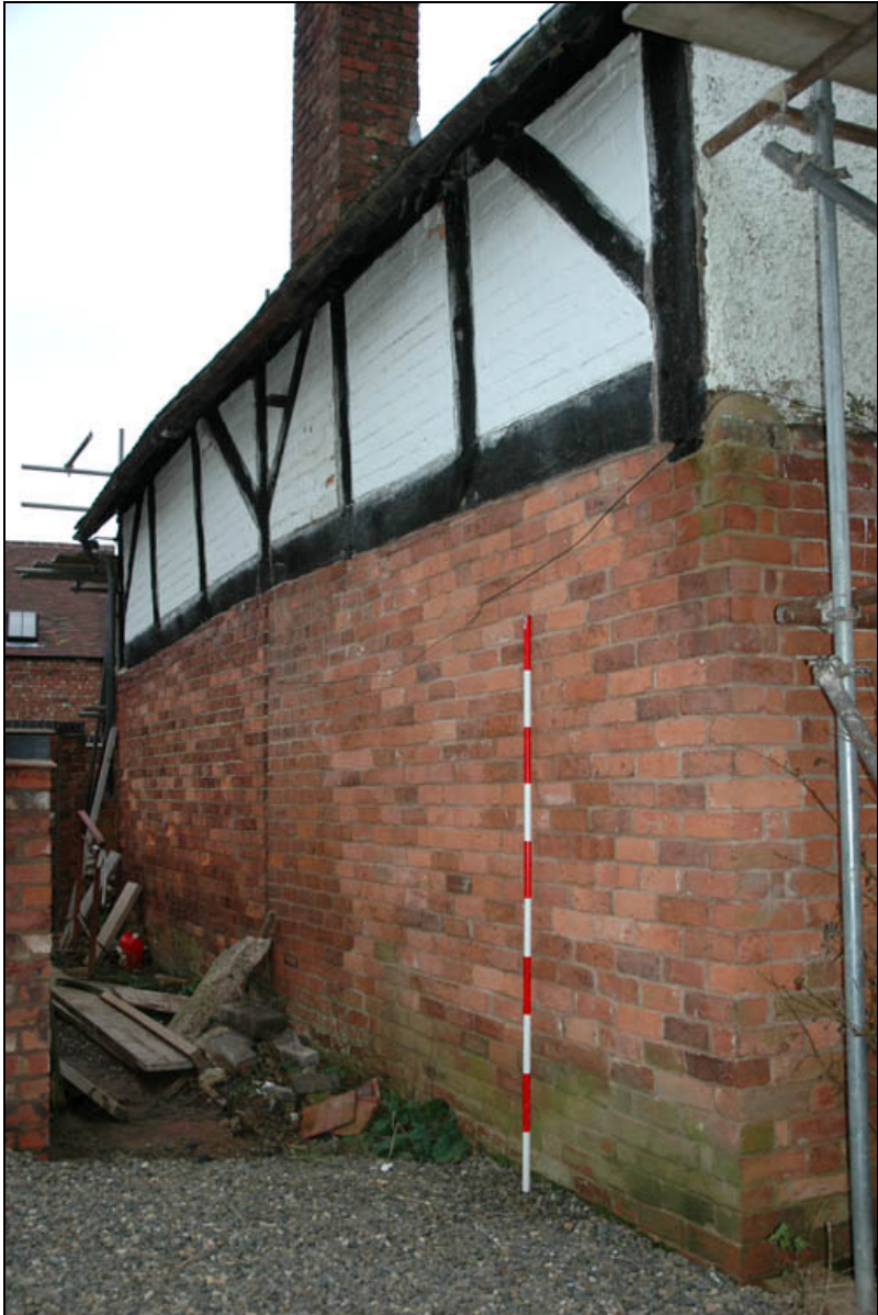
Plate 25: West elevation 19 th century ground floor rebuild (right)
