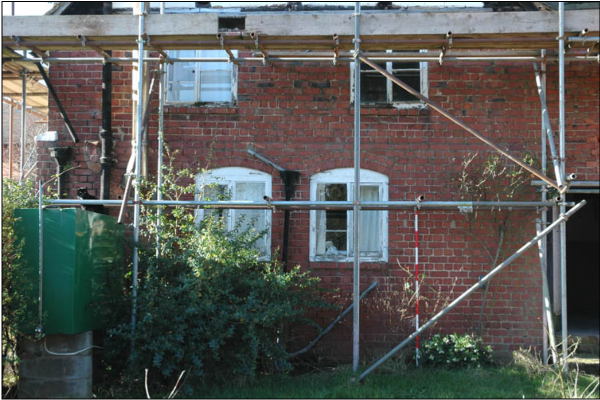
Plate 24: East elevation 19 th century rebuild
