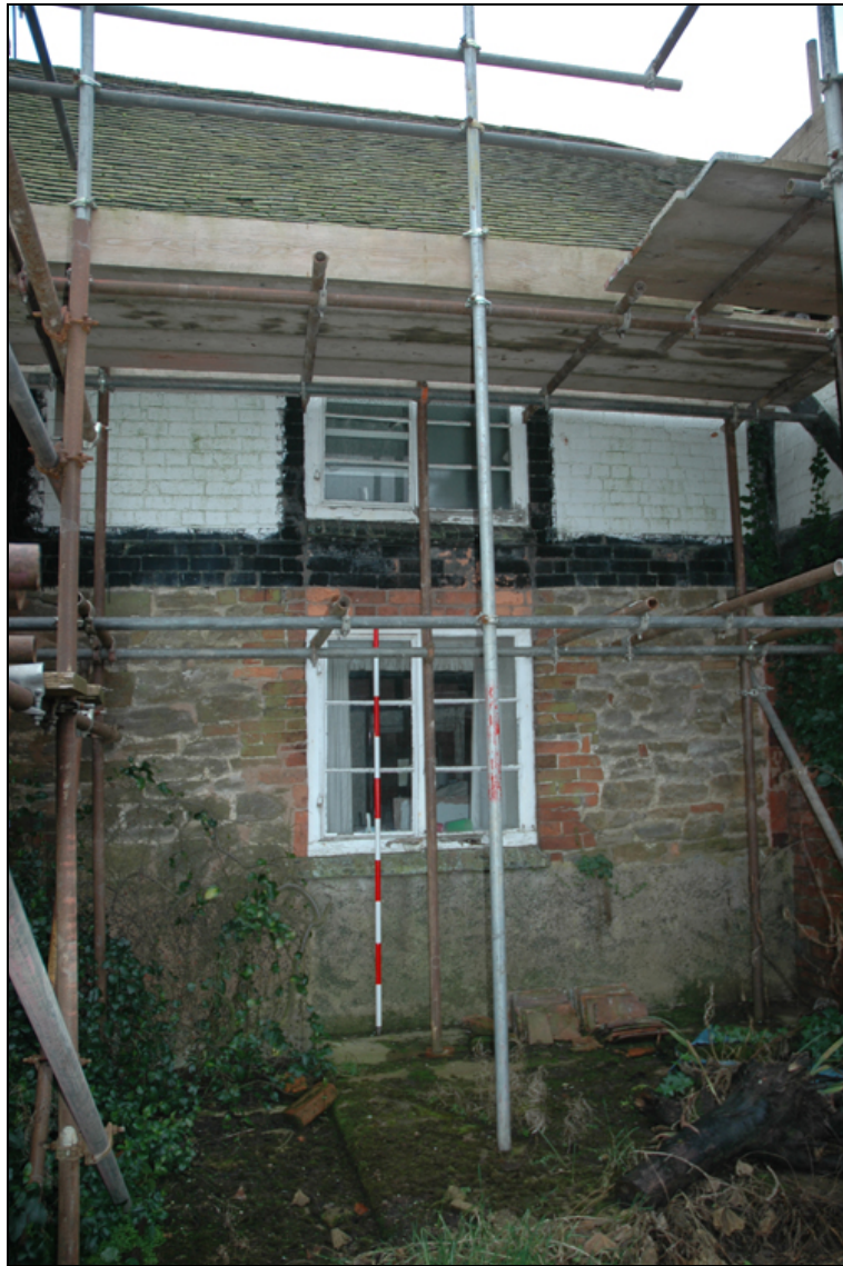
Plate 7: Position of hall window in north east wall of building
