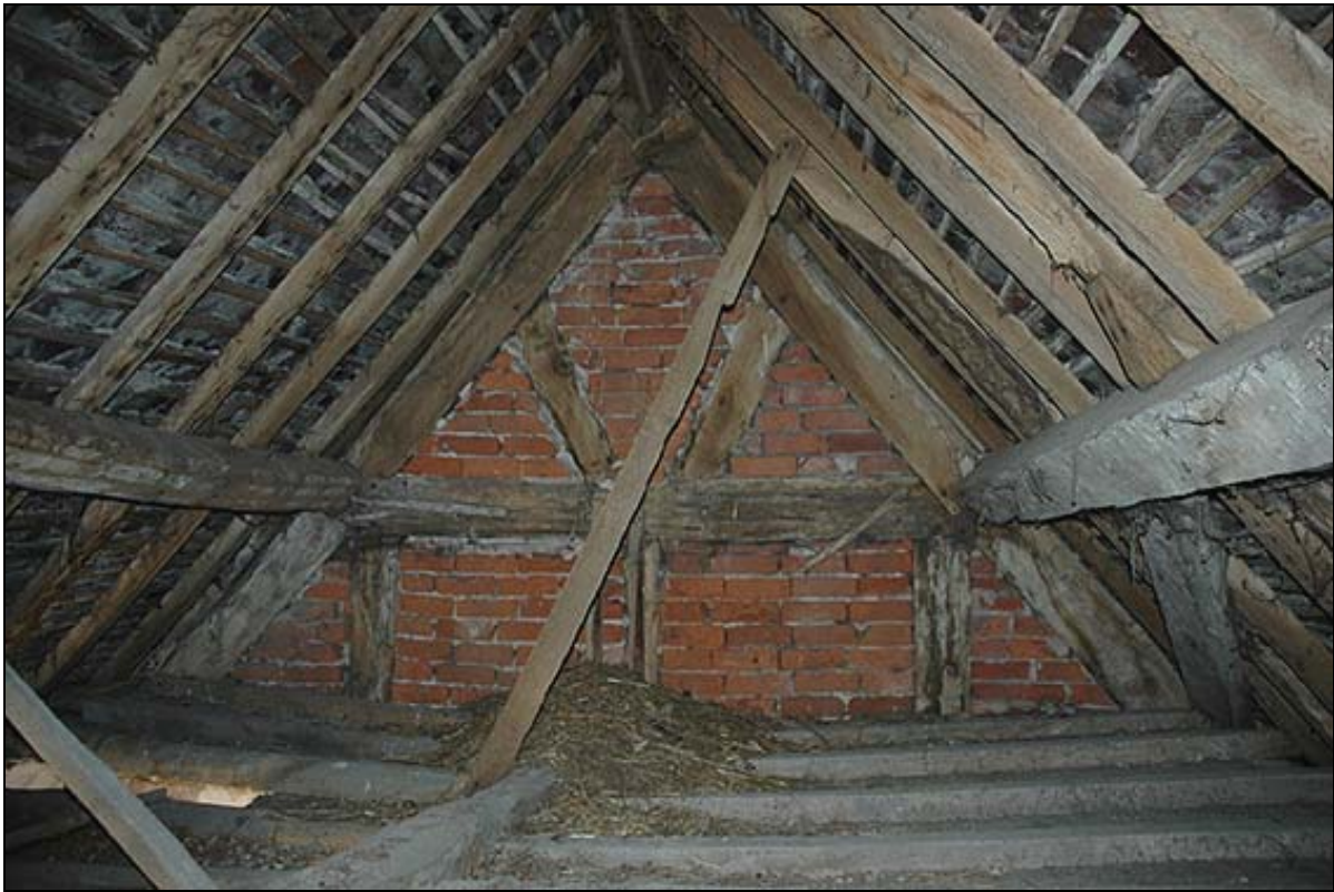
Plate 5: V-struts above collar, roof space of cross-wing
