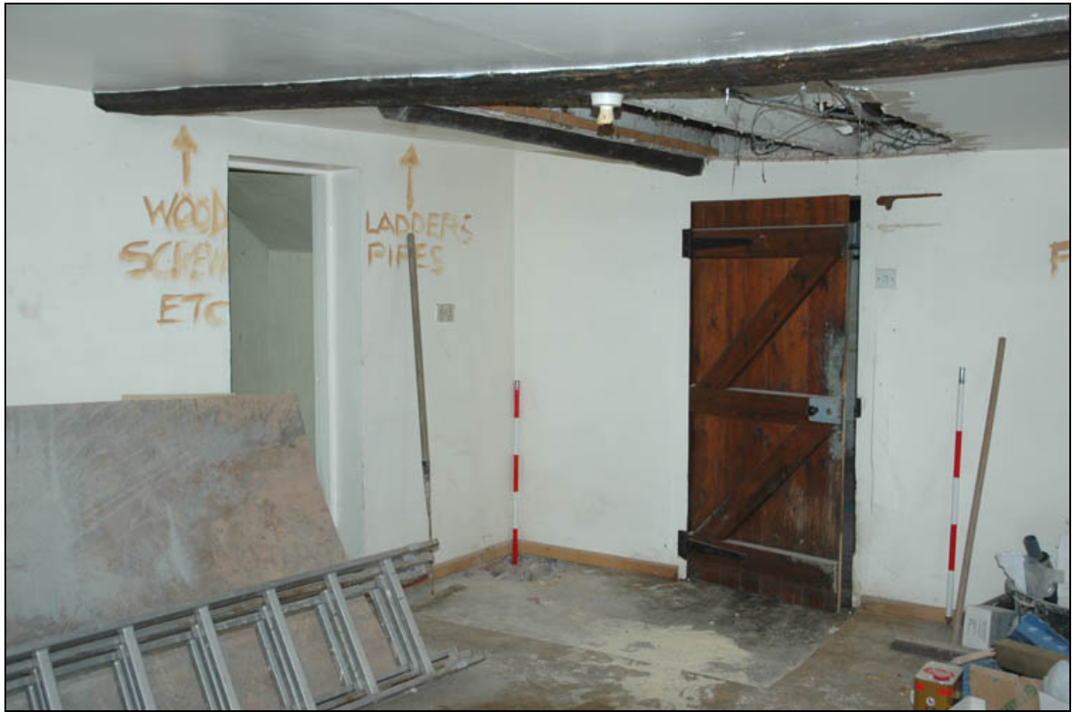
Plate 14: Ceiling beams in room G2 showing possible staircase position
