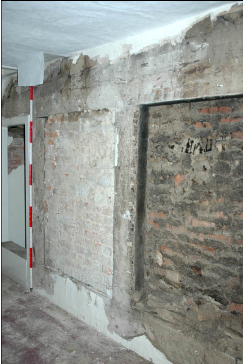
Plate 13: part of timber-frame wall behind chimney stack
