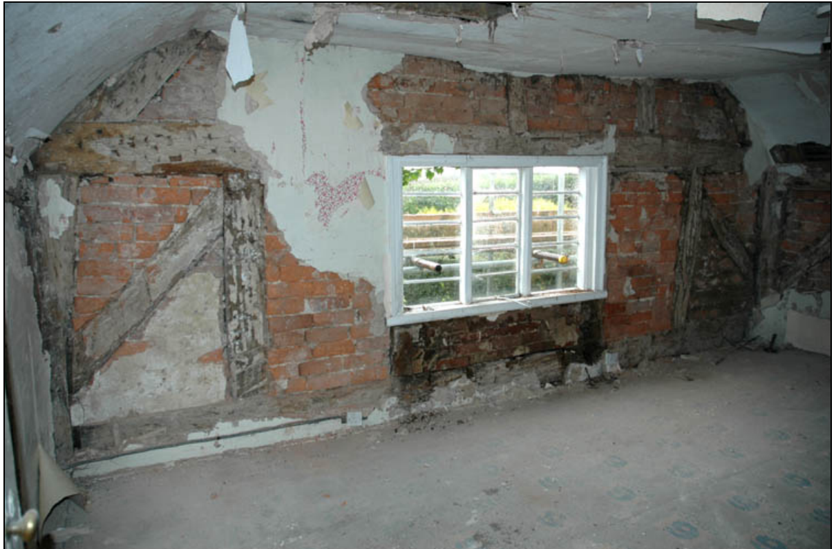
Plate 4: Revealed timber frame in room F8 (see also Fig 6)
