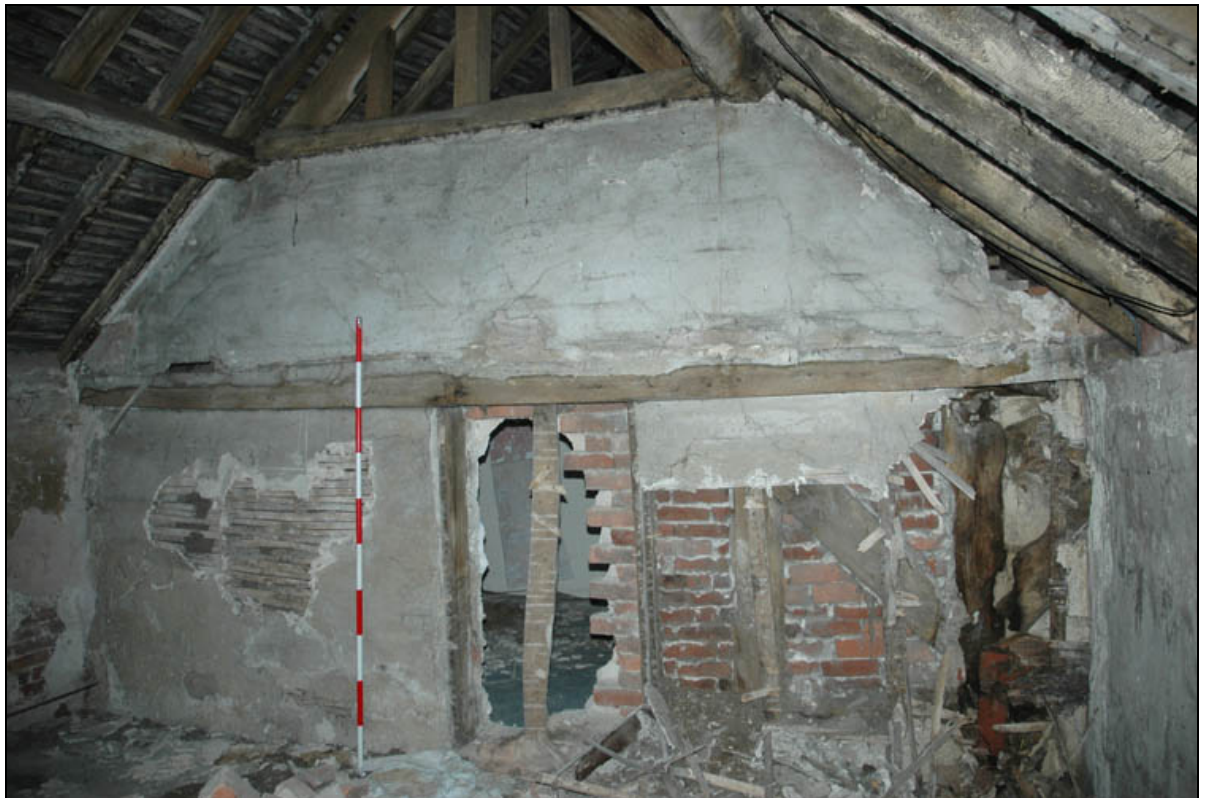
Plate 21: Party wall between 18 th century extension and 16 th service wing
