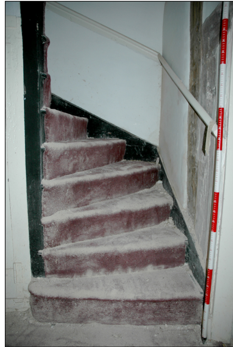
Plate 8: Original staircase position in room G7
