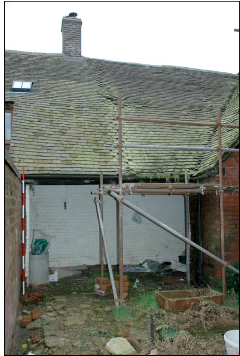
Plate 31: Cat slide roof on porch
