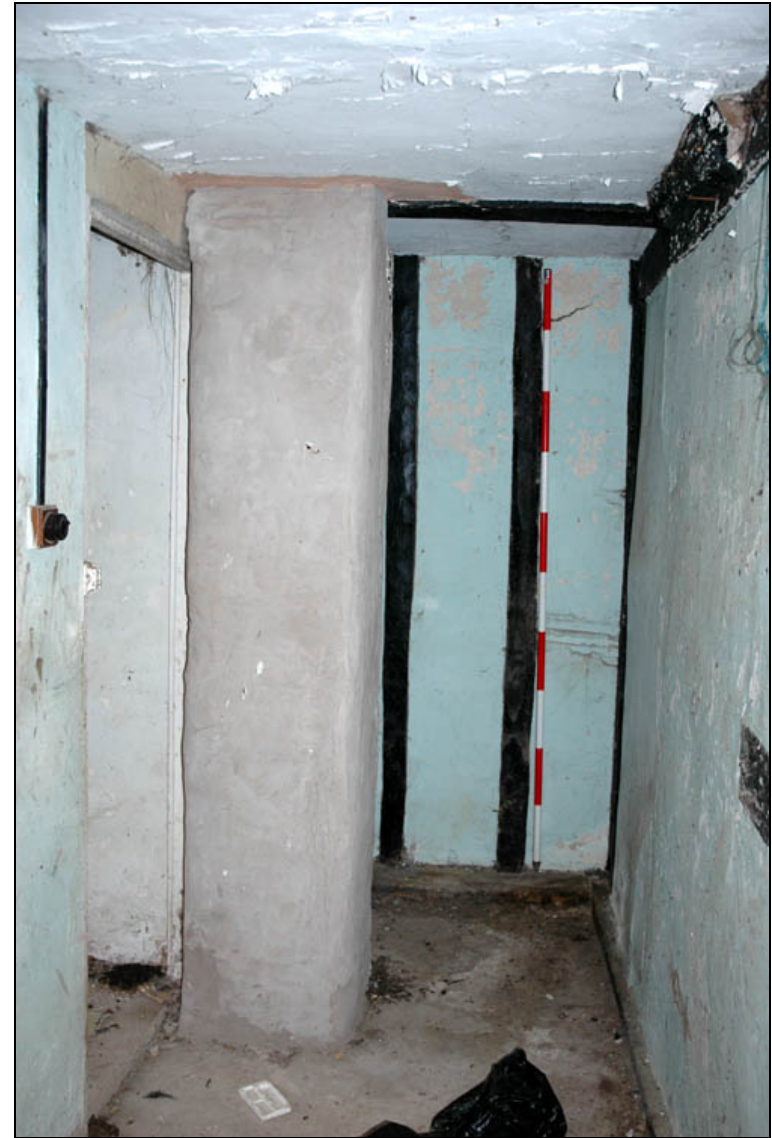
Plate 28: Timber cellar stairs partition wall
