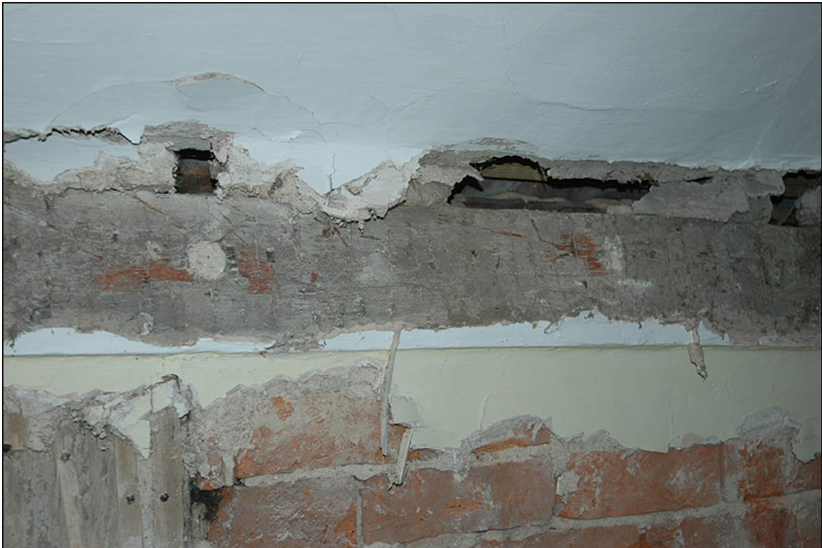
Plate 10: Red paint on timbers in room F9
