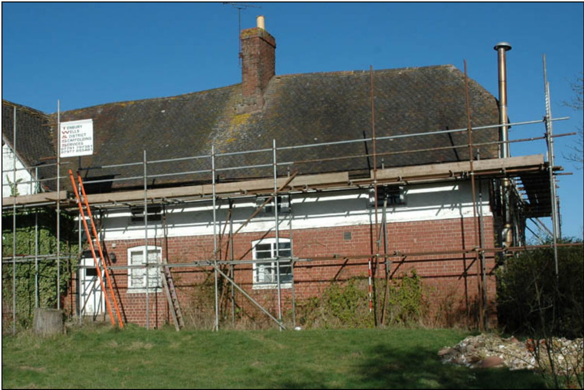
Plate 23: South elevation, ground floor 19 th century rebuild
