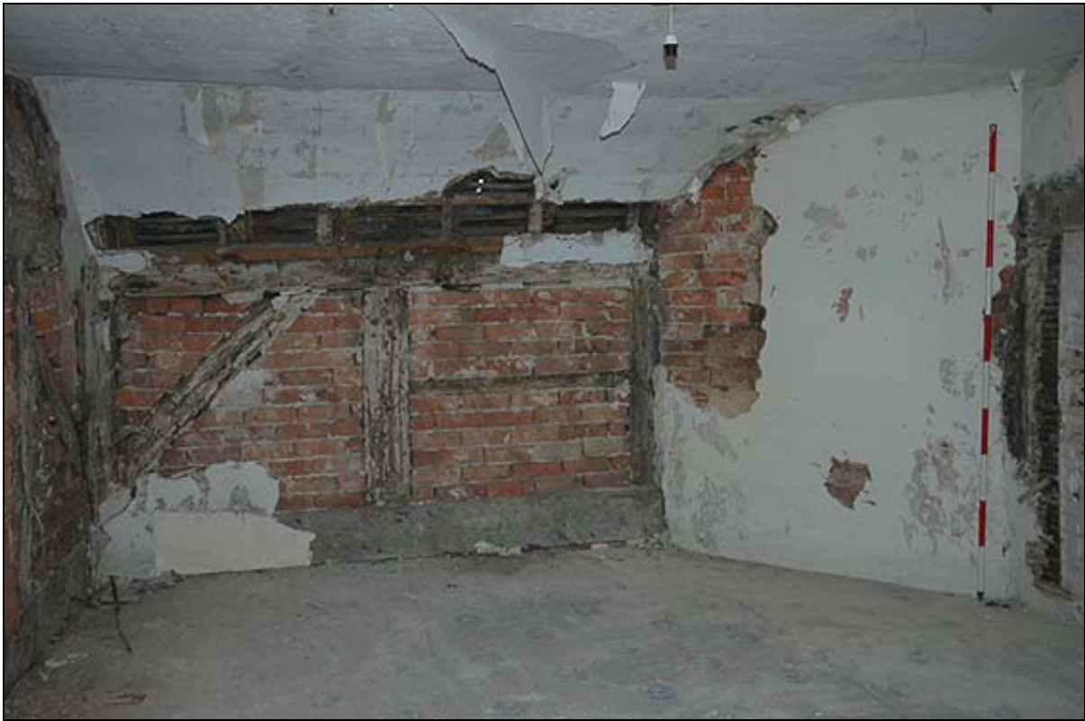
Plate 6: Timber frame panels and up brace
