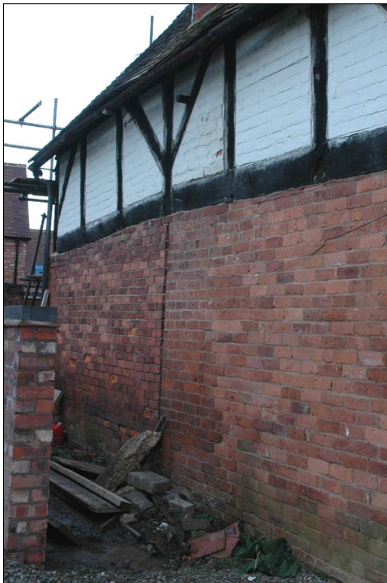
Plate 22: 18 th century (left) rebuild of west elevation ground floor
