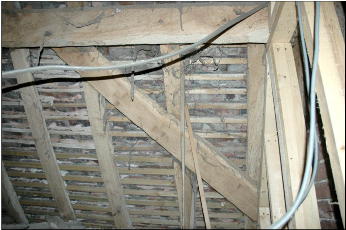
Plate 11: Wind brace in roof space of cross-wing
