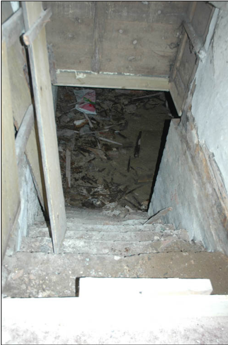
Plate 27: Stairs to cellar
