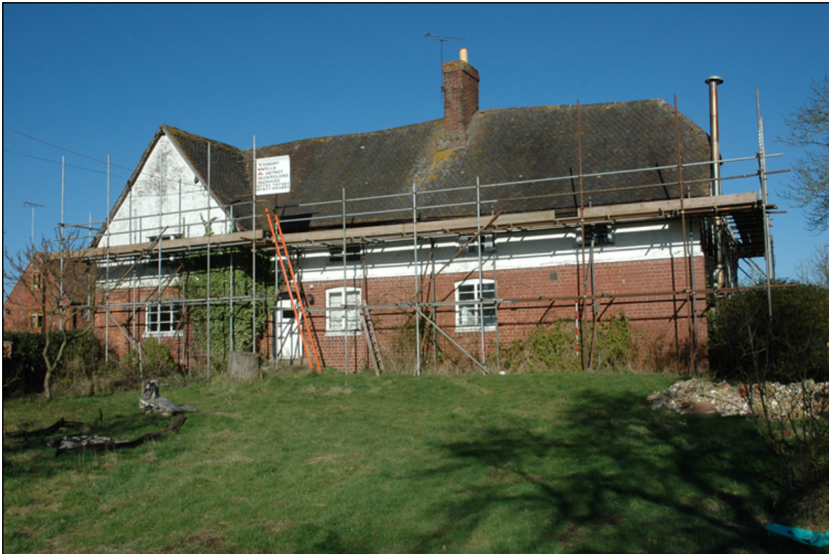
Plate 1: Plowstall Farmhouse south west elevation
