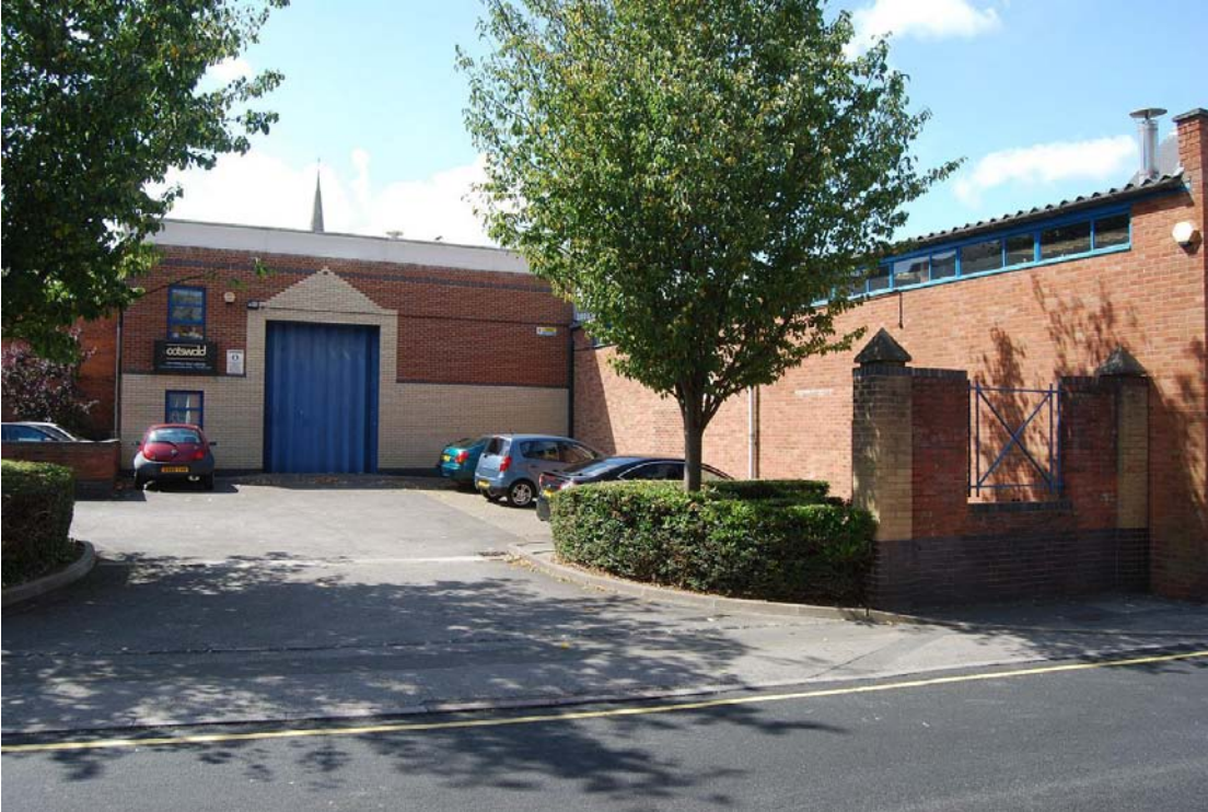
Plate 3: Cotswold Golf Ltd factory and car park, from Alvin Street, looking north-west
