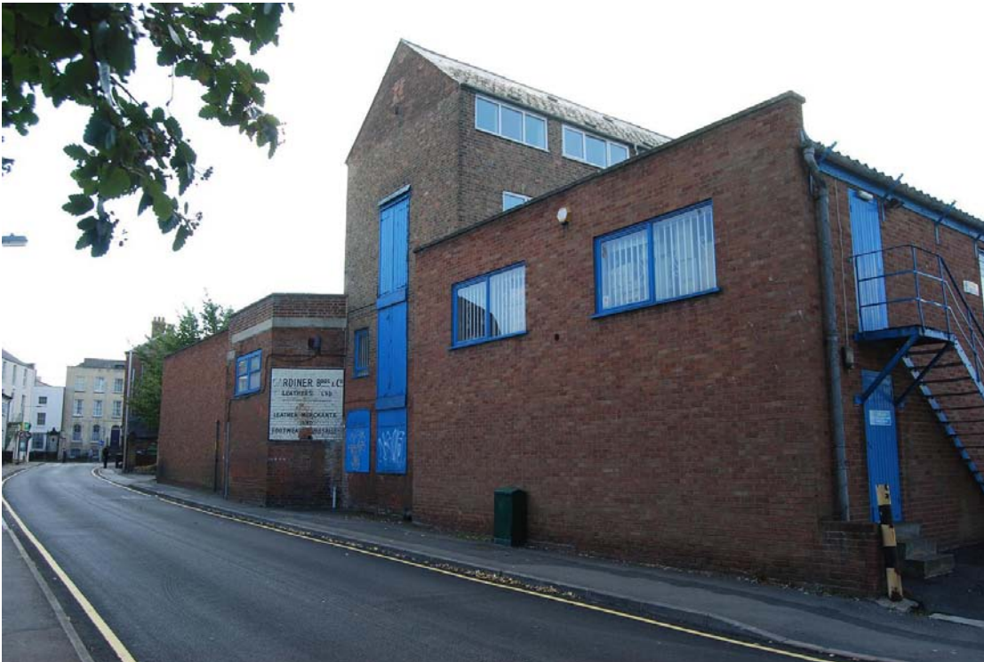
Plate 1: Gardiner Bros and Co (Leather) Ltd factory, from Alvin Street, looking south-west
