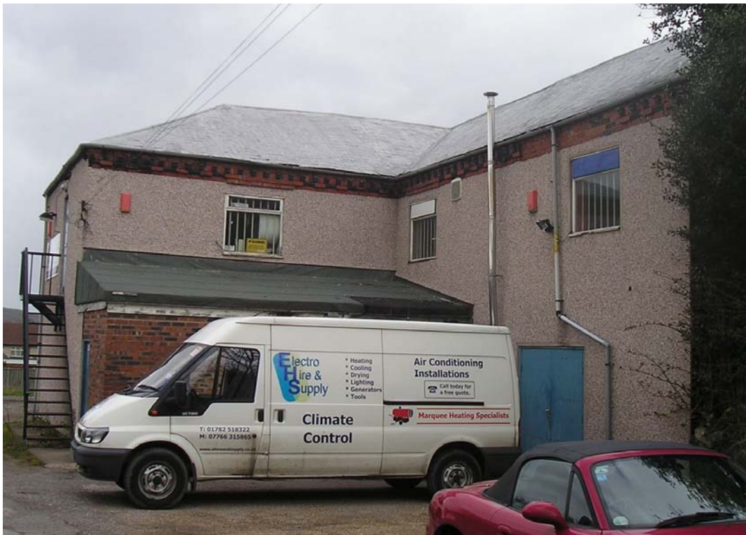
Plate 6, Workshop in the centre of site occupied by Electro Hire and Supply
