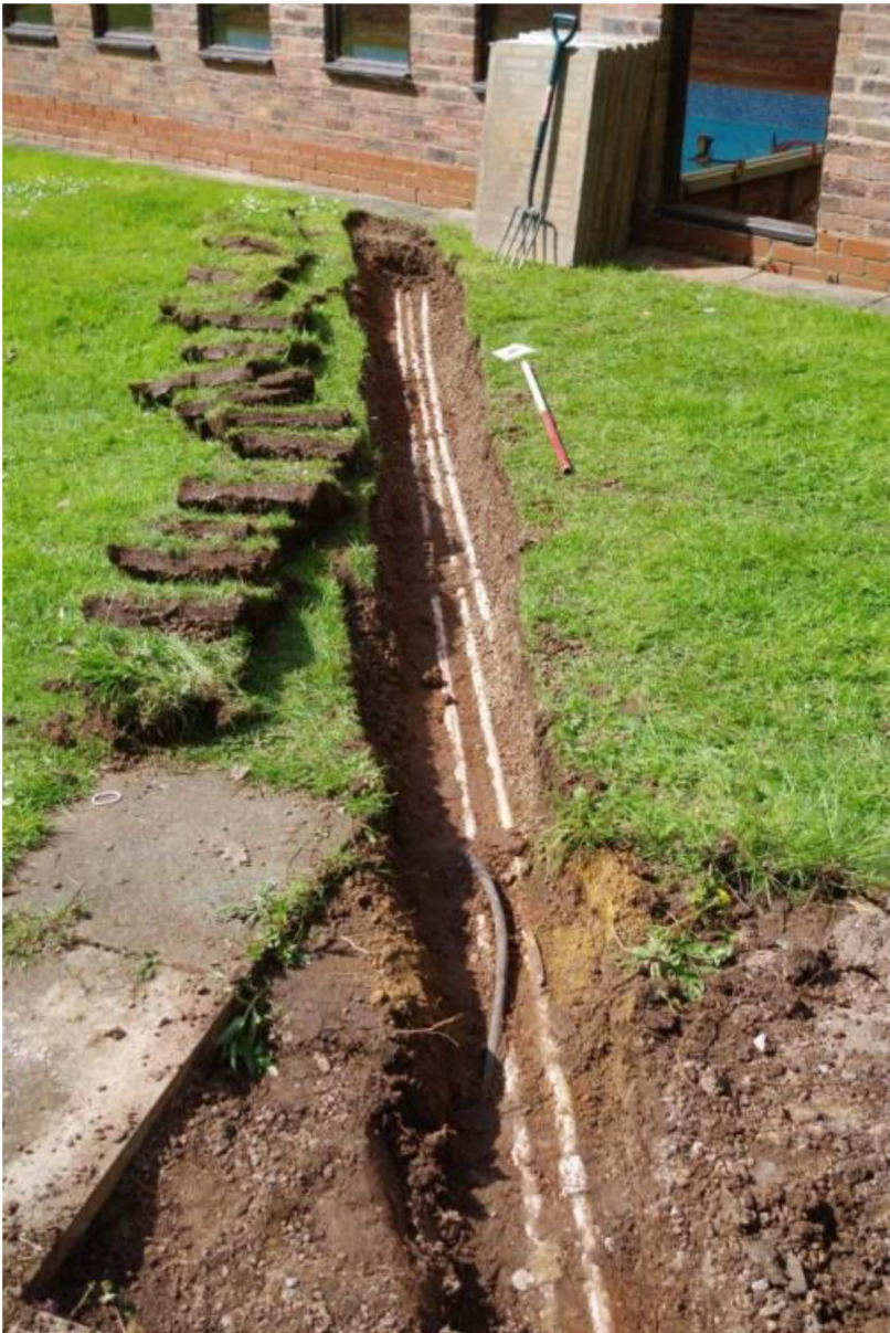
Plate 2 Trench 2 excavated, view north-west, 1m scale
