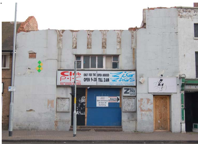
Figure 5: Zig Zags after demolition in March 2008
