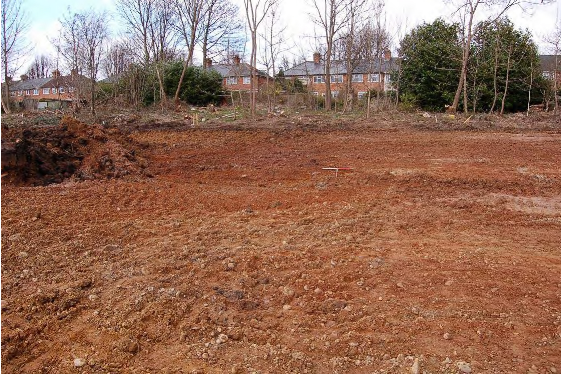
Plate 3 Natural sands and gravels exposed during groundworks, facing North-west
