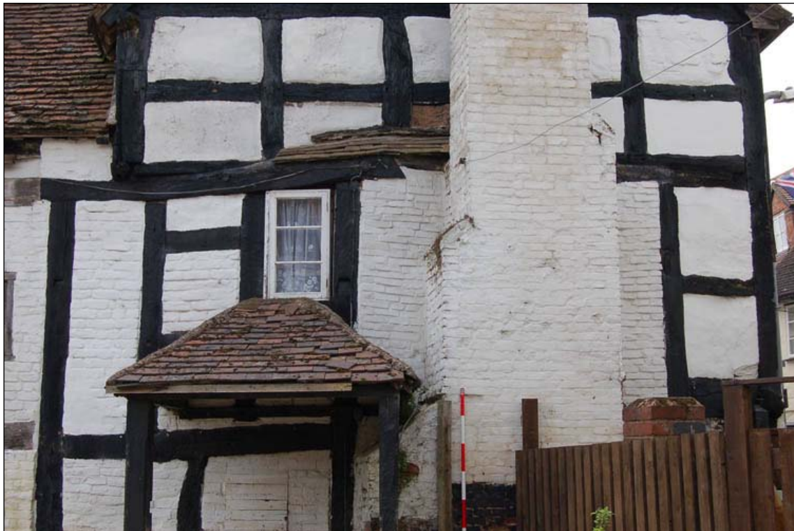
Plate 21: Chimney stack against north gable
