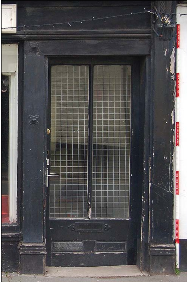
Plate 40: Pilasters on 1 Court Street shop front
