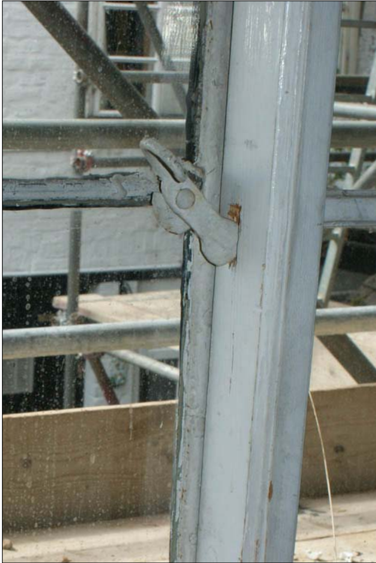
Plate 31: 18 th century turnbuckle catch
