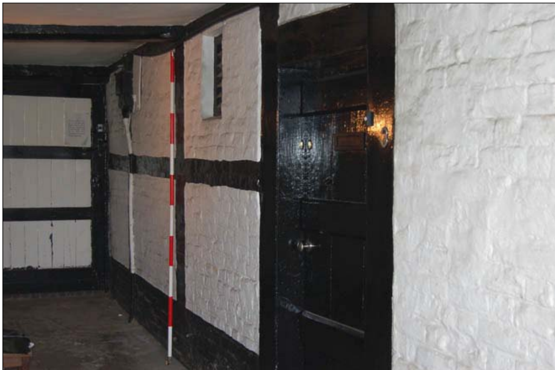
Plate 37: 18 th century rebuilt passageway wall
