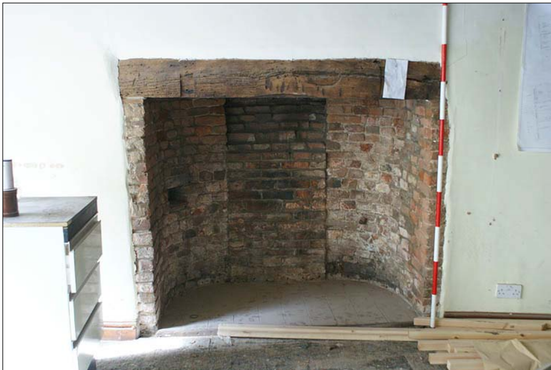
Plate 22: 18 th century fireplace in room G5
