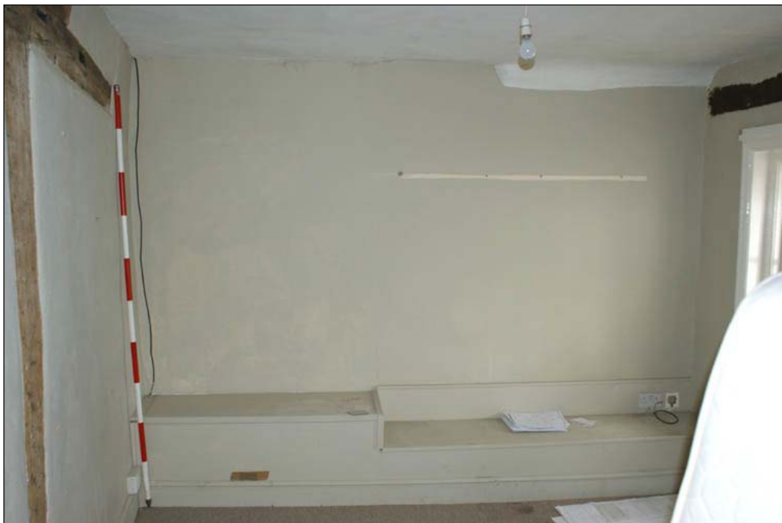
Plate 35: 3 Court Street, 18 th century extension interior
