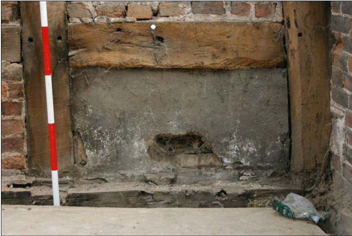
Plate 5: Wattle and daub panel in Attic 1b
