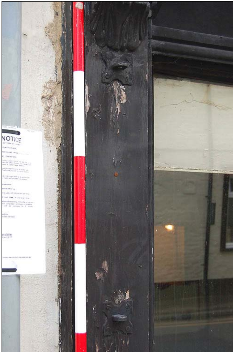
Plate 42: Fixing eyes for awning or bars
