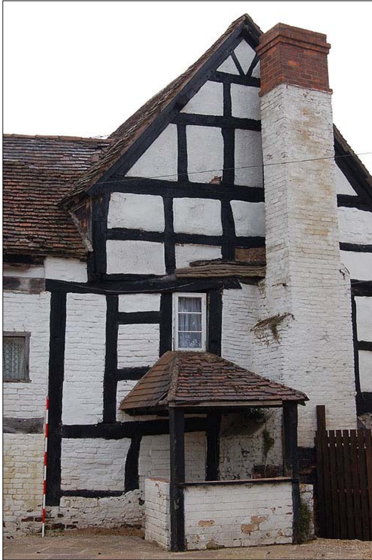
Plate 11: Partly rebuilt north gable
