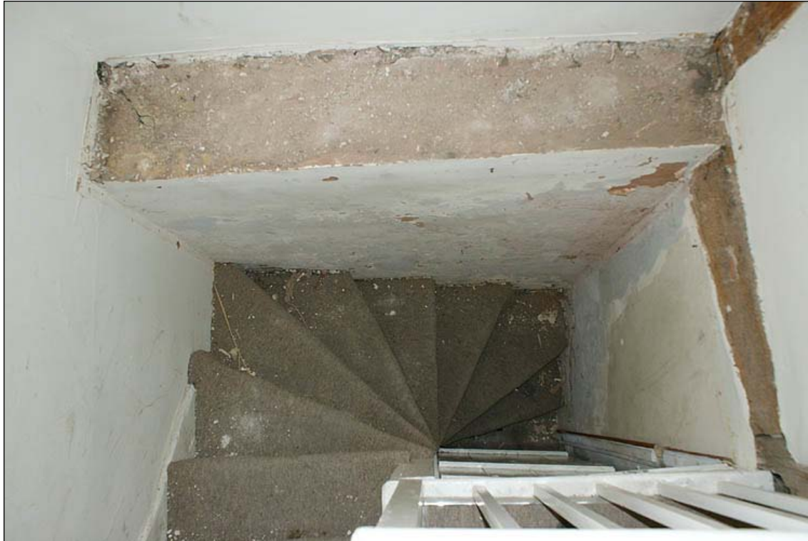
Plate 36: 3 Court Street, 18 th century winder staircase
