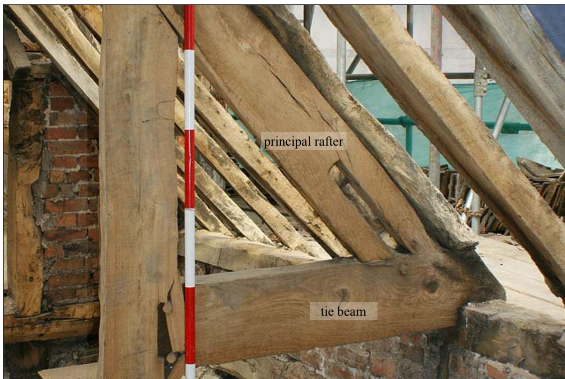
Plate 49: 17 th century roof truss showing tie beam and principal rafter
