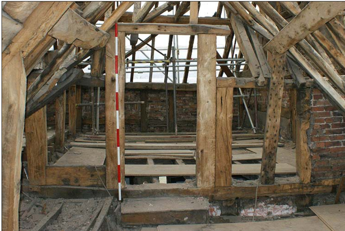
Plate 29: Inserted doorway and step from attic 2 to attic 1B
