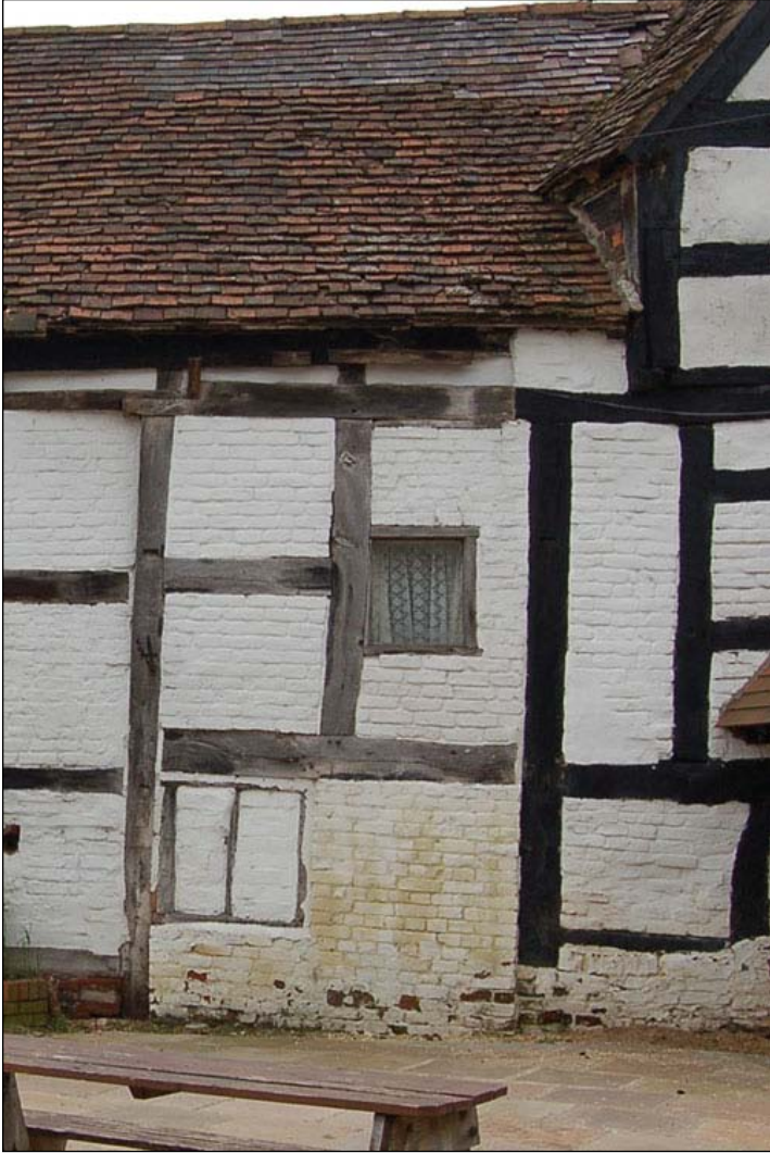
Plate 10: Small extension to rear, east, of main structure
