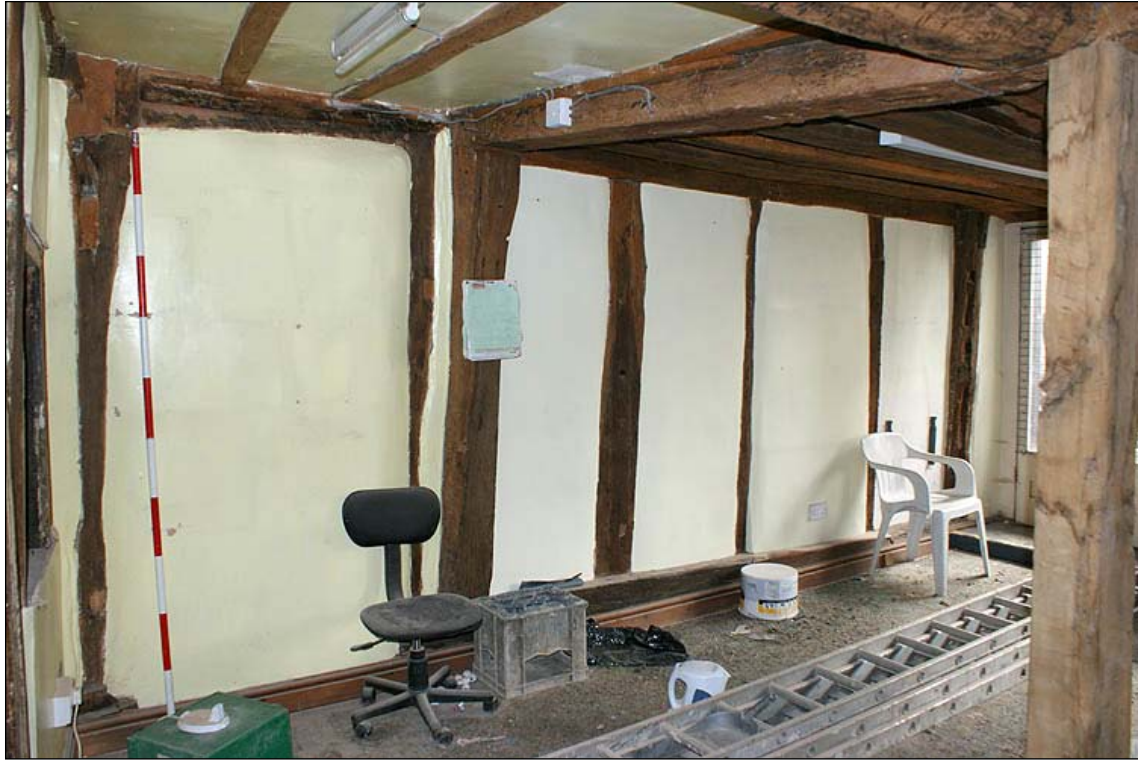
Plate 50: Blocked door on ground floor of 1 Court Street
