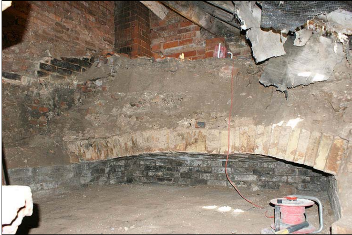
Plate 15: Internal structure of the oven, from south west
