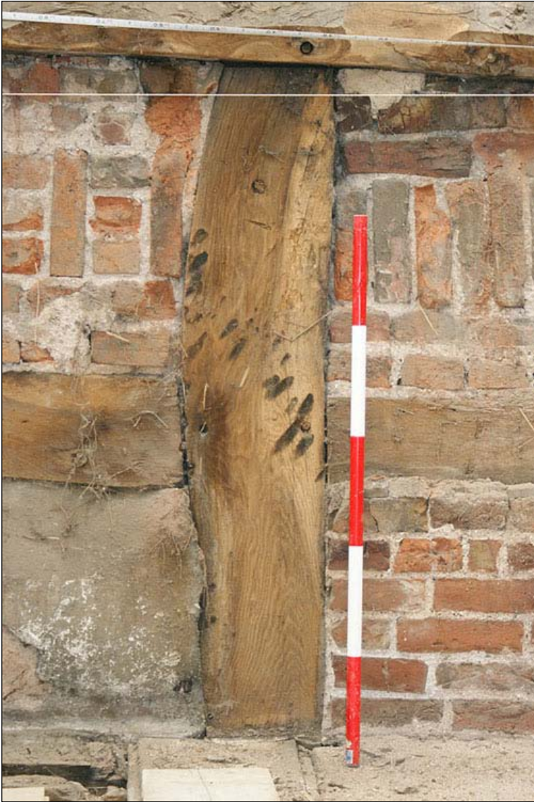
Plate 9: Deliberate burn marks on timbers of Attic 1B gable wall
