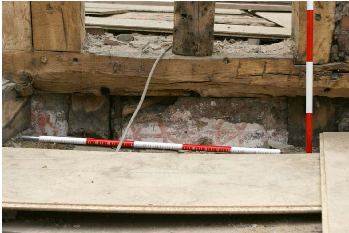
Plate 7: Wall painting, below wall beam, across two infill panels
