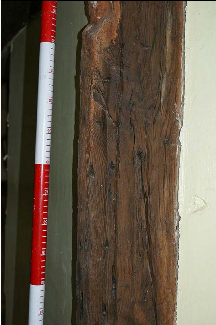
Plate 20: Moulded wood in 18 th century entrance way
