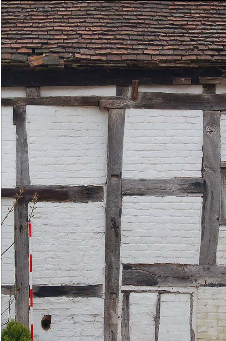
Plate 12: Scarf joint and construction notches
