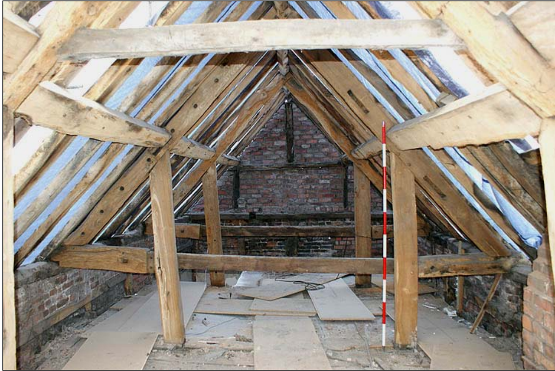
Plate 28: Central roof truss in attic 2
