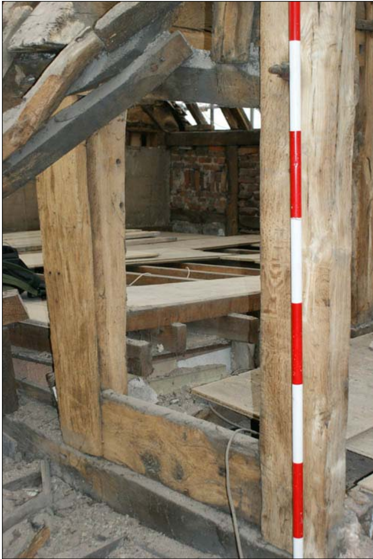
Plate 6: Early weatherboard infill, east wall of attic 1b
