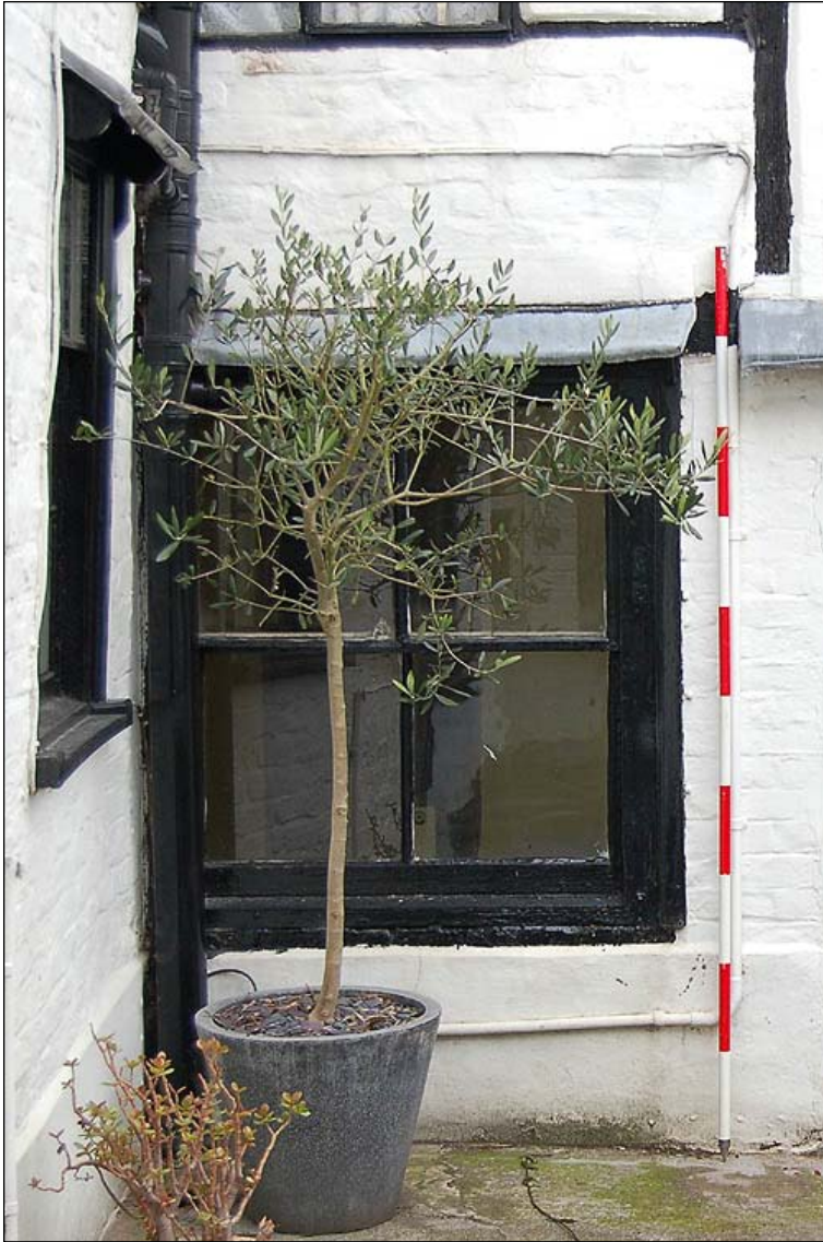
Plate 18: Former 18 th century entrance
