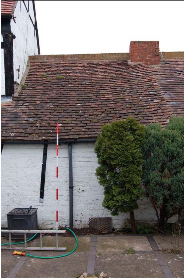
Plate 14: External, south, elevation of bakehouse
