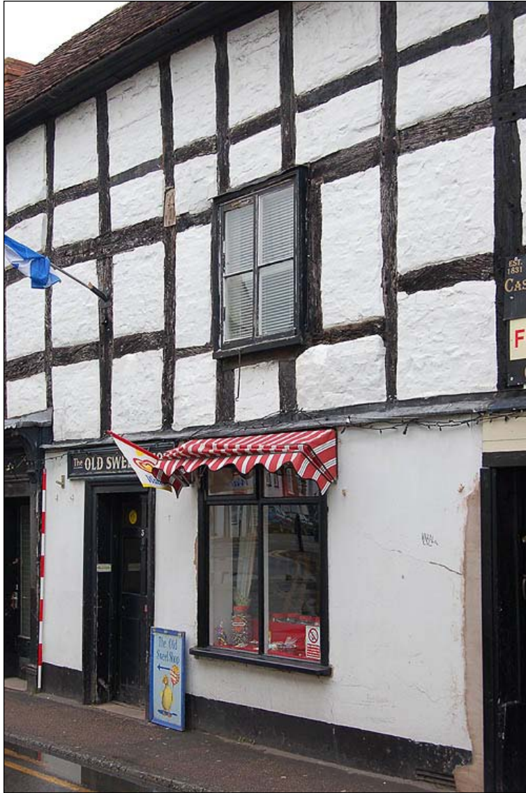
Plate 38: West elevation of 3 Court Street showing brick of infilled jetty
