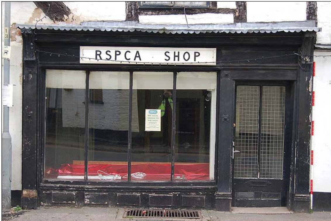
Plate 39: 19 th century shop window of 1 Court Street
