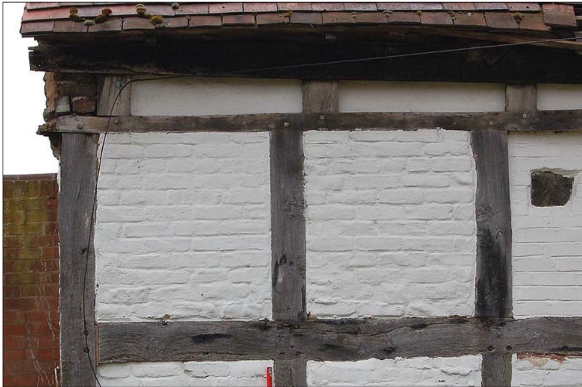
Plate 27: Raised roof line on 17 th century extension
