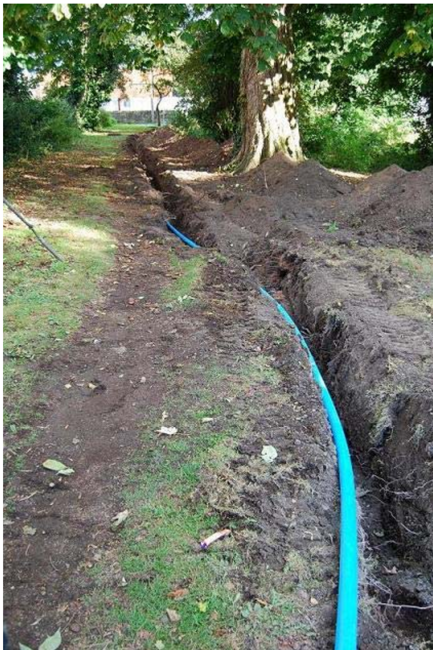
Plate 9: Trench 4 looking south-east
