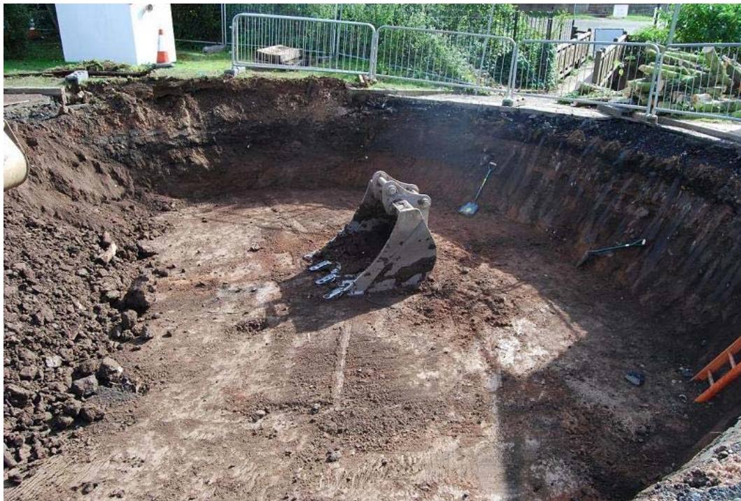
Plate 11: Excavation of the rising shaft, Trench 5, looking south
