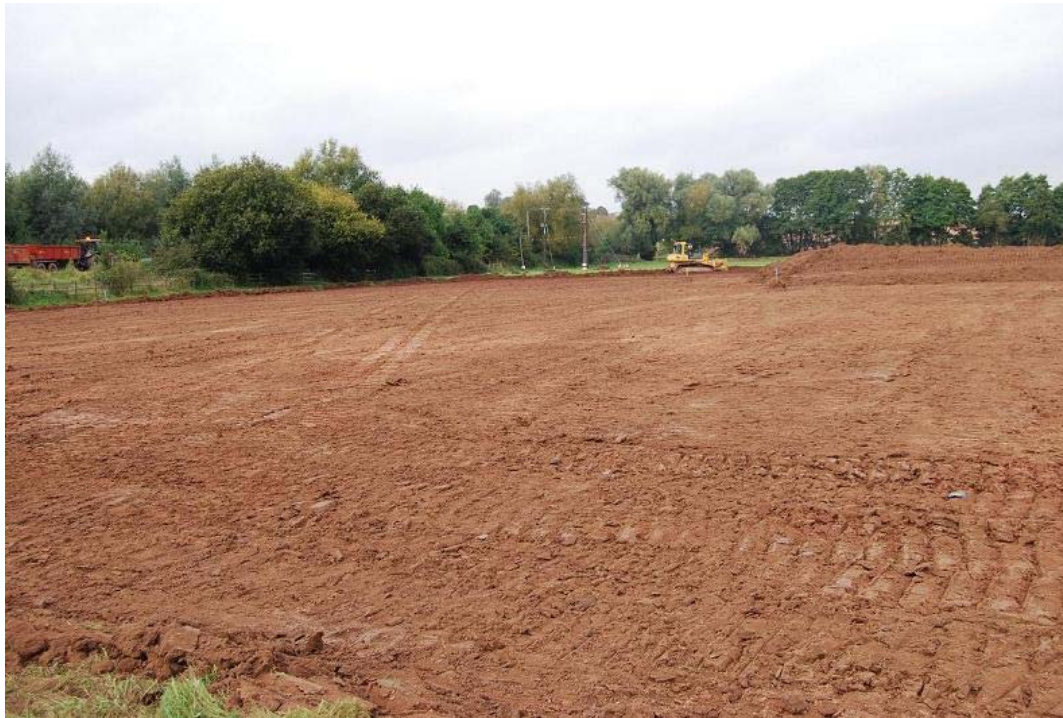
Plate 12: Soil stripping at Marsh Farm, Trench 3, looking north-east.
