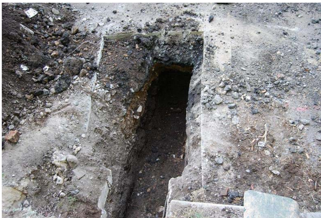
Plate 8: Part of Trench 4 within Homs Road Car Park, looking north.
