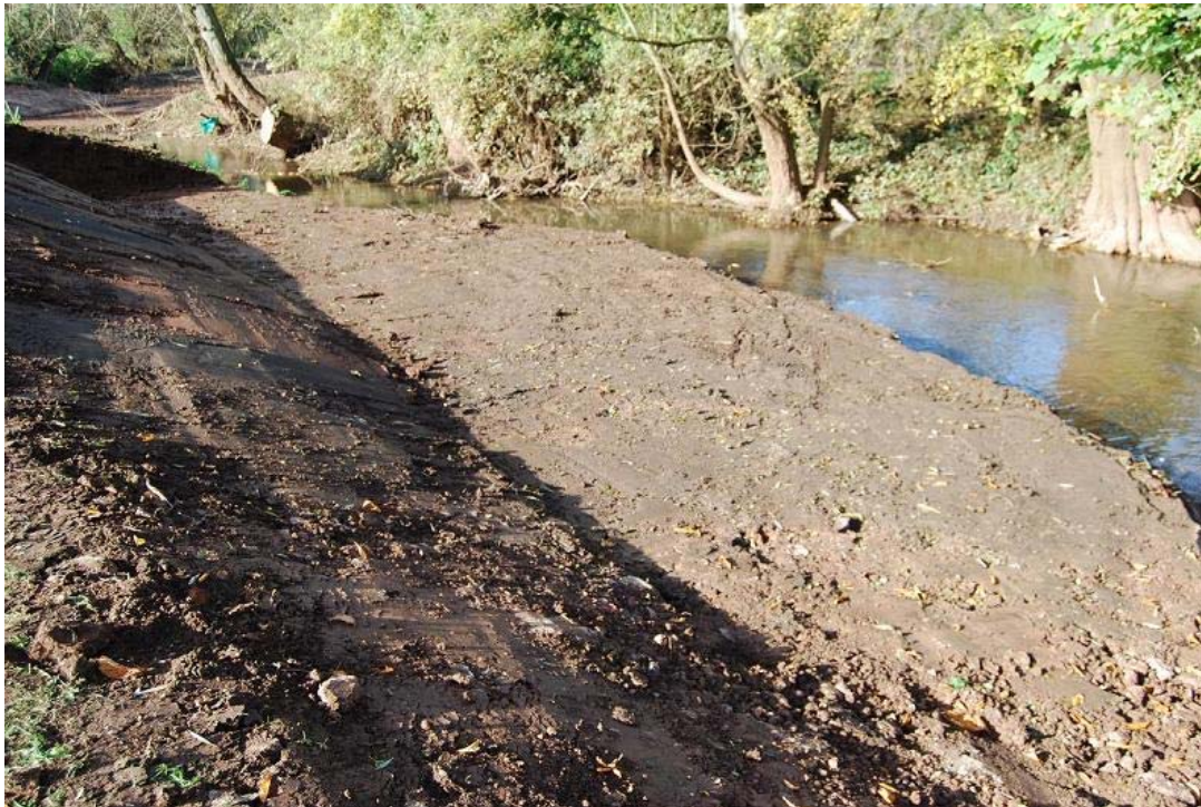
Plate 5: Trench 6 fully excavated, looking west.
