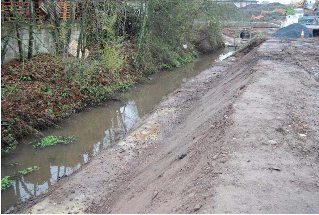
Plate 14: Trench 8 for the Chatterly Brook channel enlargement, looking south-west.
