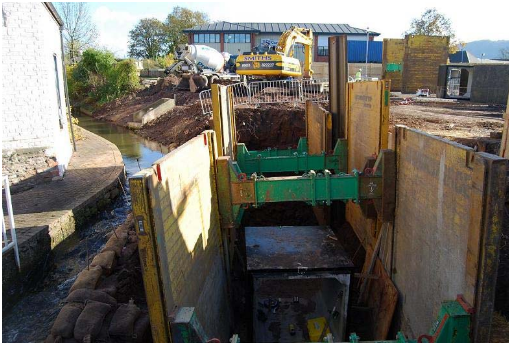
Plate 15: Excavation using box shuttering for the Chatterly Brook channel enlargement.
