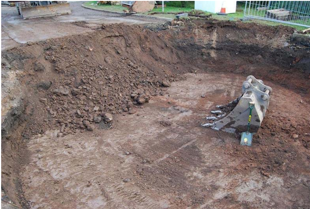
Plate 10: Excavation of the rising shaft, Trench 5, looking east.
