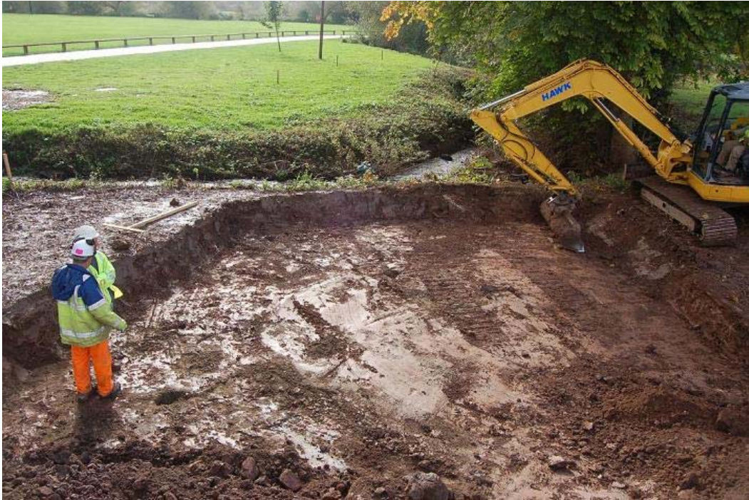
Plate 1: Excavation of Trench 1, looking north.
