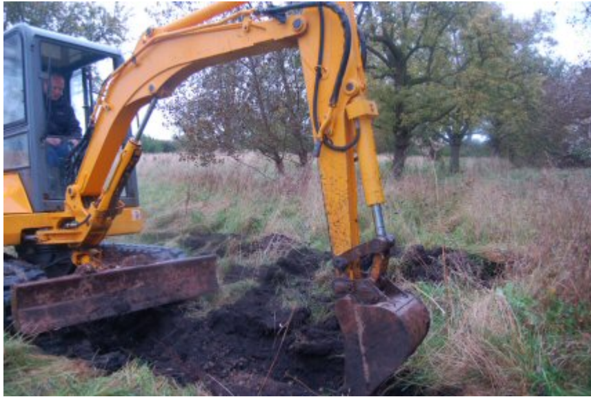
Plate 1: Machine Excavation, Trench 1
