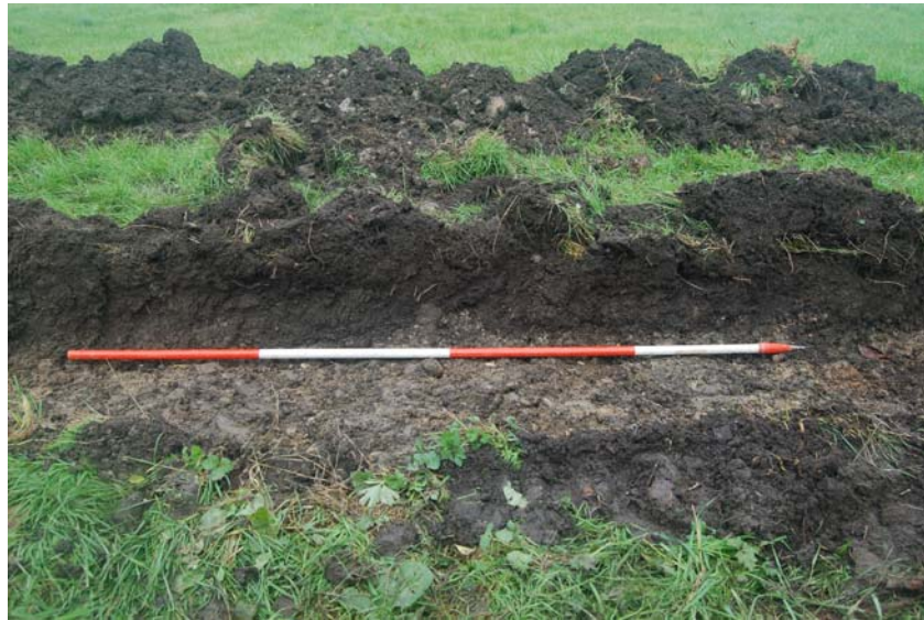
Plate 5: Degraded road surface, Trench 2 (facing north)
