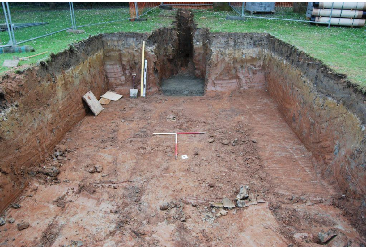
Plate 4 General view of Trench 3, looking south
