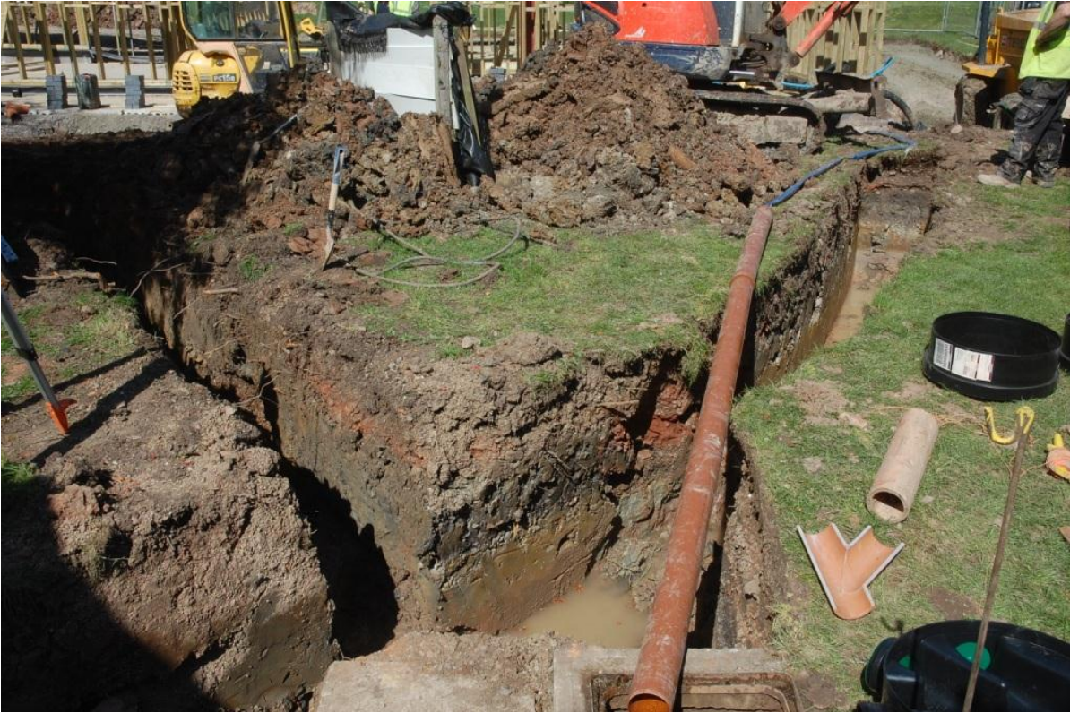
Plate 1 General view of Trenches 1 and 2, looking north
