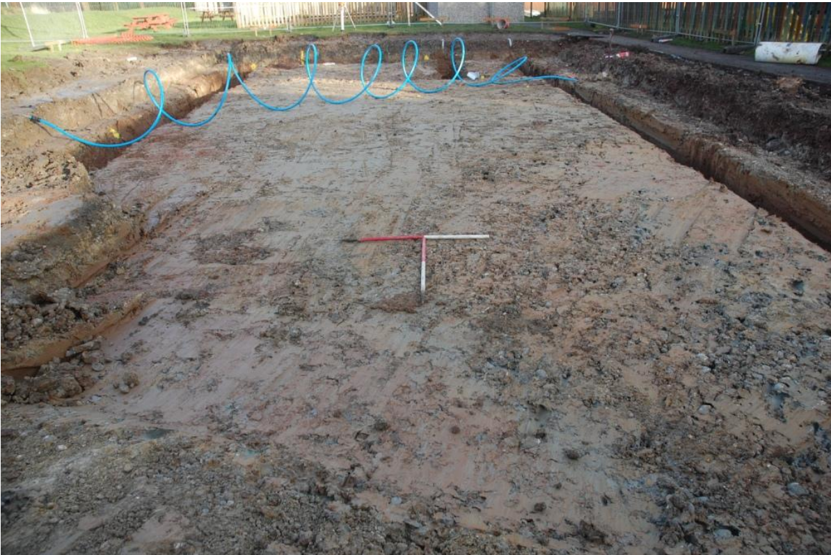
Plate 6 Trench 4 looking east
