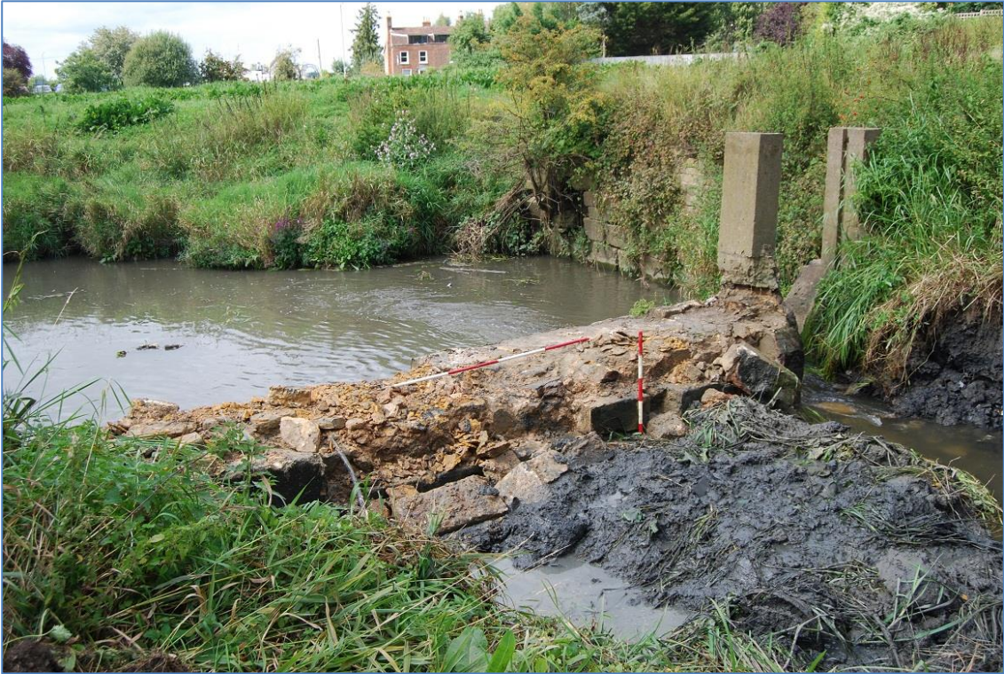
Plate 3: The weir [302] partially removed, looking northwest.
