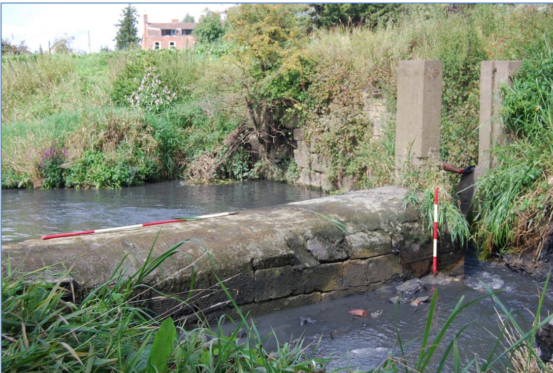
Plate 2: The weir [302] looking northwest.
