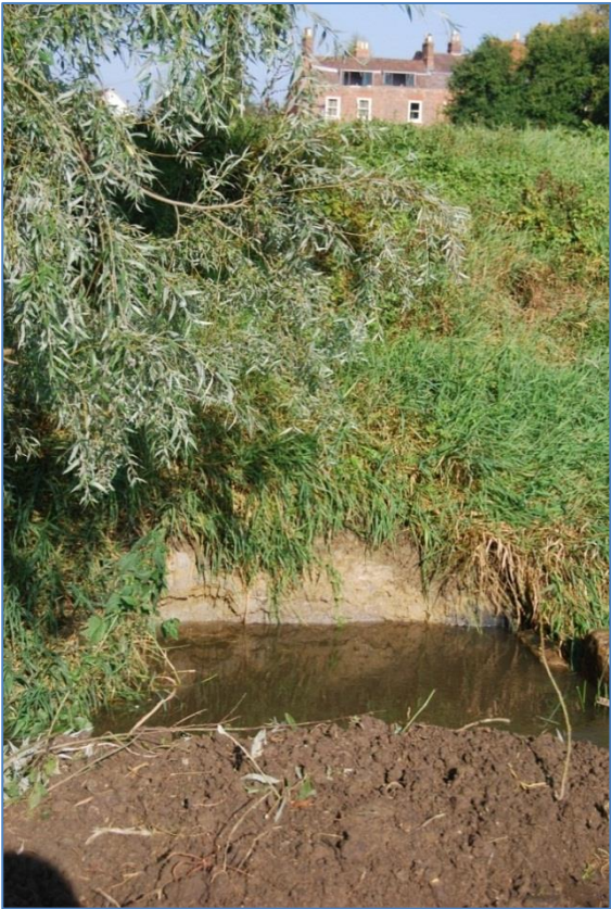
Plate 12: Slot 1 on completion of excavation, looking northwest.
