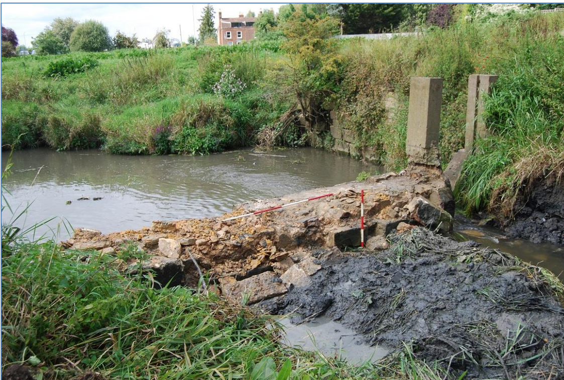
Plate 3: The weir [302] partially removed, looking northwest.
