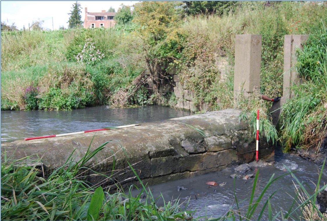
Plate 2: The weir [302] looking northwest.
