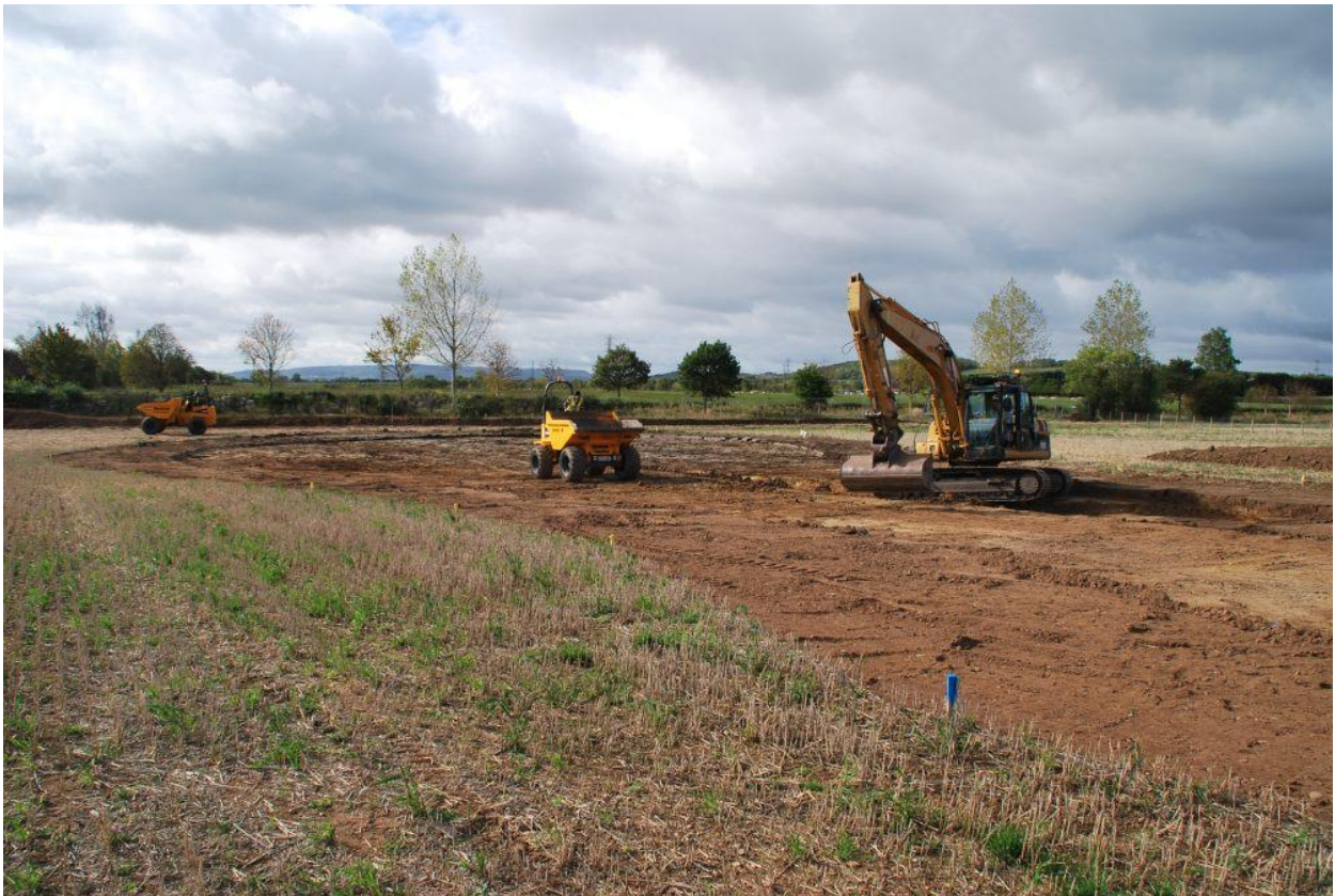
Plate 10 general view of Area 1 after soil stripping:
