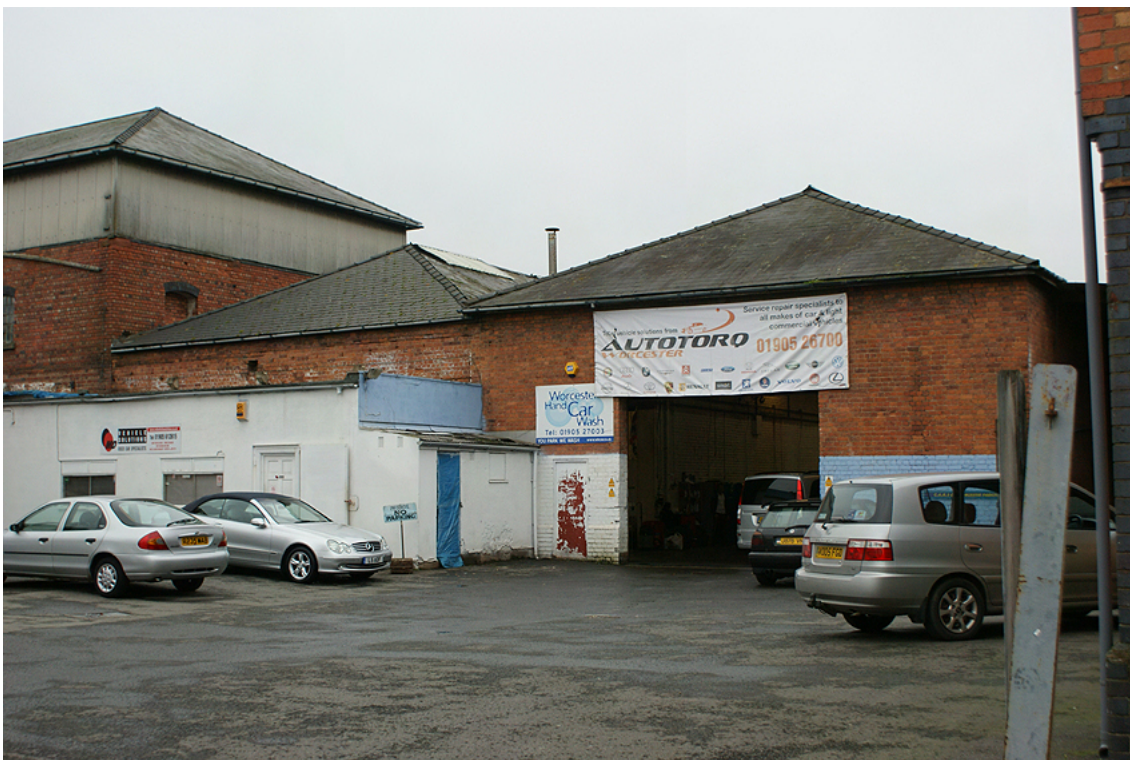
Plate 6: South Acidifying Shed from west
