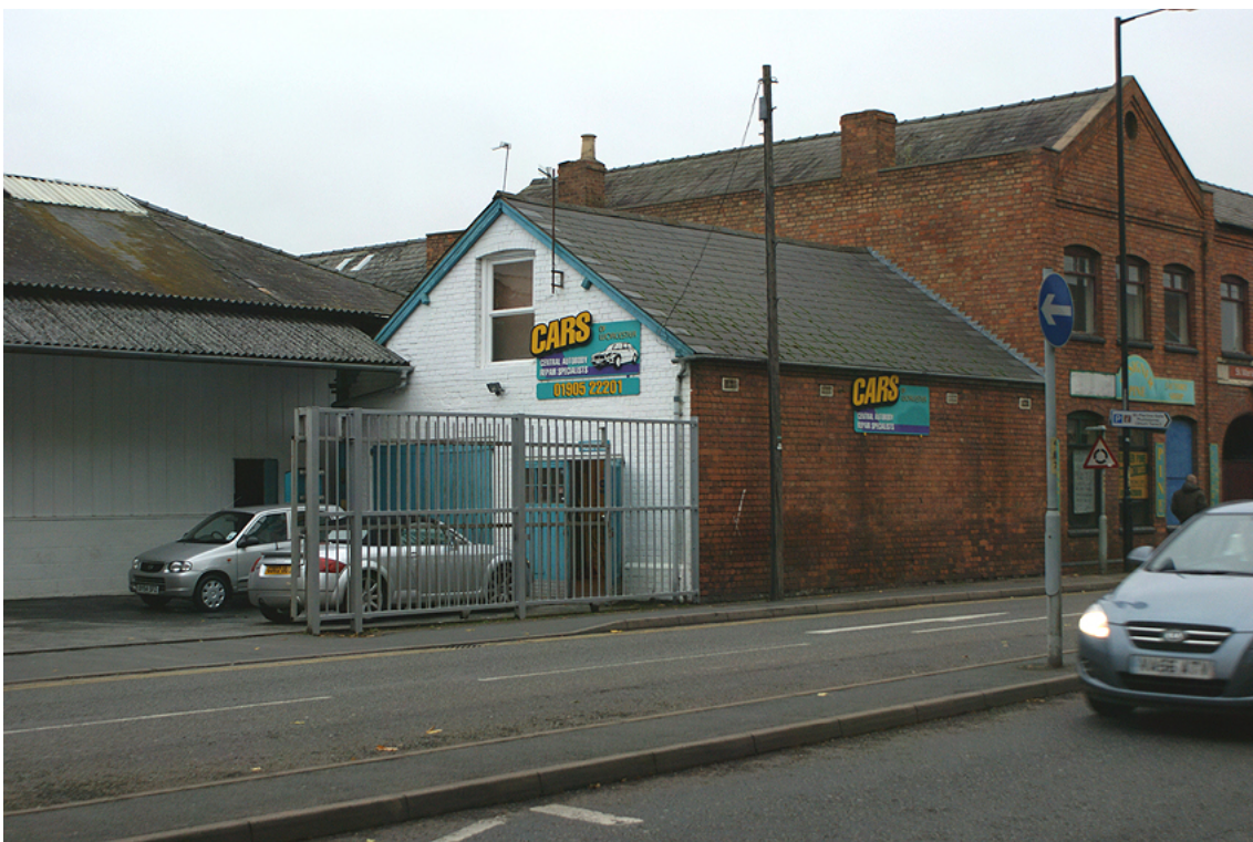
Plate 8: South east building on southern boundary
