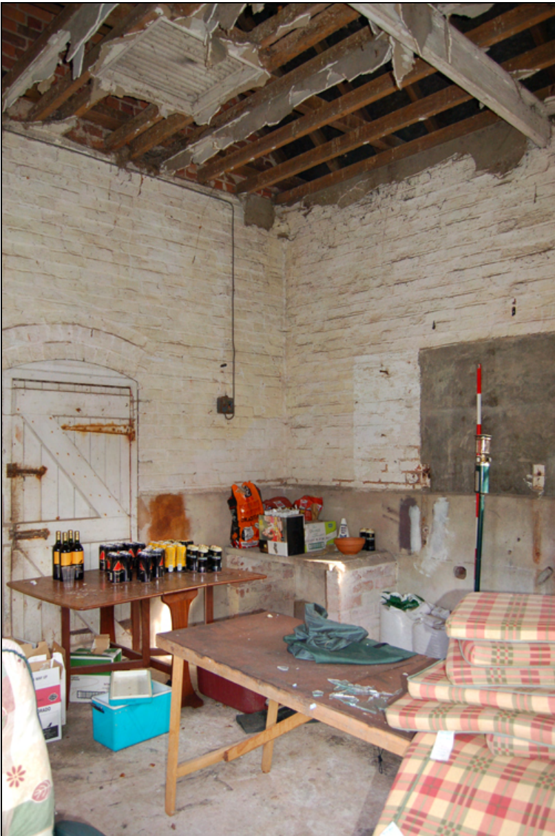
Figure 15: Work bench in north part of building
