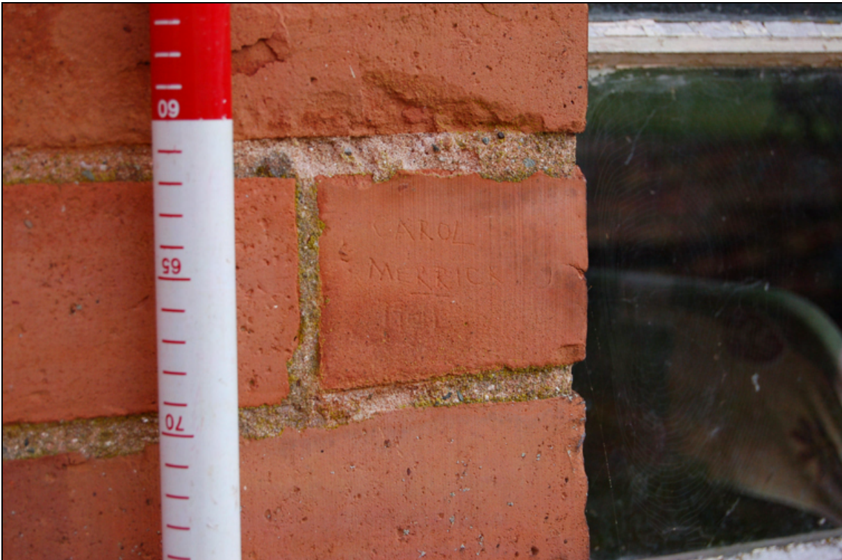
Figure 10: Graffito on the west elevation
