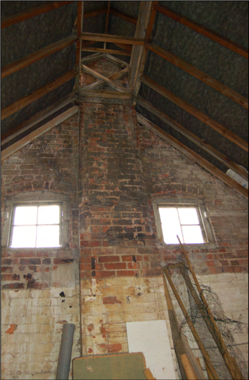
Figure 12: The chimney in the south part
