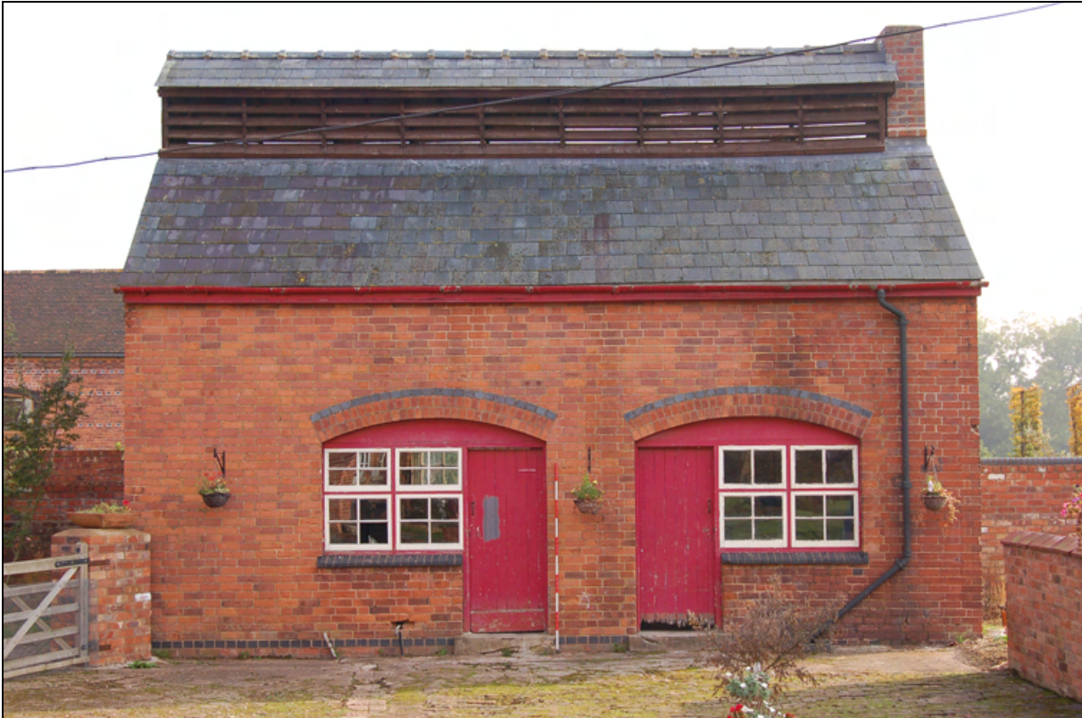
Figure 8: The west elevation
