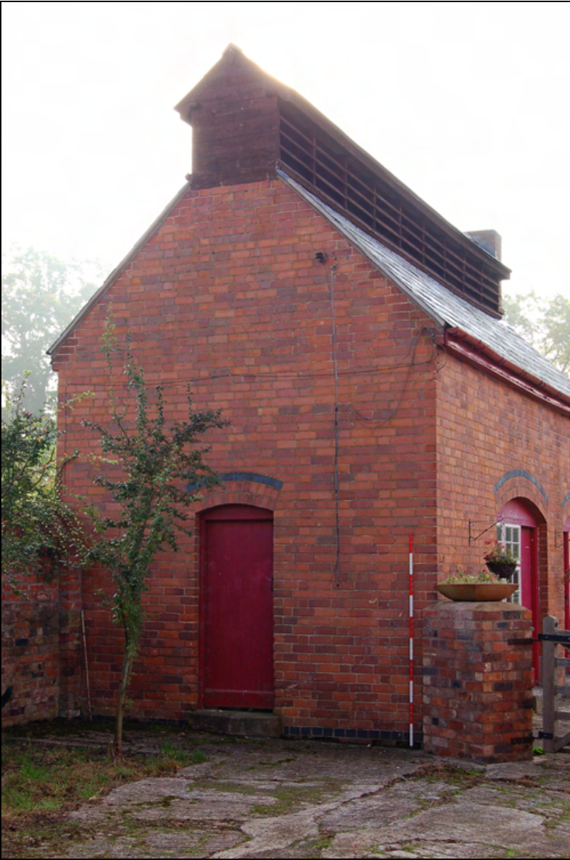
Figure 7: The north elevation
