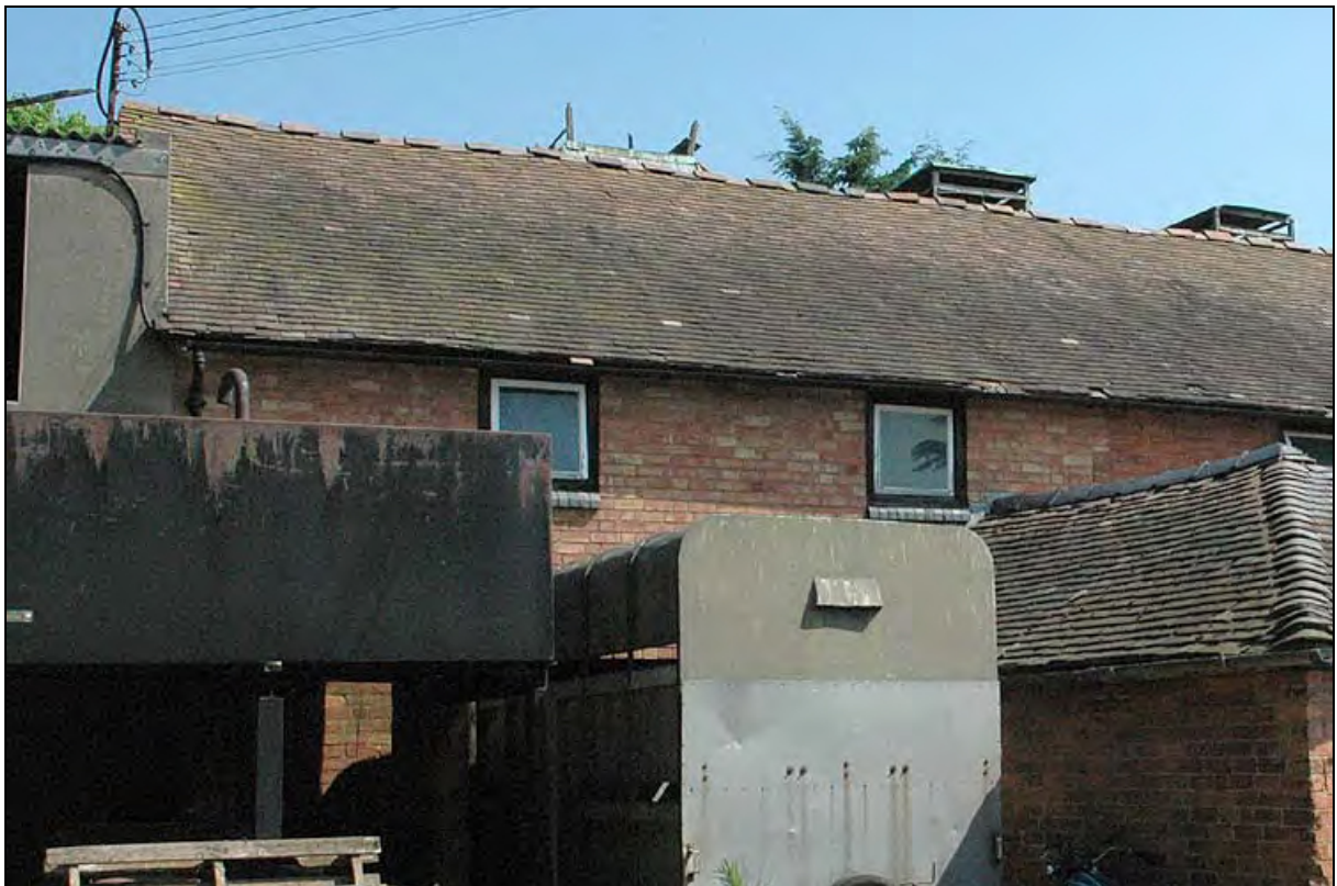
Plate 24: Mid 20 th century rebuilding of first floor of c1800 extension
