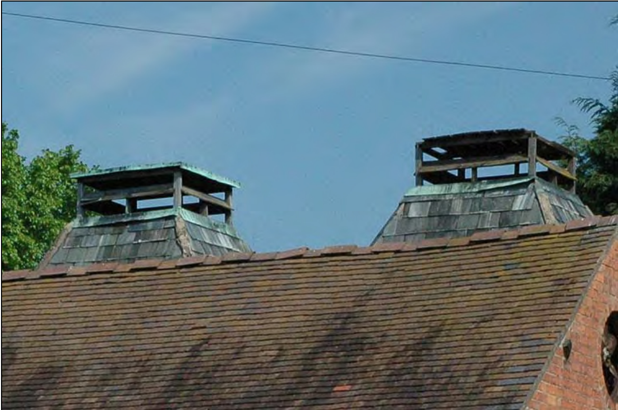
Plate 22: Louvre-vents on original kilns
