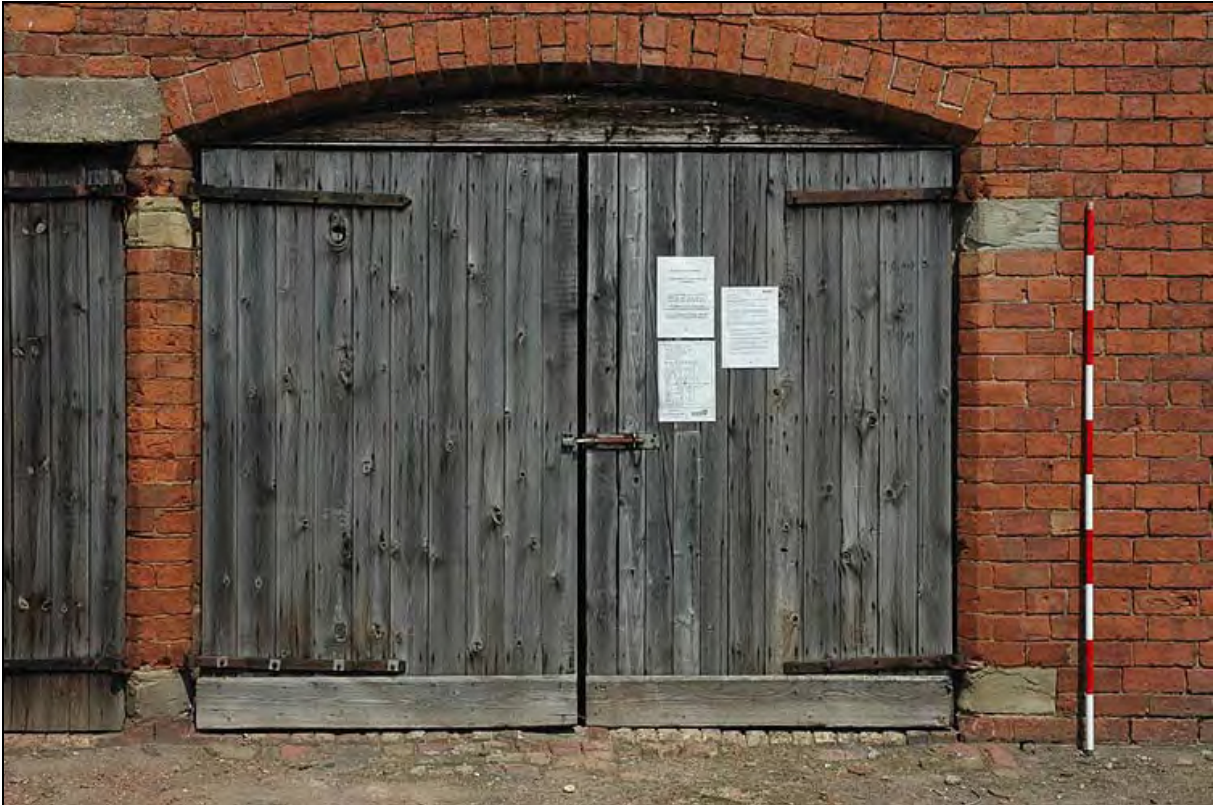
Plate 5: One of original late 18 th century segmental head openings
