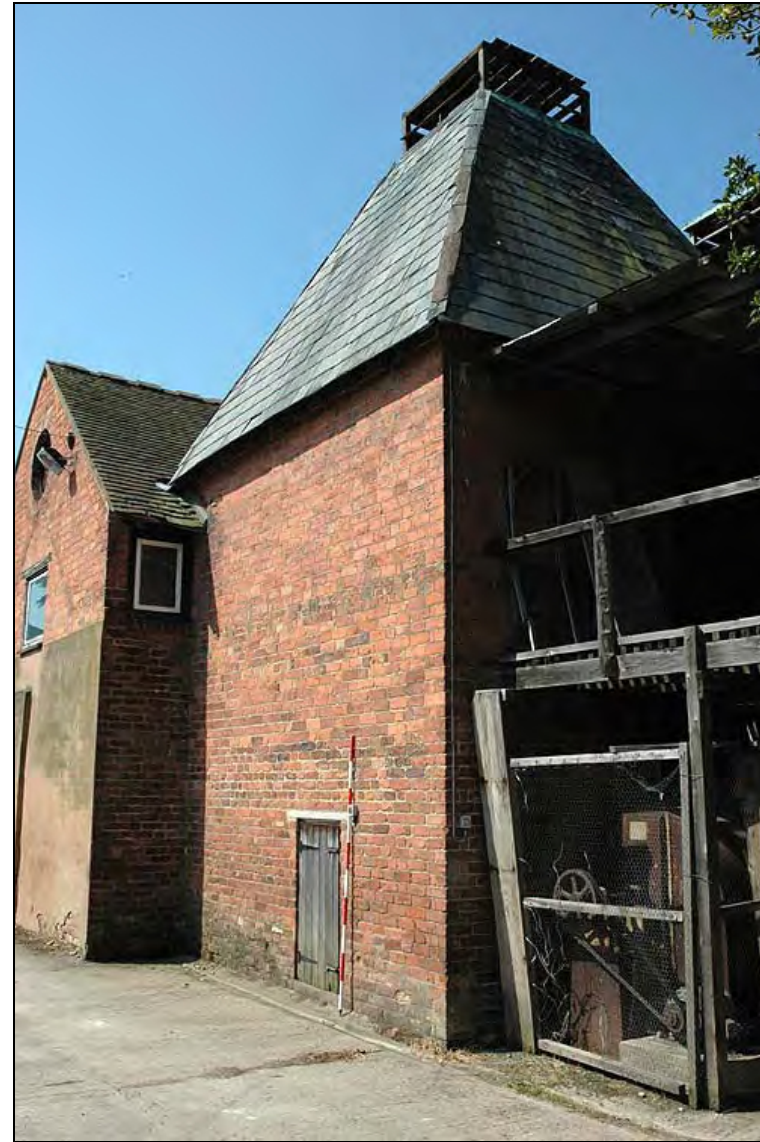
Plate 7: East elevation of late 18 th century kiln
