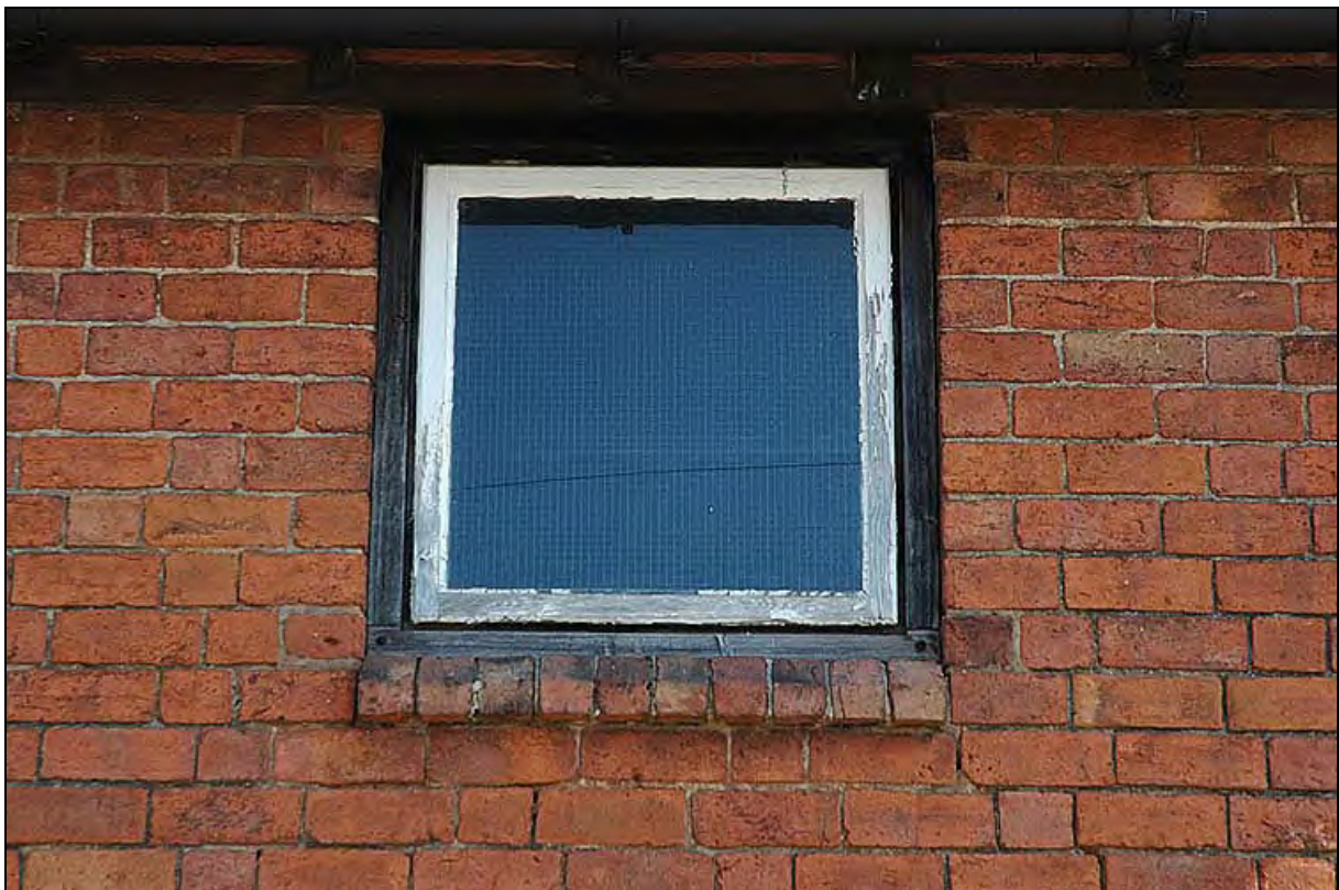
Plate 14: Segmental arch head window with chamfered brick cill
