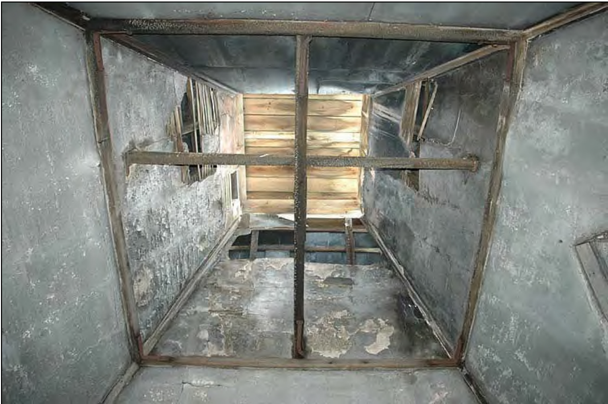
Plate 8: Internal space of the cone lined with plaster
