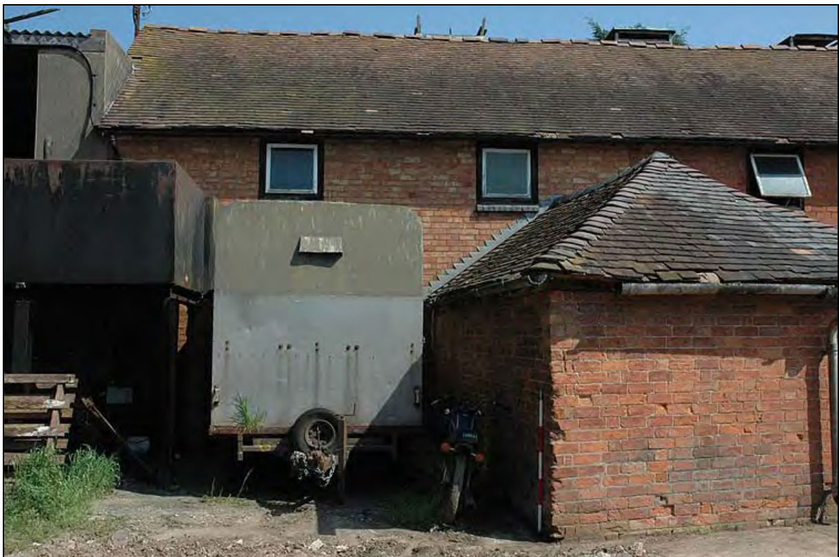
Plate 11: c1800 extension to west of the oast house (ground floor)
