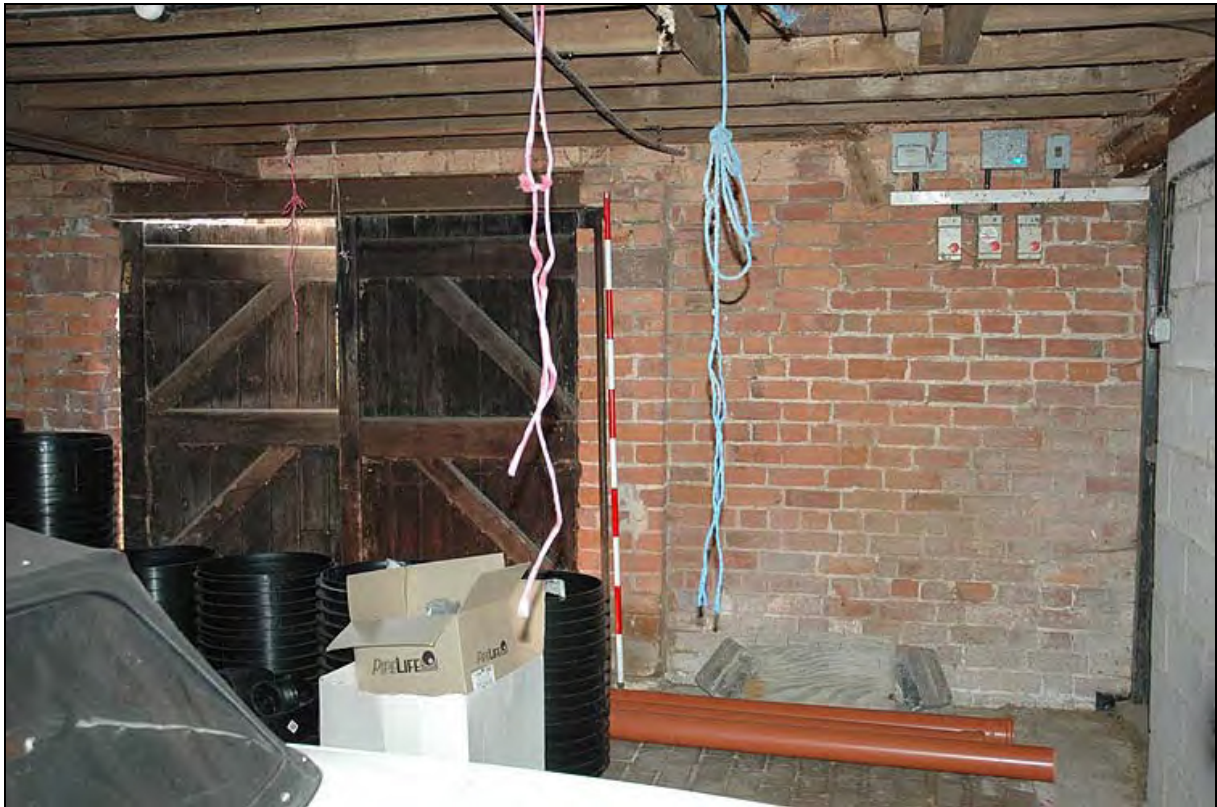
Plate 13: Large opening of c1800 with red sandstone hinge bases
