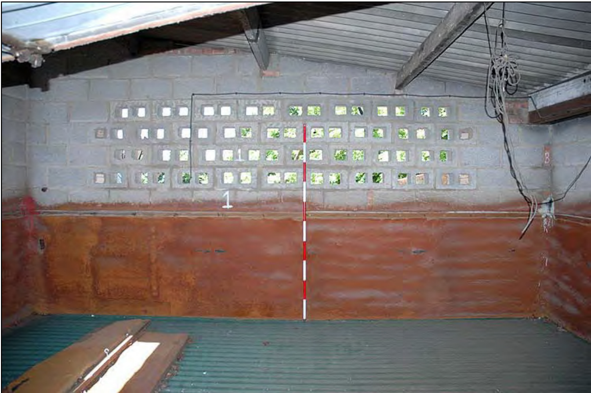
Plate 27: Honeycomb panel in modern breezeblock kiln
