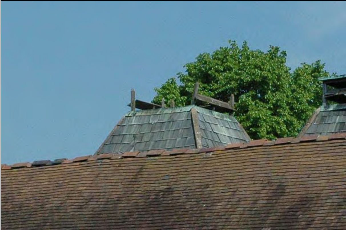
Plate 21: Louvre-vent on early 20 th century kiln
