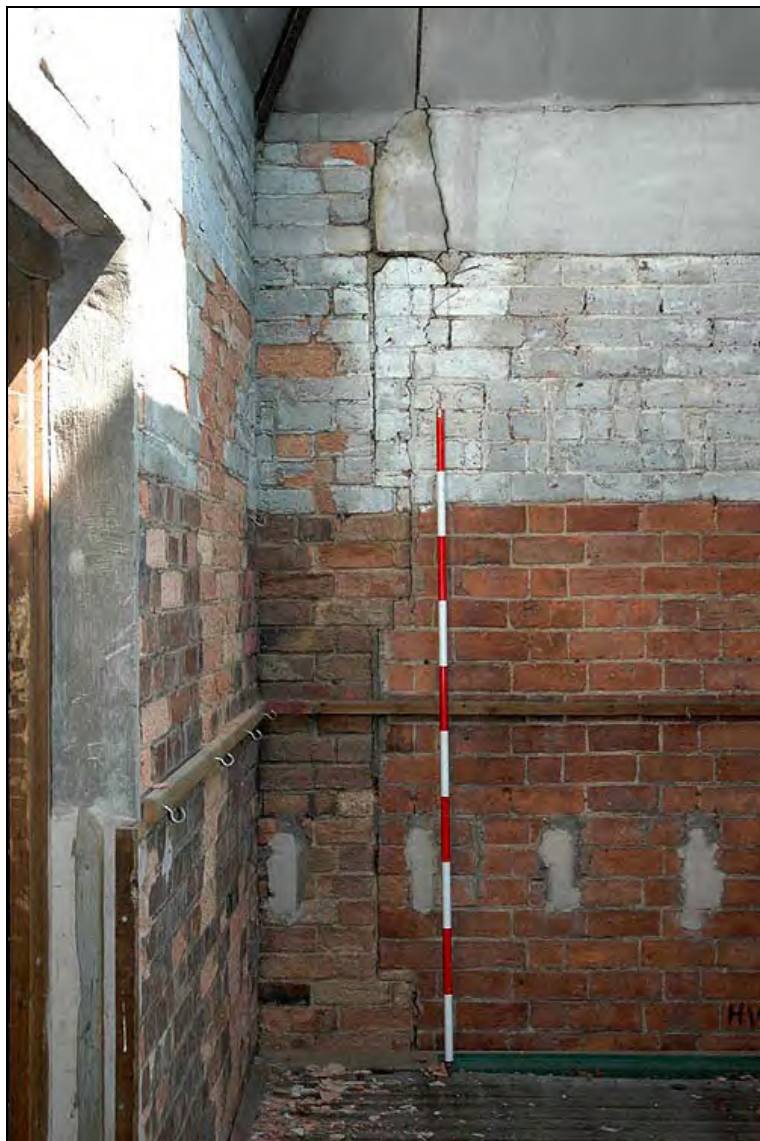
Plate 19: Joint between original kiln and early 20 th century kiln
