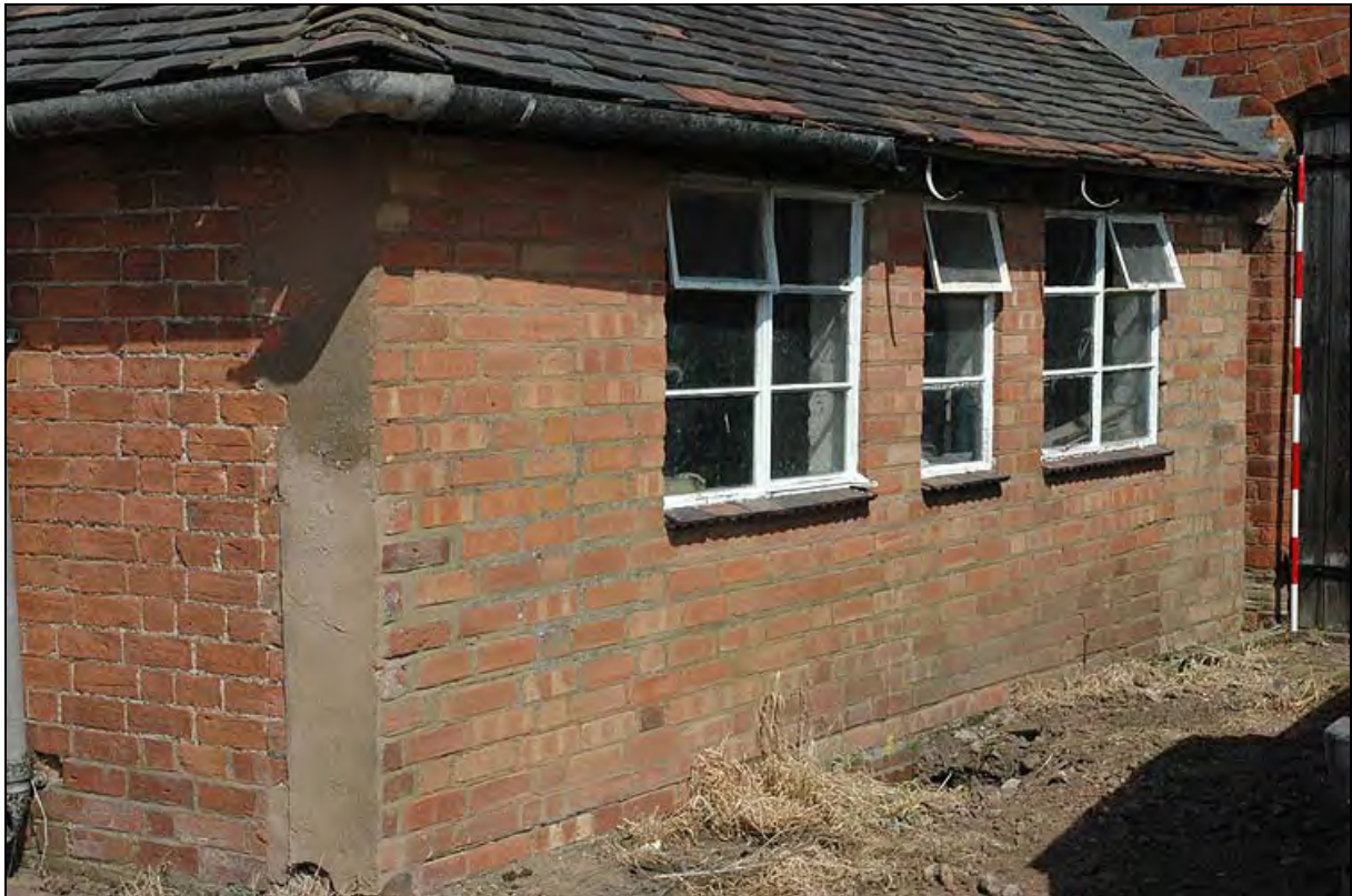
Plate 23: Mid 20 th century blocking of early 19 th century extension in London brick and iron-frame casements
