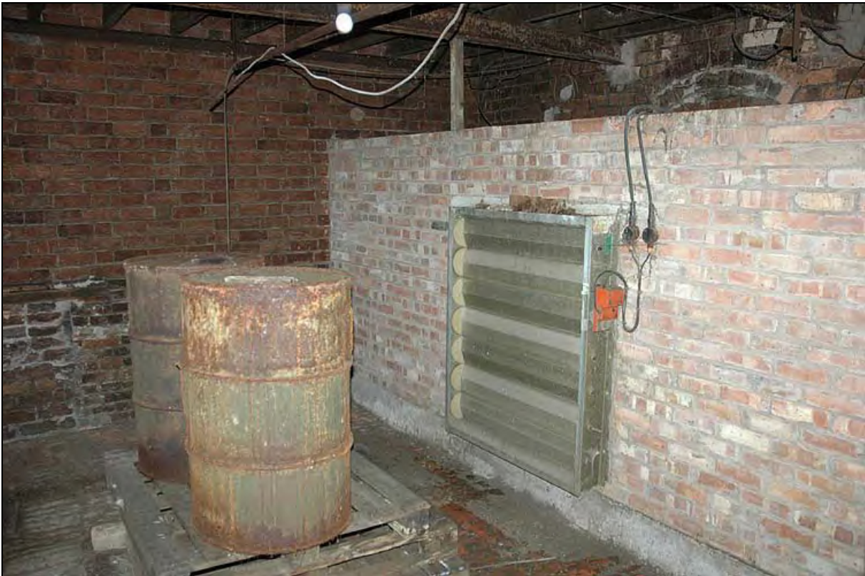
Plate 30: Vent and exterior of air tunnel inserted into the kiln
