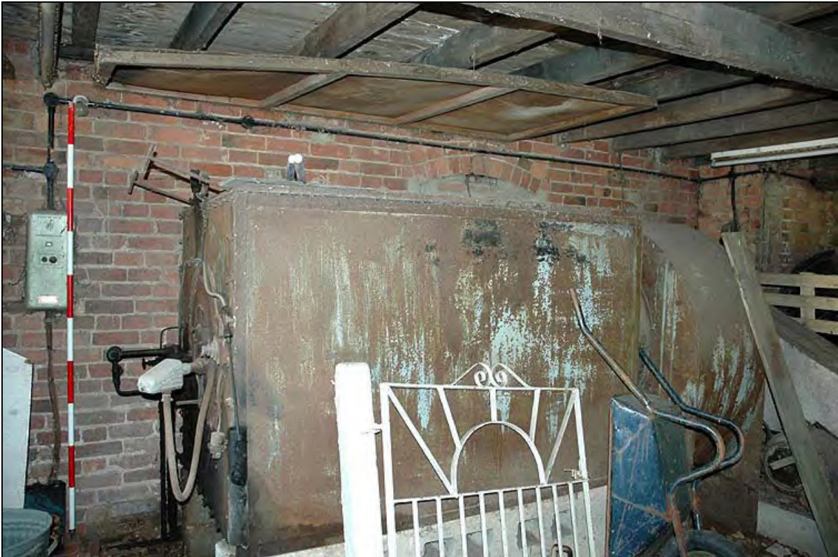
Plate 9: Segmental head doorway to plenum chamber hidden behind later oil-burning furnace
