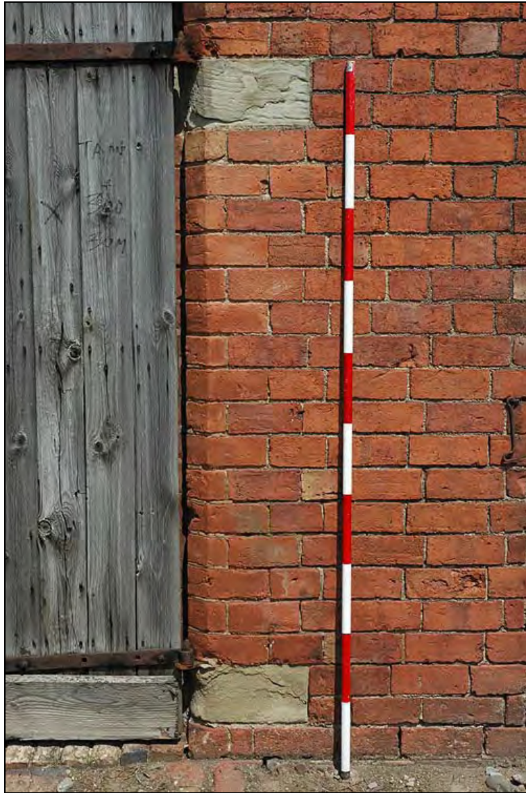
Plate 6: Moulded chamfered brick and decorative sandstone
