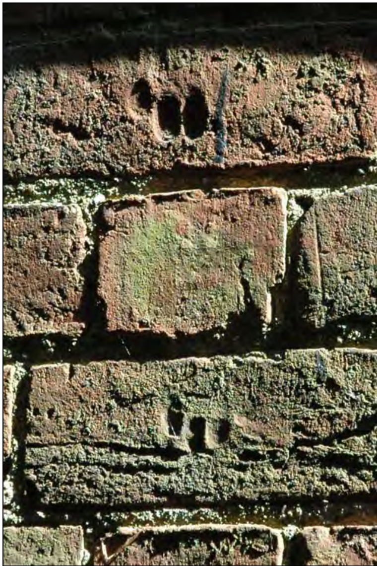
Plate 12: Example of finger marks on c1800 wall surface
