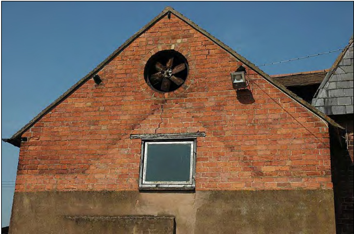
Plate 10: Building scar on east elevation of storage structure
