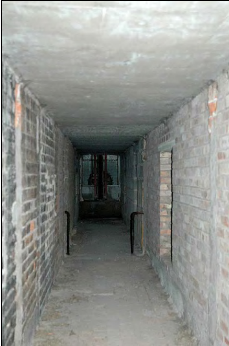
Plate 29: Air tunnel leading through the ground floor of the kilns
