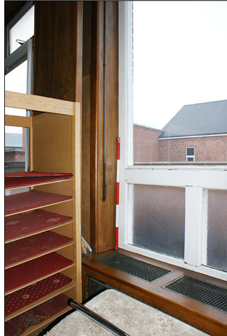
Plate 54: Window opening mechanism in 1950s showroom
