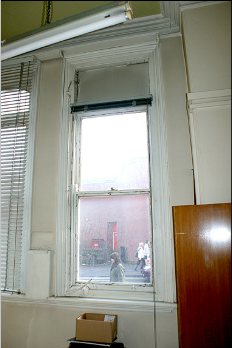
Plate 27: Tall ground floor window with bar and catch opening system
