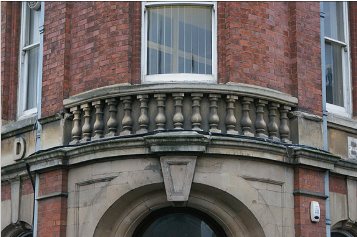
Plate 14: Balustrade above main entrance
