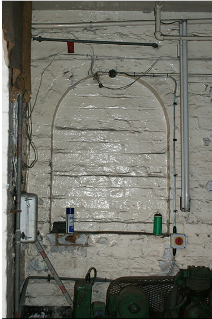
Plate 3: One of the blocked windows in the early 19 th century building
