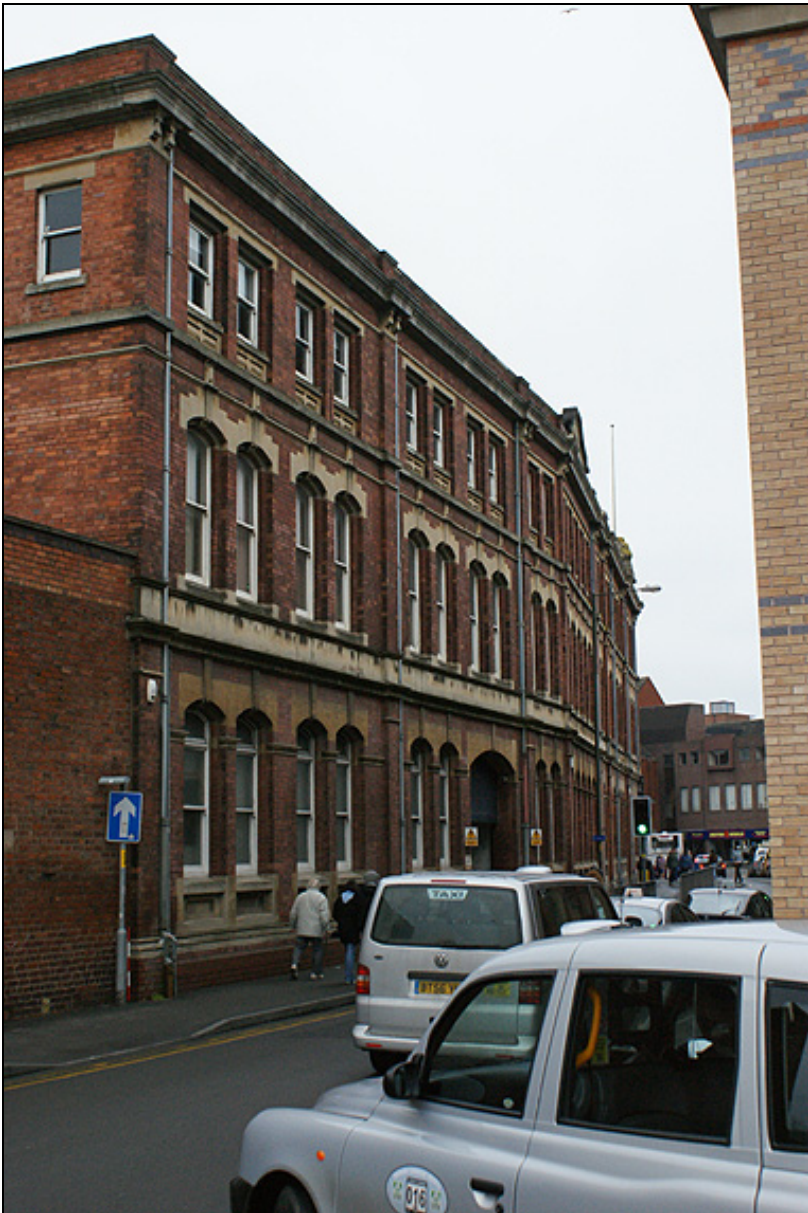
Plate 1: The building from the south west
