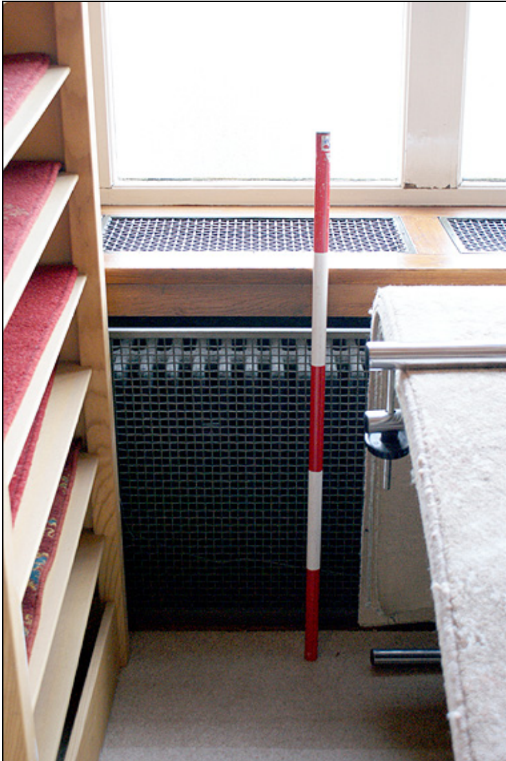
Plate 53: Built in radiator and grill in 1950s showroom
