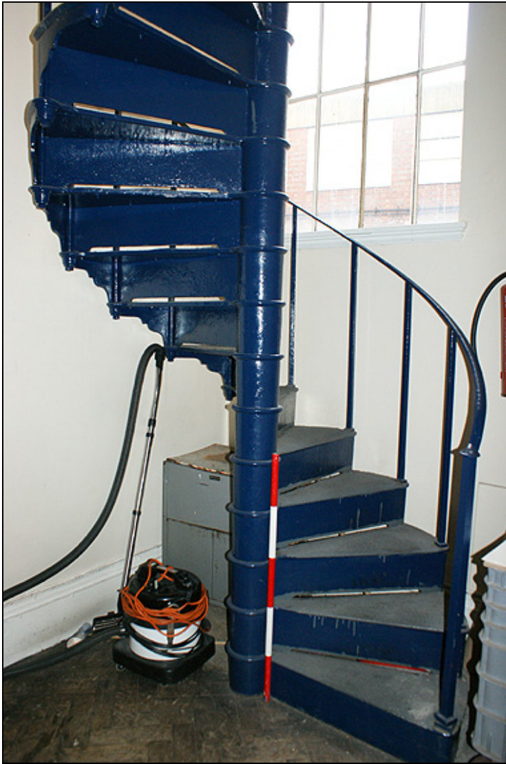
Plate 44: Steel spiral staircase
