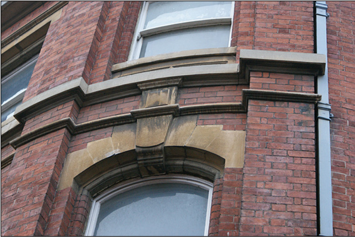
Plate 18: Stringcourse between the first and second floors
