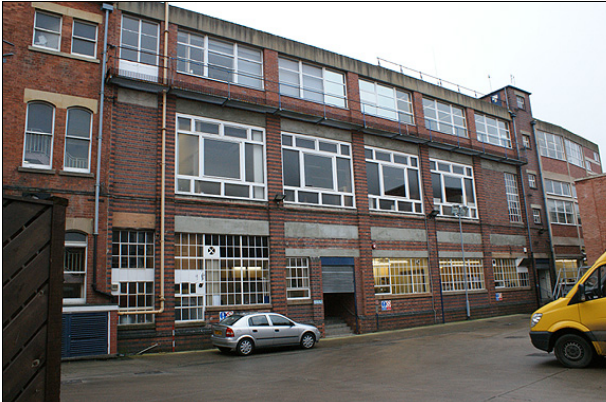
Plate 10: Mid 19 th century building from the north east, note the polychrome brickwork
