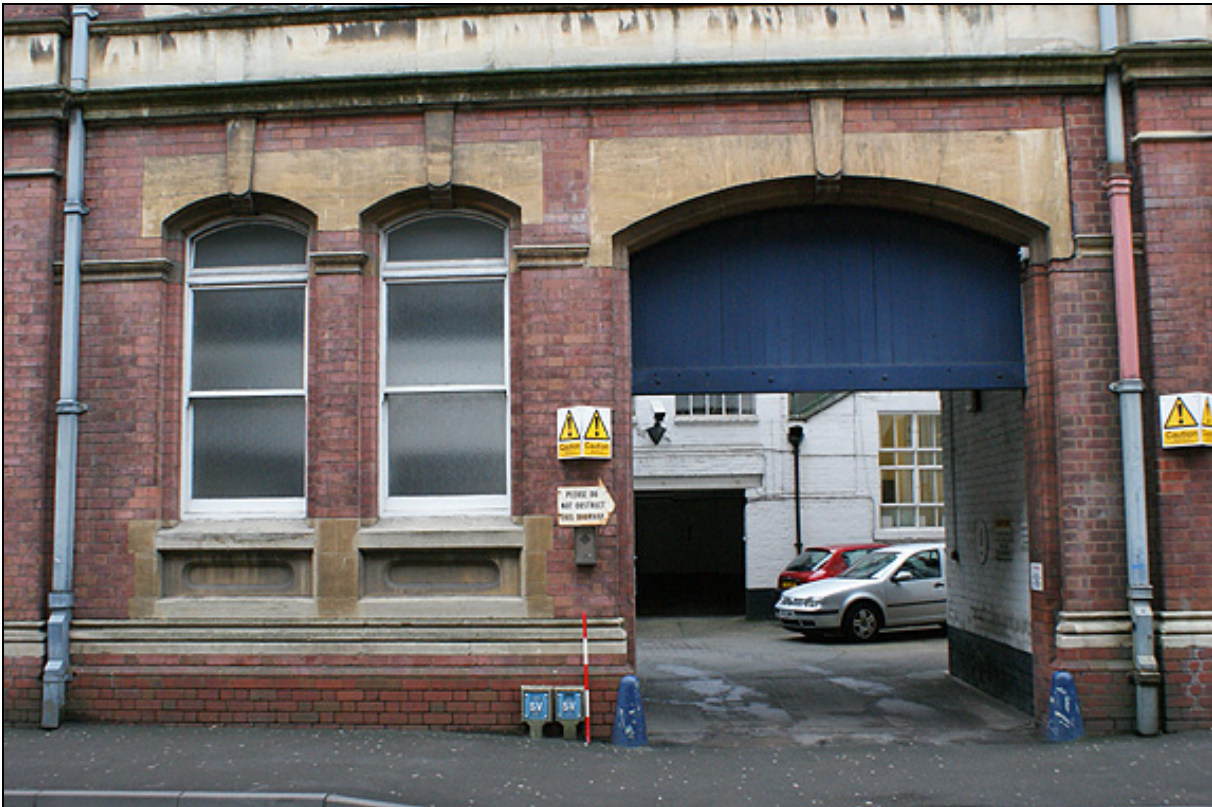
Plate 39: Large opening on Exchange Street, part of 1926 structure
