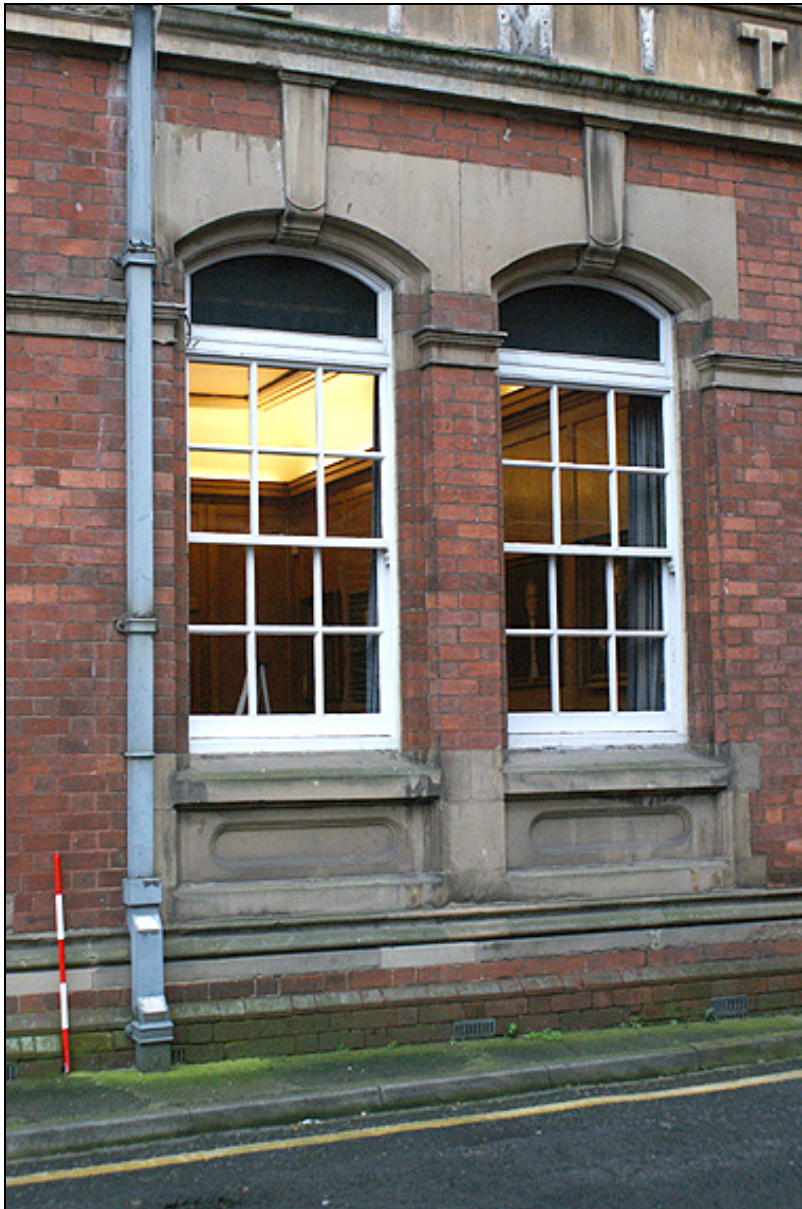
Plate 19: Ground floor windows and aprons of 1876 building
