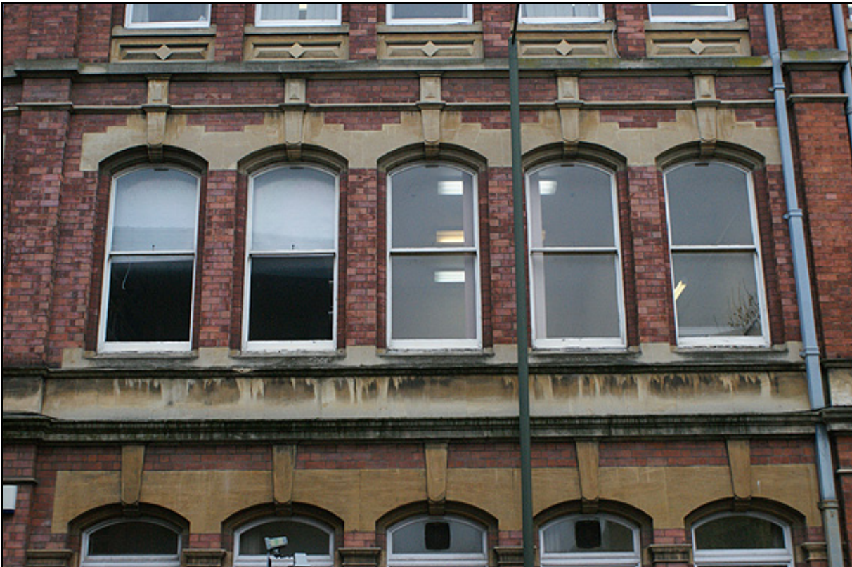
Plate 37: Arches over windows on 1926 building, different to 1896 building
