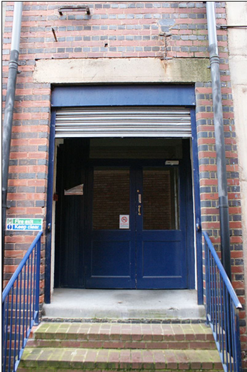
Plate 46: Large opening in remodelled mid 19 th century building
