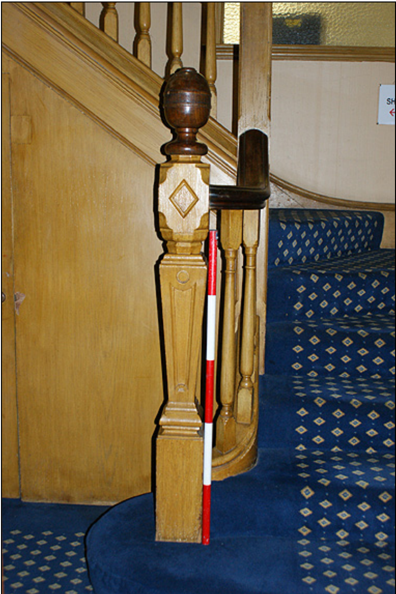
Plate31: 1876 mahogany staircase with tapered balusters and chunky newel post
