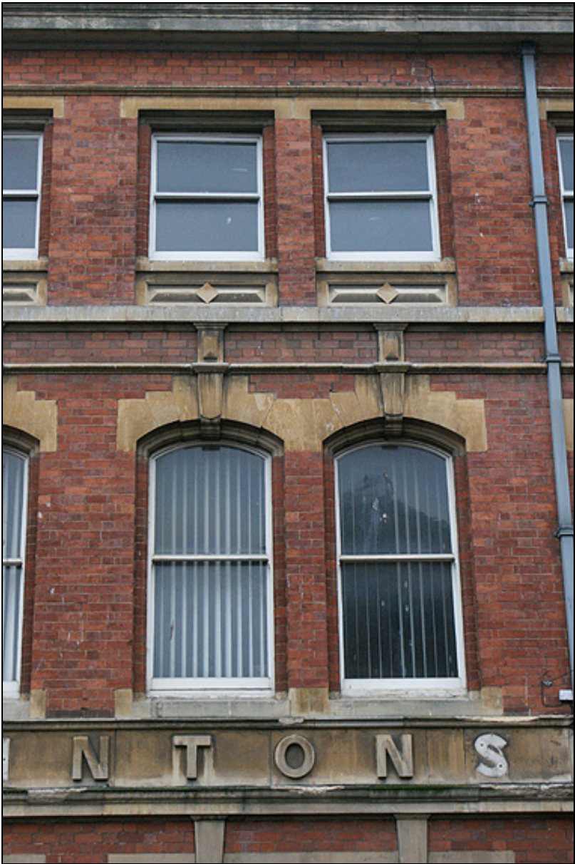
Plate 13: Cambered stone arches on 1876 building
