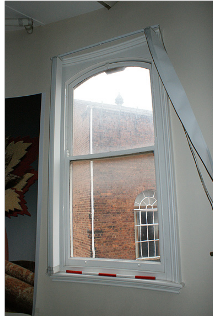
Plate 25: Segmental arched glass and moulded architrave and cill
