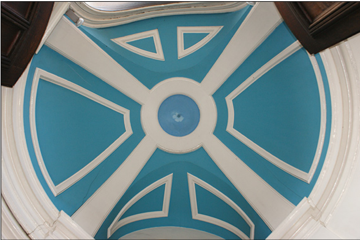
Plate 21: Entrance way domed ceiling with moulded plasterwork
