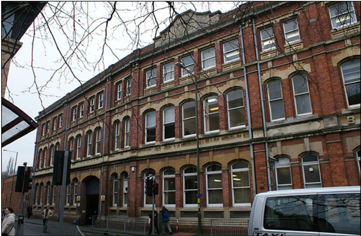
Plate 34: 1876 style matched in the 1926 structure (left of the double drainpipes is 1926, to the right is 1876).
