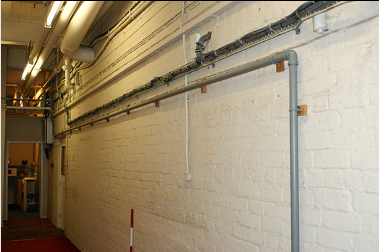
Plate 8: Rear wall of mid 19 th century building with blocked openings
