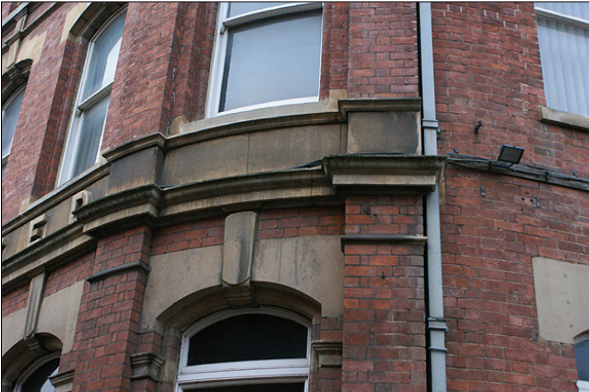
Plate 17: Stringcourse between the ground and first floors
