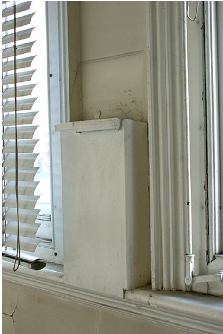
Plate 29: Surviving 1876 air vent
