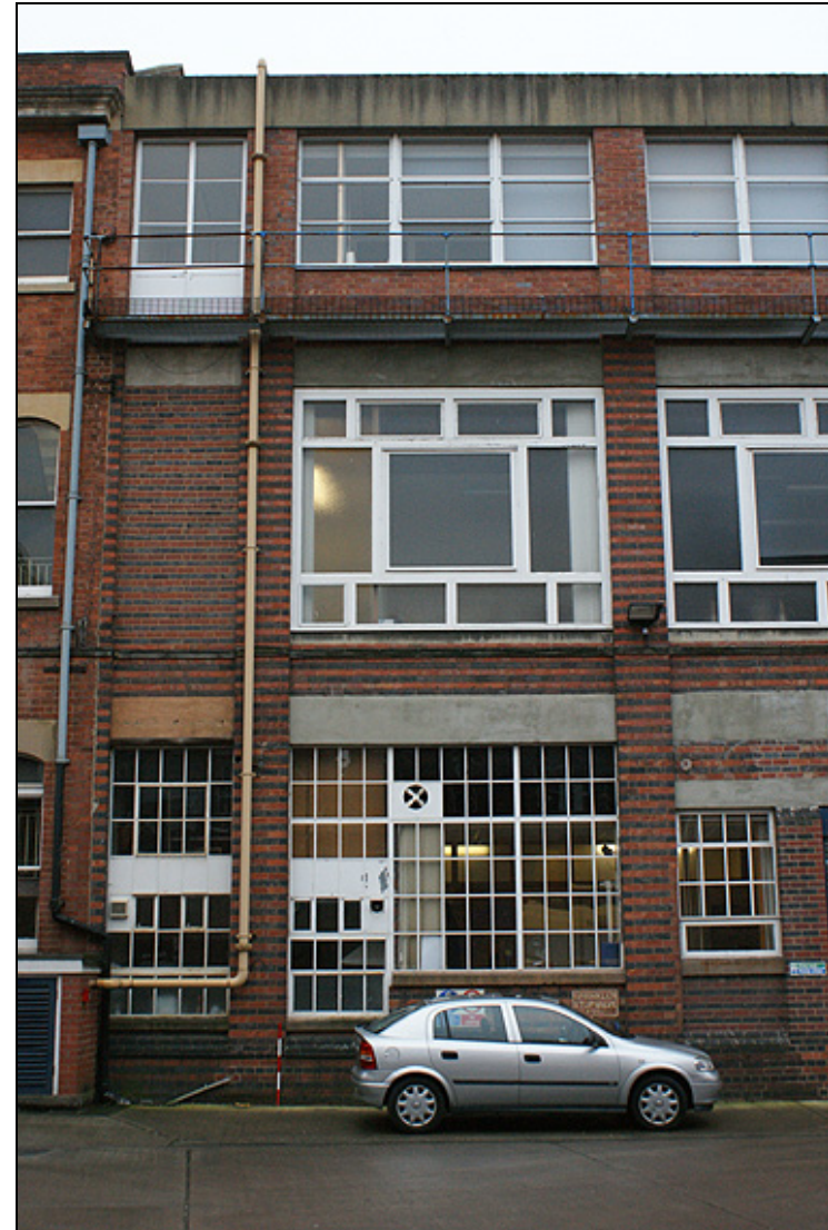
Plate 45: Top floor added to mid 19 th century building, notice different bricks
