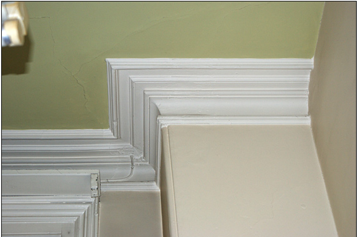
Plate 26: Heavily moulded cornice
