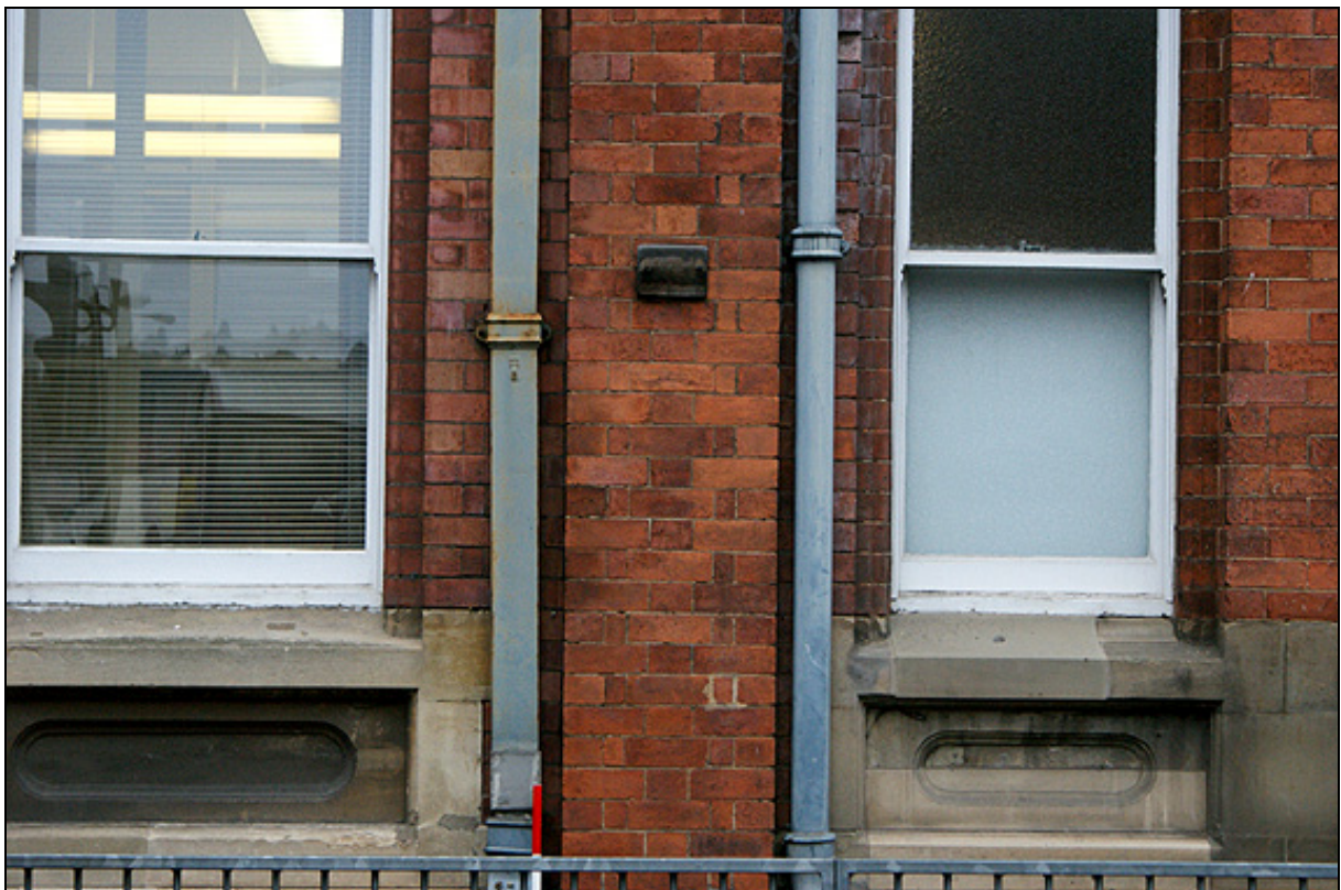
Plate 35: Different brick colours (left of the drainpipes is 1926, to the right is 1876).
