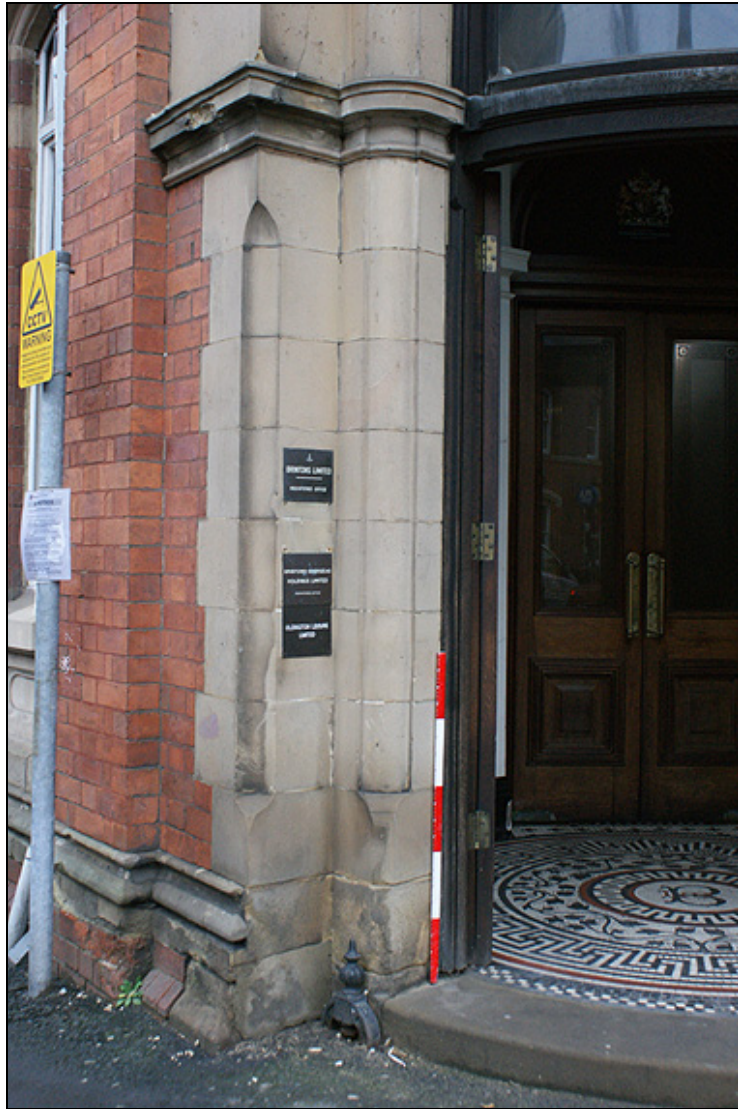
Plate 15: Recessed pilasters at entrance
