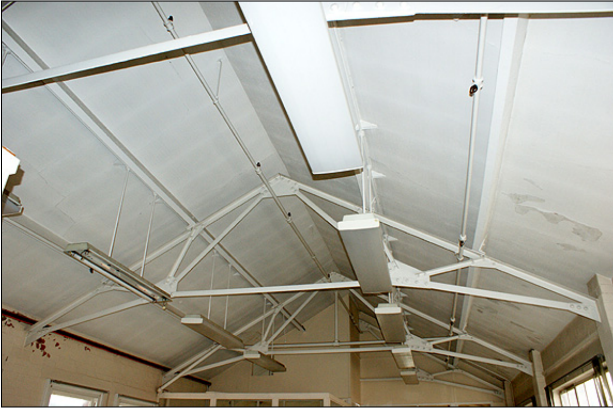
Plate 40: Steel trusses in 1926 structure
