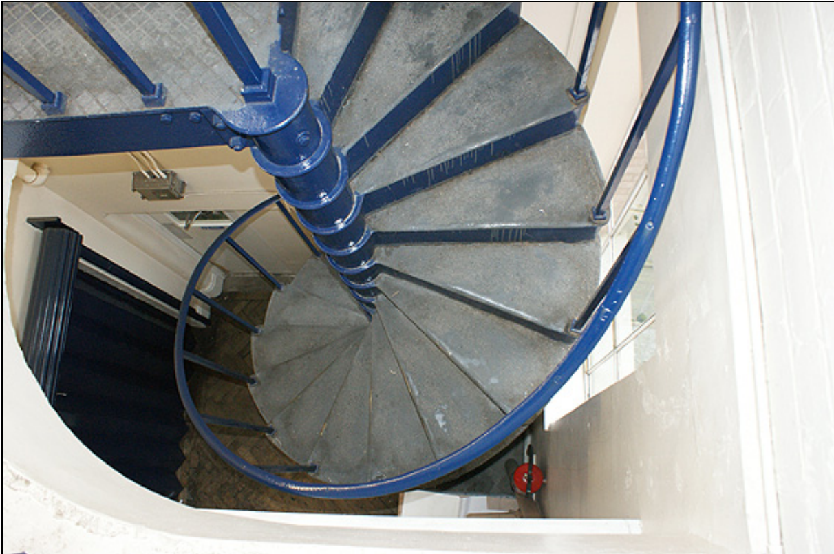
Plate 43: Steel spiral staircase
