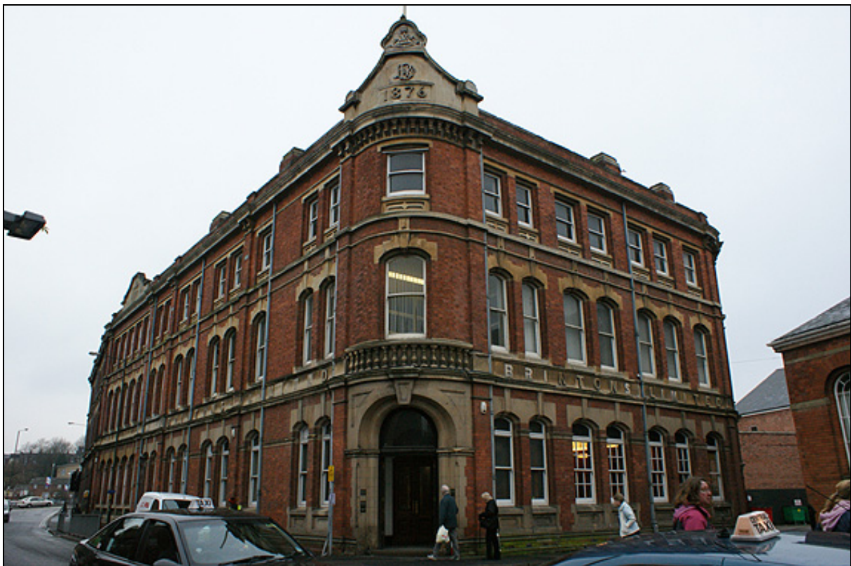
Plate 11: 1876 Brinton's Offices building
