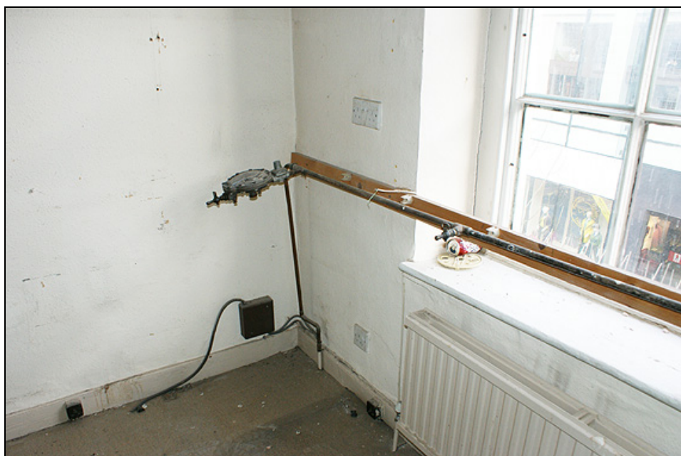
Plate 28: Industrial gas fittings, 84 High Street
