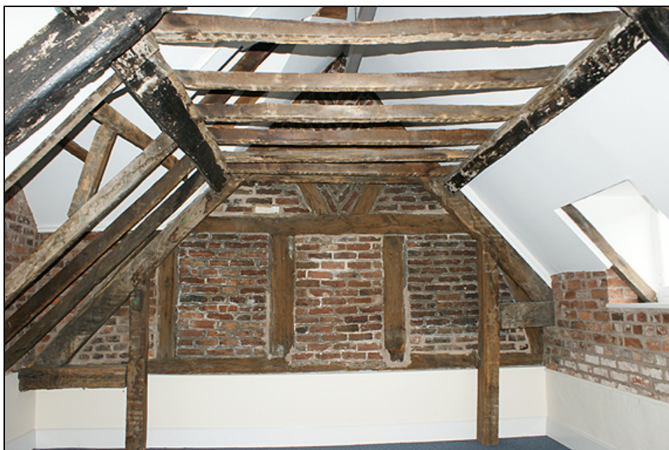
Plate 34: 17 th century timber framing of 84 High Street, visible from 85 High Street
