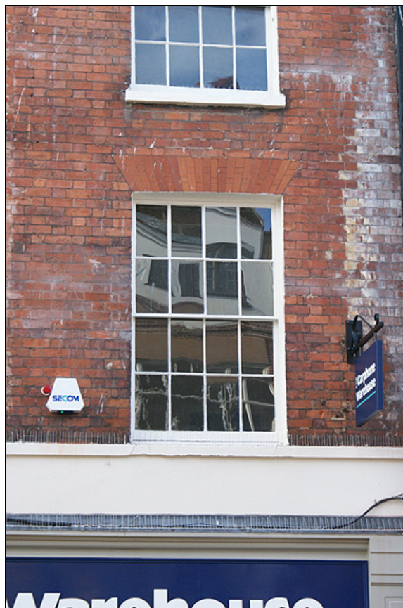
Plate 11: Original 8/8 sash window
