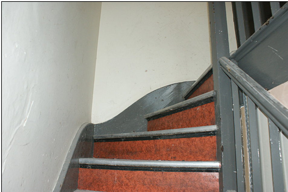
Plate 24: 19 th century staircase skirting board, 84 High Street
