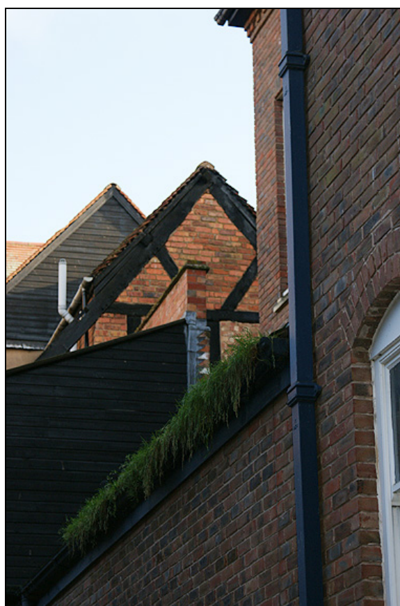
Plate 32: 17 th century timber framing, 84 High Street
