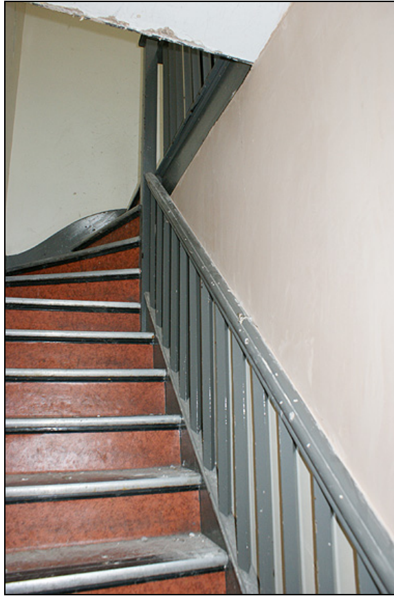
Plate 23: 19 th century first to second floor staircase, 84 High Street, with stick balusters
