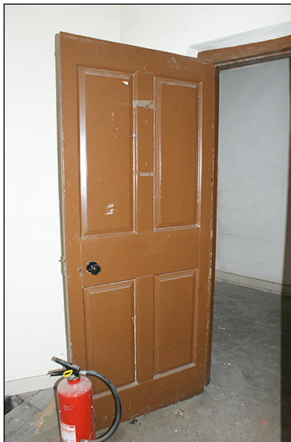
Plate 26: 19 th century panelled door with Bakelite handle, 84 High Street
