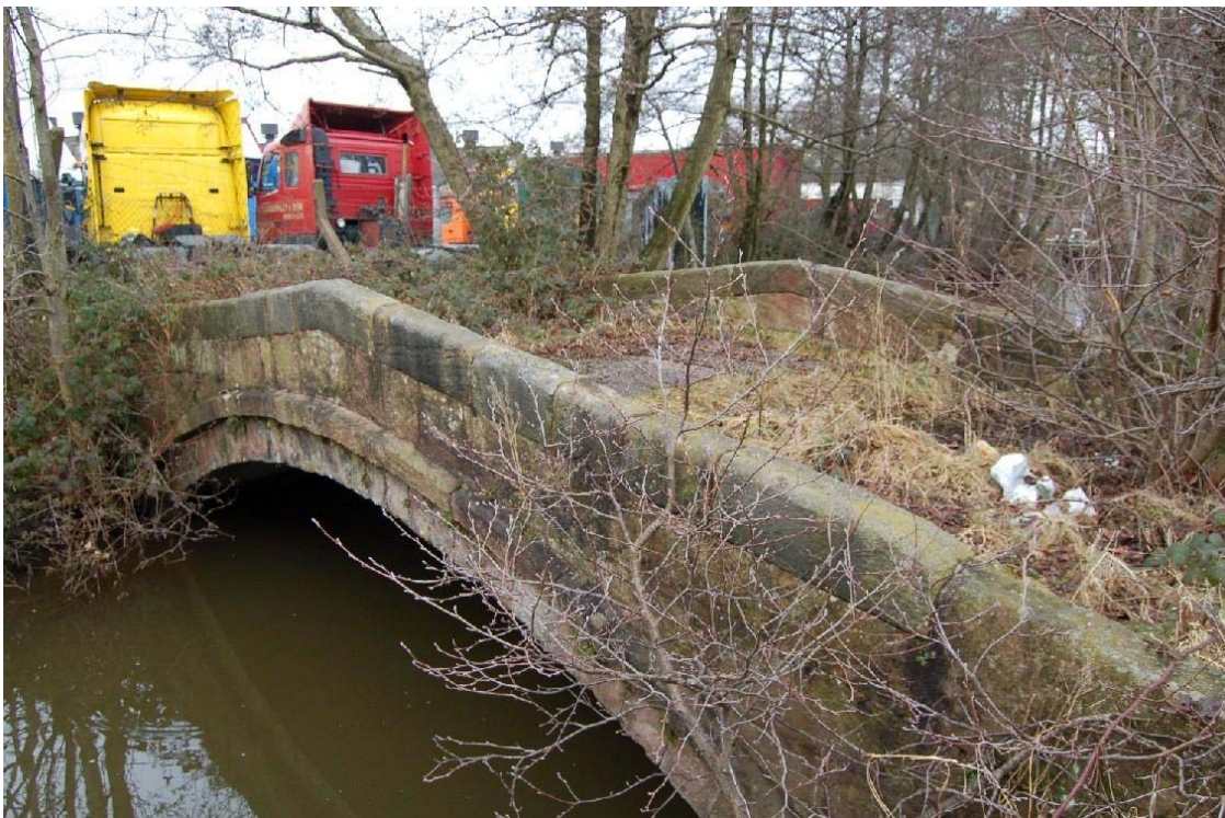
Plate 6, the River Churnet stone footbridge, facing west
