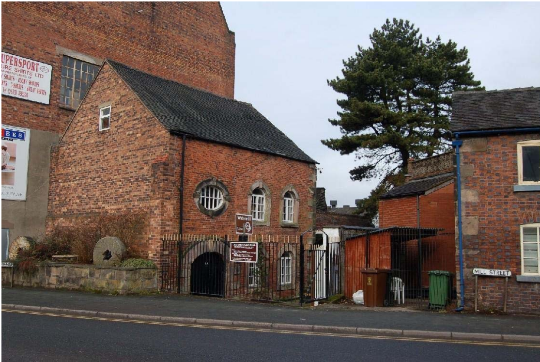
Plate 3, Brindley Corn Mill, from Mill Street, looking northwest
