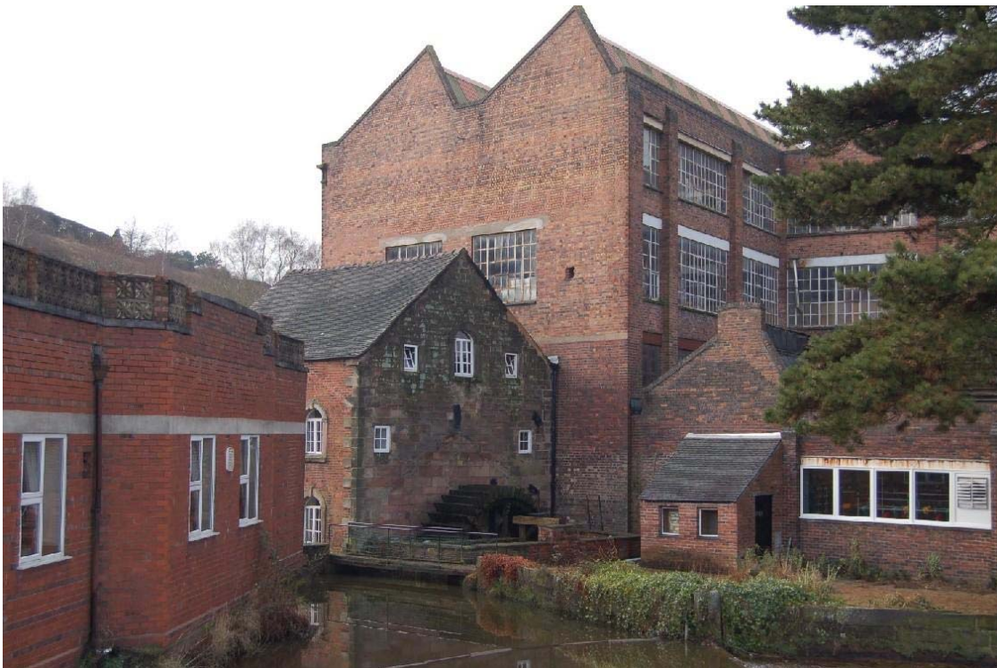
Plate 4, Brindley Corn Mill, from Abbey Green Road site entrance, looking southwest
