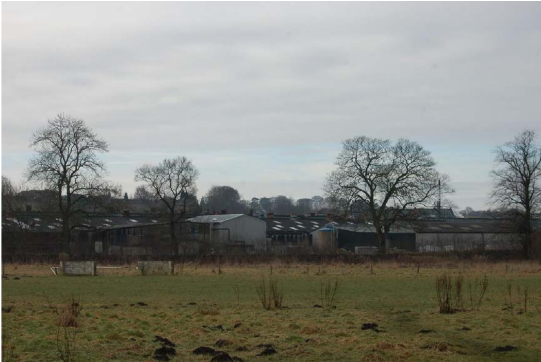
Plate 1, the site from Broad's Bridge, facing south
