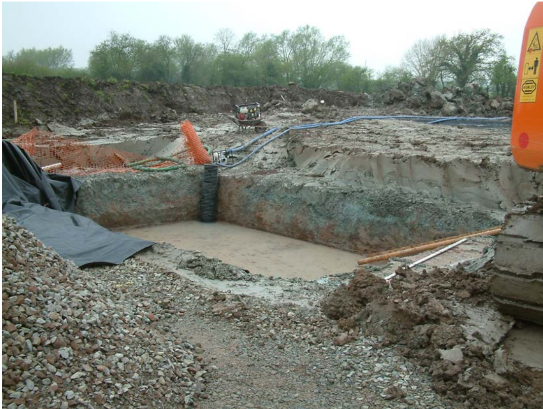
Plate 3: Machined excavation for settling tank, facing southwest
