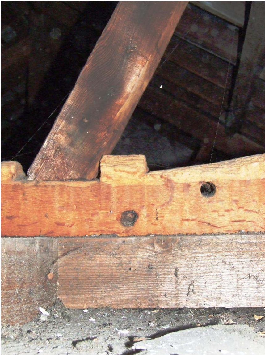
20. Detail of reuse of earlier roof beams
