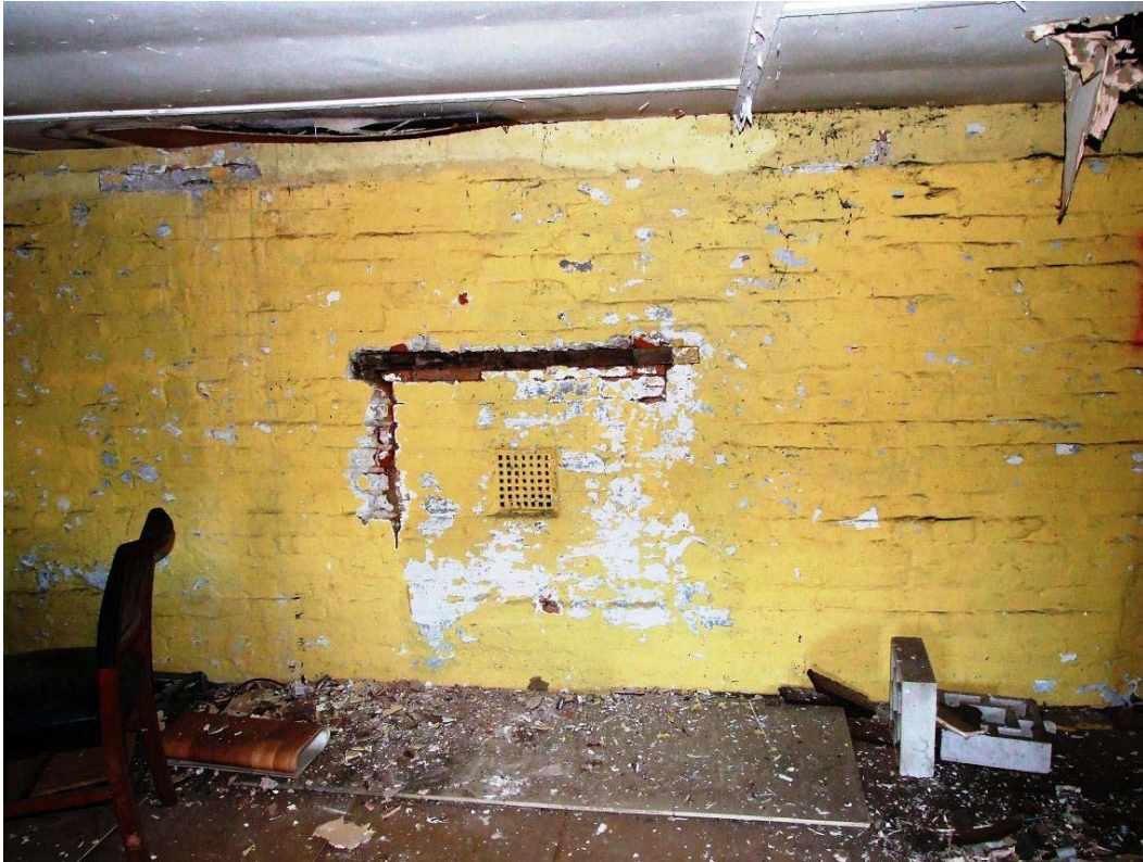
18. View of blocked 1 st floor windows in W. Elevation
