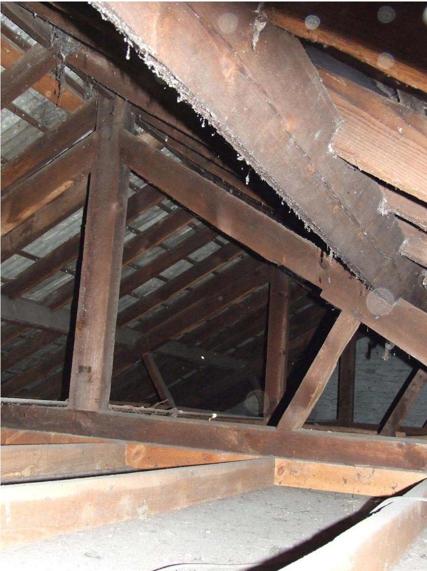
19. Detail of later roof truss assembly
