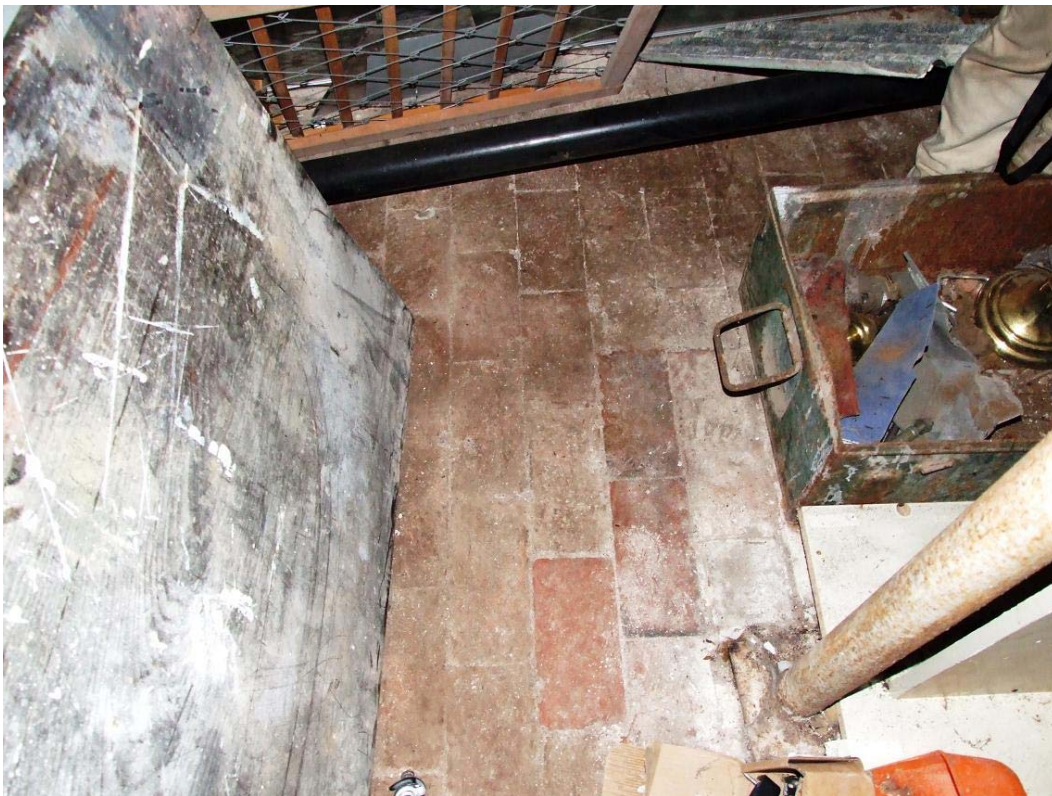
16. Basement, brick pavements and quarry-tiled floor
