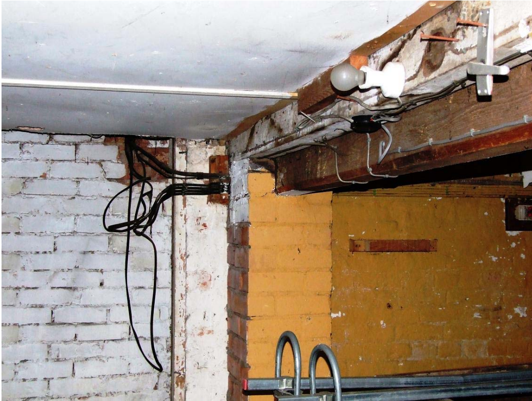
15. Basement, kiln party wall, later strengthening and blocking of access ways
