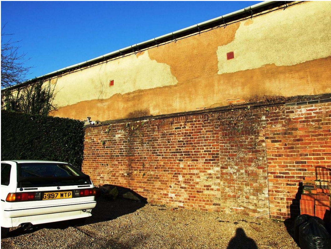
4. Detail of W. Elevation including blocked doorway in garden wall
