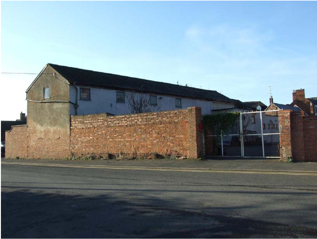
1. General view of S. Gable and E. Elevation
