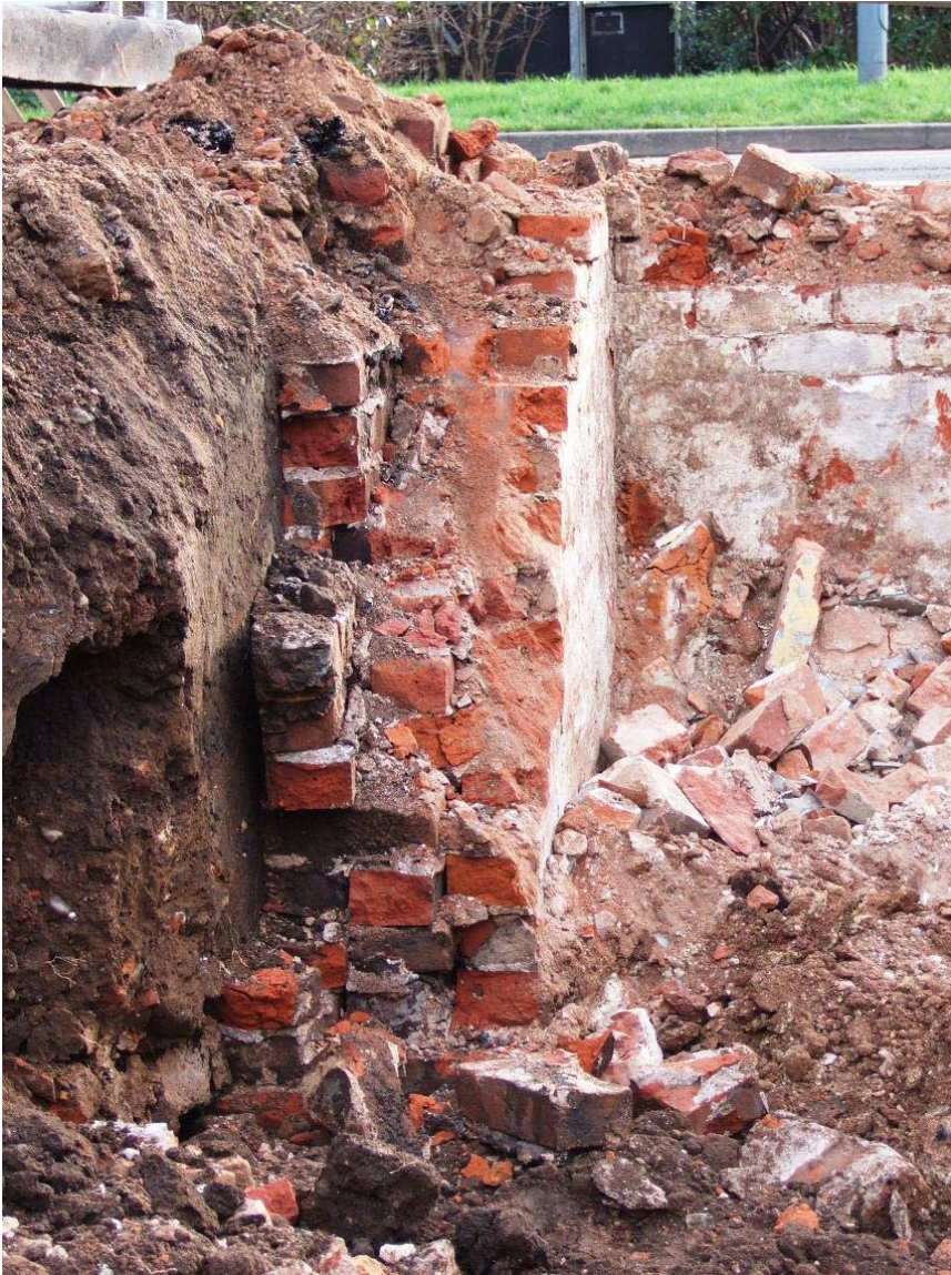
7. Detail of construction of eastern basement wall
