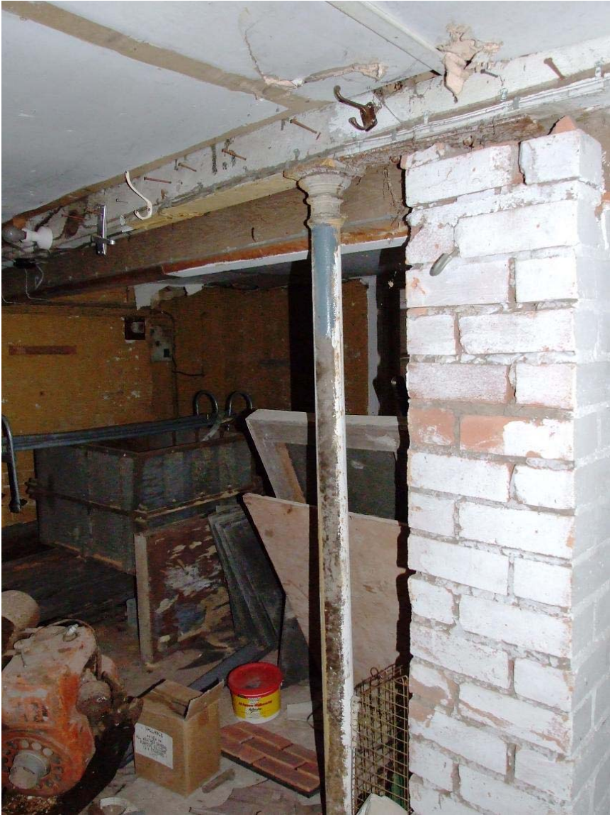
14. Basement, central spine beam and later strengthening
