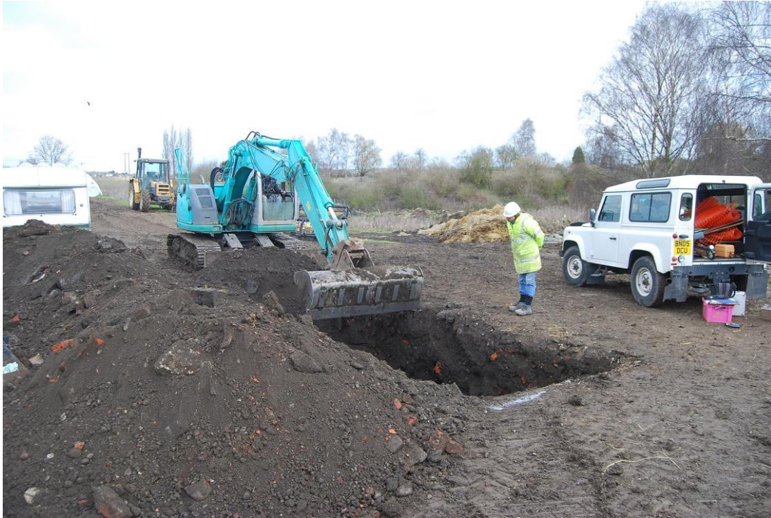
Plate 1, Excavation of the trench, view north-east
