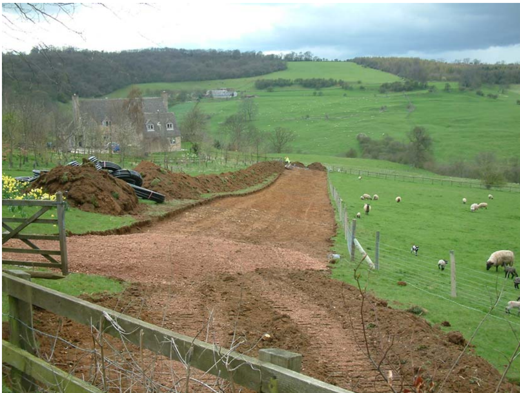
Plate 2: Field 1 after excavation, facing west
