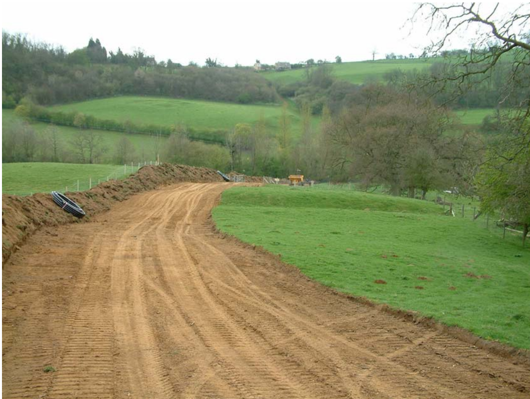
Plate 5: Field 3 after soil removal, facing south
