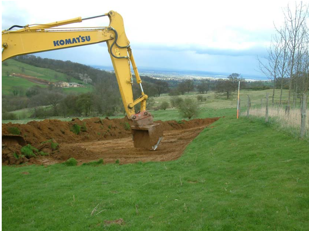
Plate 3: Field 2 during soil removal, facing north
