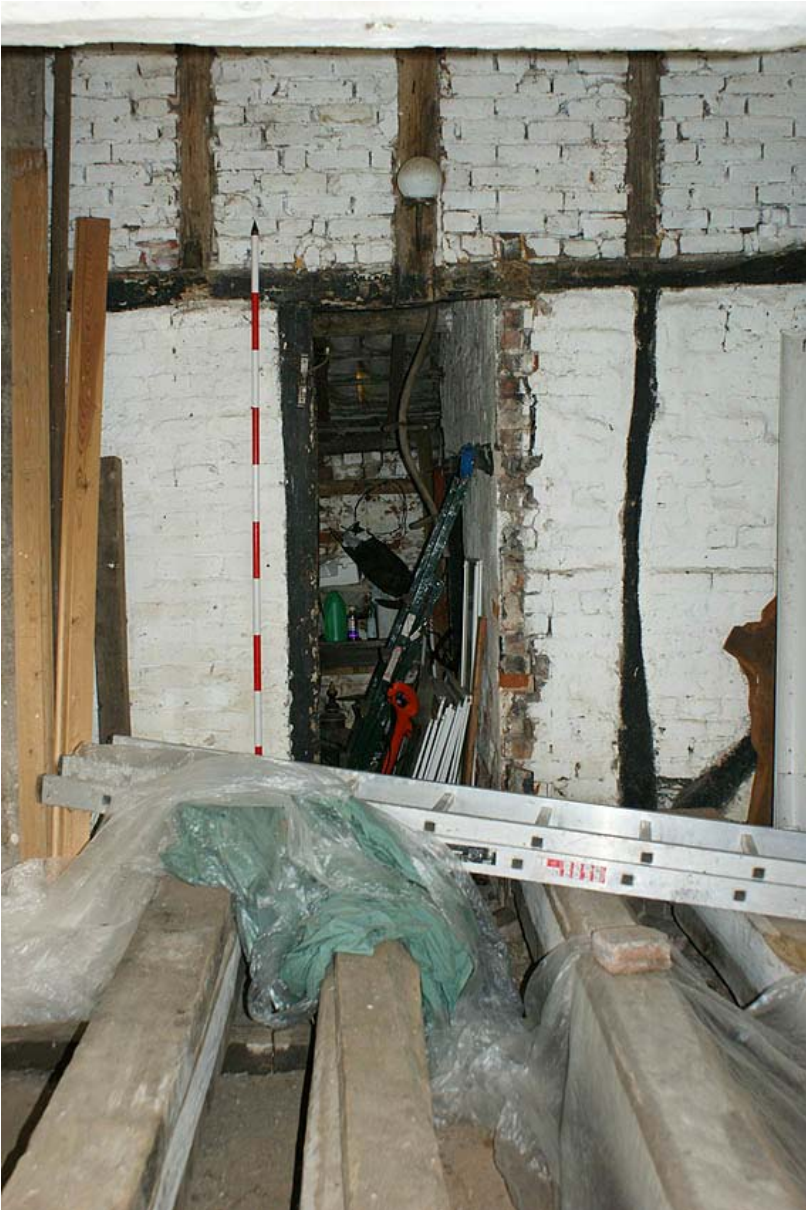
Plate 19: Inserted opening into brick extension, from the east
