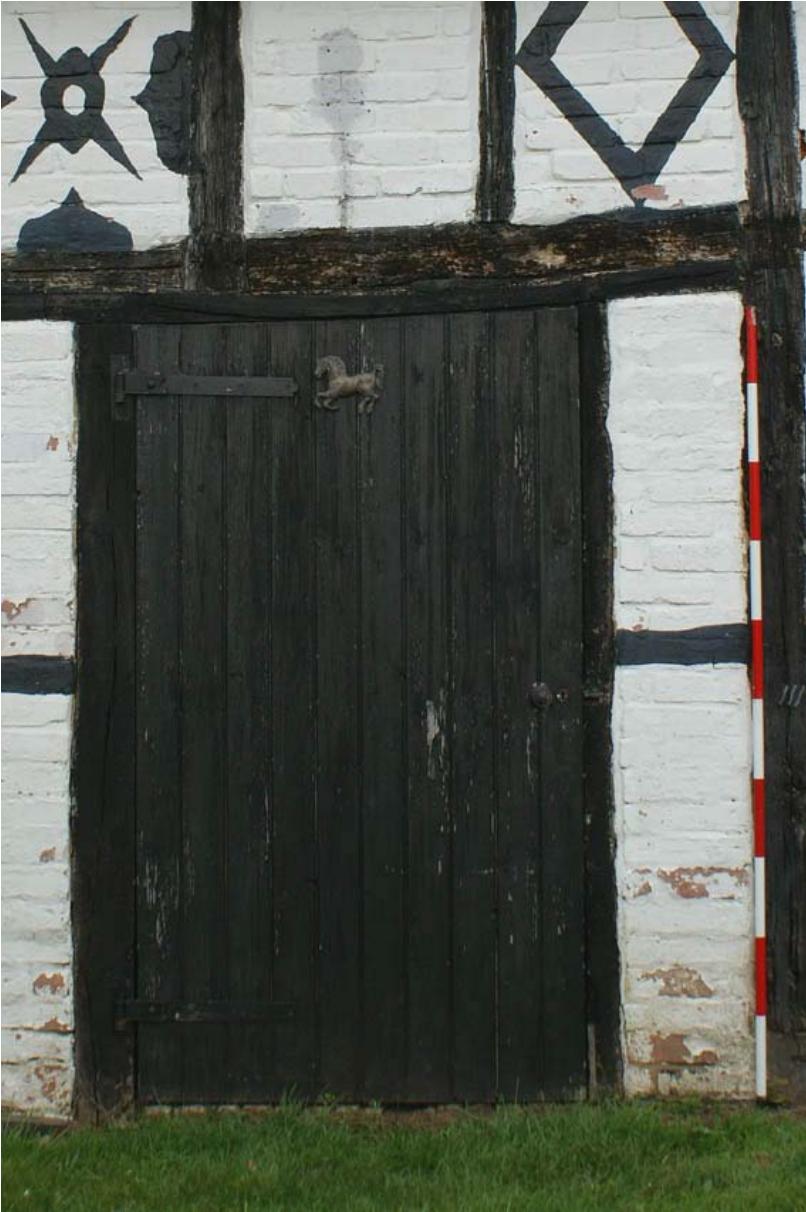
Plate 20: Large door on south elevation of building, from the south
