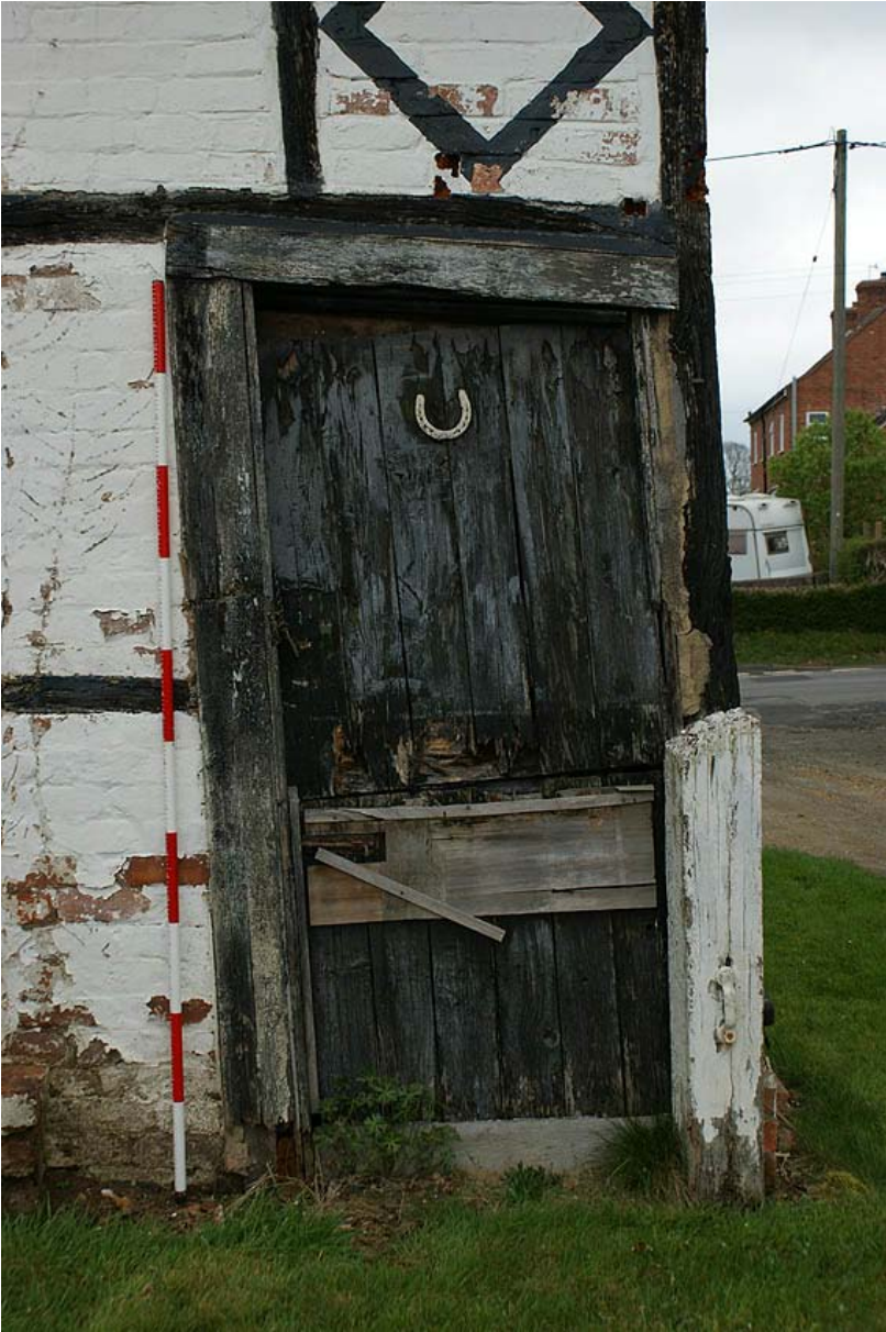
Plate 18: Former doorway into the building, from the south
