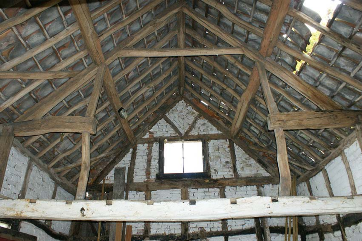
Plate 7: Truss 2 of the building from the east
