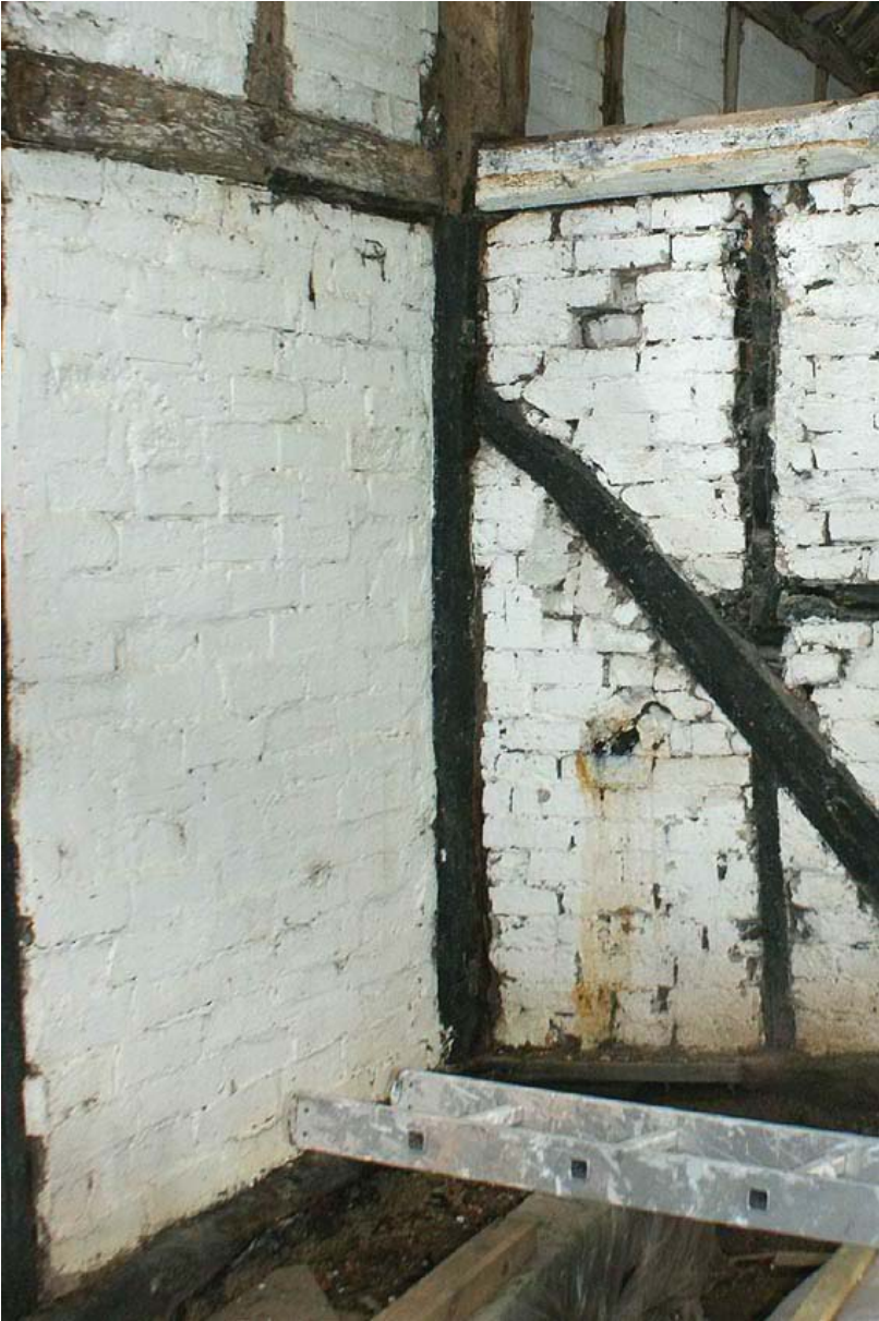
Plate 11: North elevation internal pintles (on post in centre)
