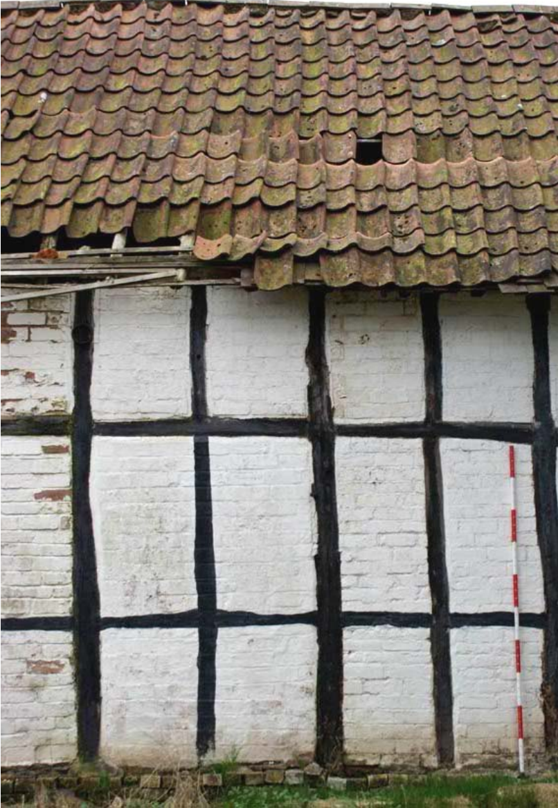
Plate 9: North elevation, blocked opening
