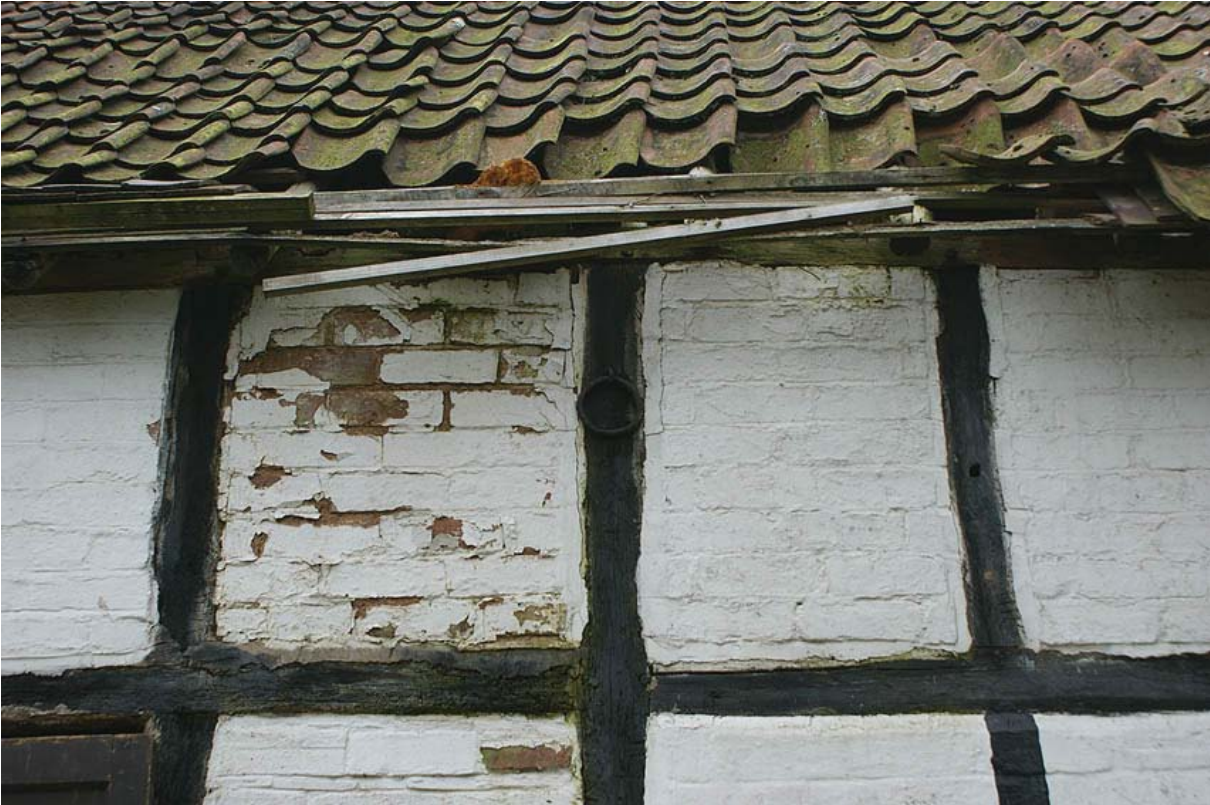
Plate 21: Tethering ring on north wall of building, from the north
