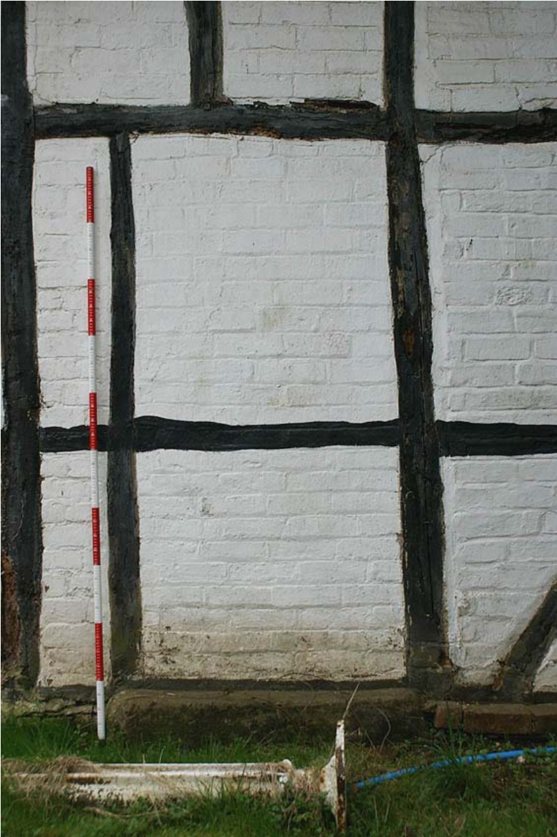
Plate 17: Doorway and step on north side of the building, from the north
