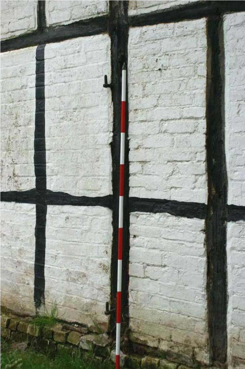
Plate 10: North elevation pintles
