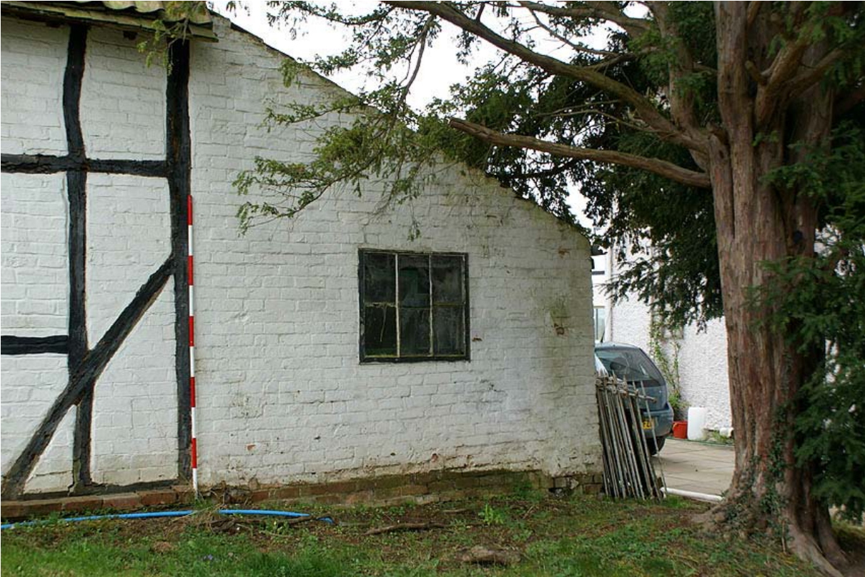
Plate 16: Brick extension from the north east
