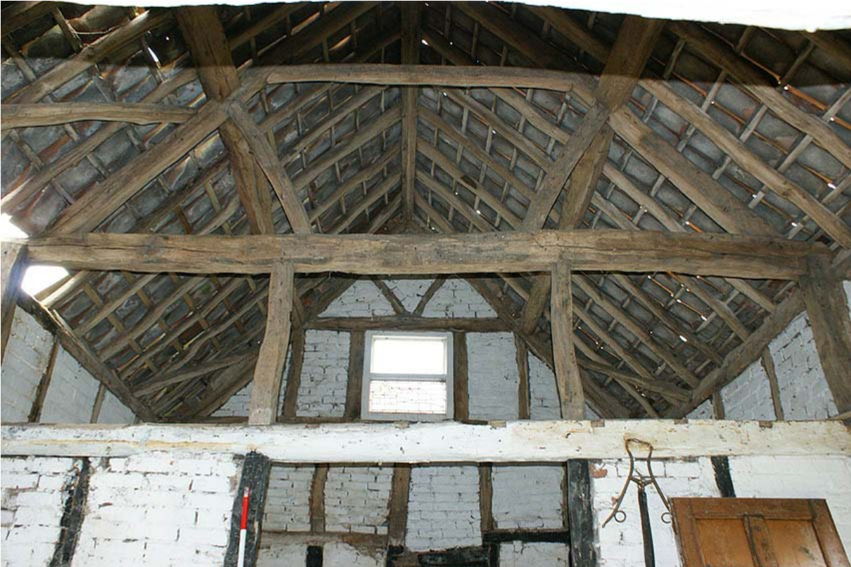
Plate 8: Truss3 of the building from the west
