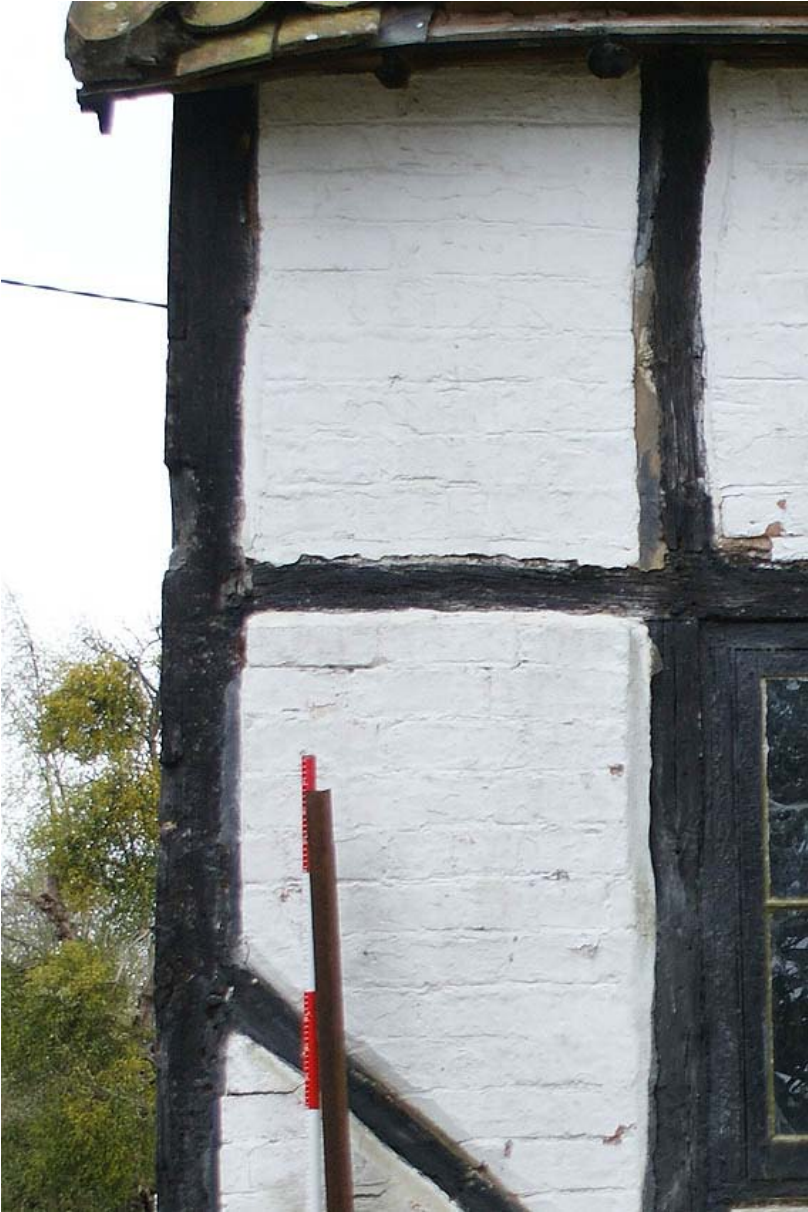
Plate 6: Construction notch on north east corner of building
