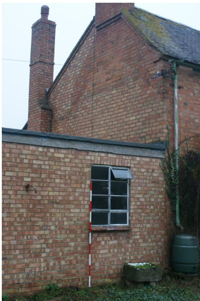
Plate 9 Former gable of demolished building visible in the brickwork, looking north
