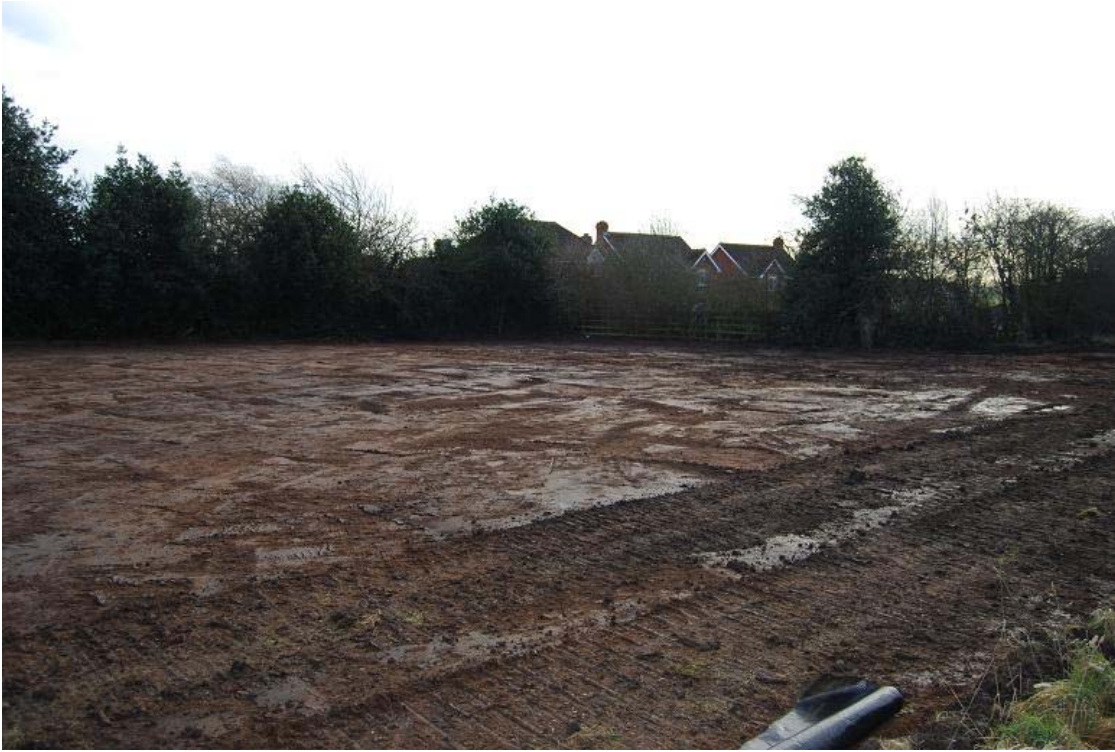
Plate 3: The site following completion of the strip, from the south east
