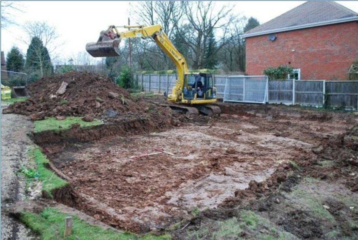
Plate 3 View of south-east side of the building looking west
