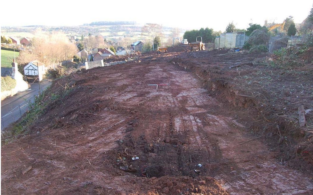
Plate 2, soil strip in progress toward frontage and modern pits, view east
