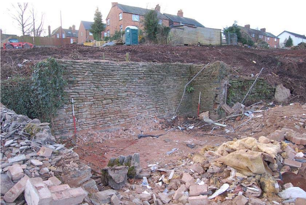
Plate 4, revetting wall to rear of No. 77 post-demolition, view south-west
