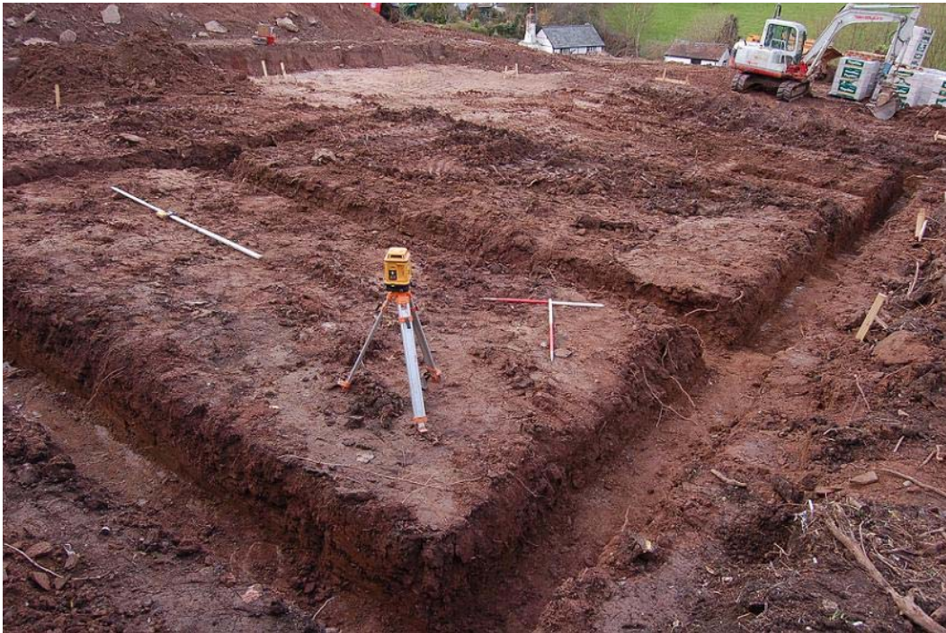
Plate 16, foundation trenches in south-east corner of site, view west
