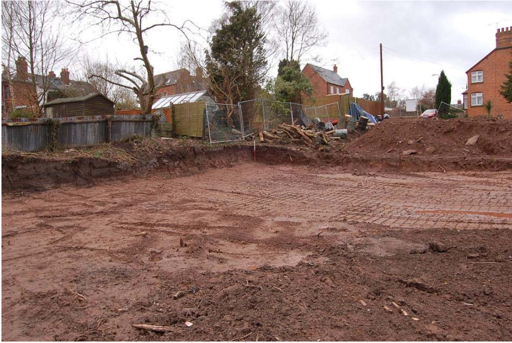
Plate 15, site strip in south-east corner, view south
