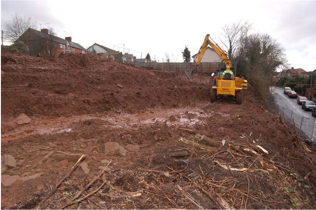
Plate 7, access road strip in progress off frontage, view south-west
