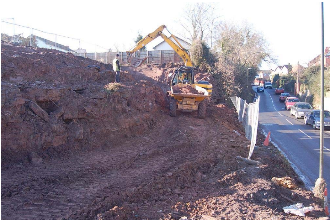
Plate 8, site strip in progress along frontage, view south-west
