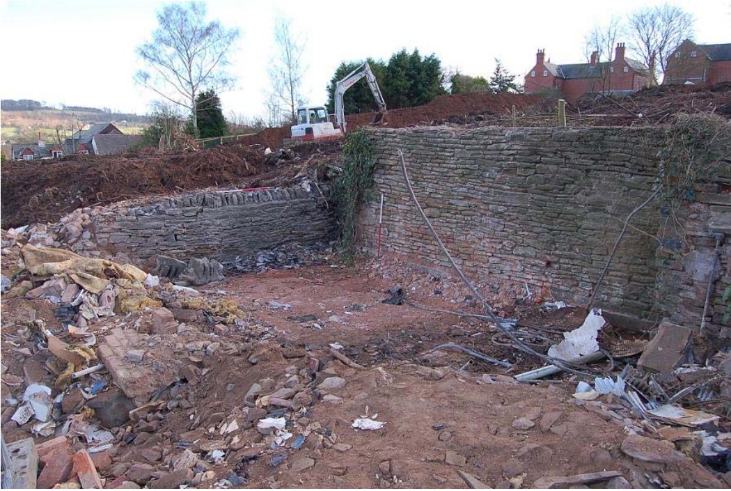
Plate 3, revetting wall to rear of No. 77 post-demolition, view south-east
