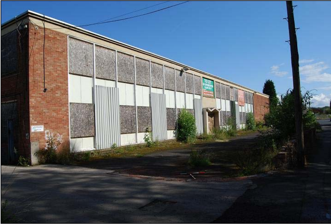
Plate 13: The carpet factory, built in the 1960s on the frontage of Clensmore Street, view northwest
