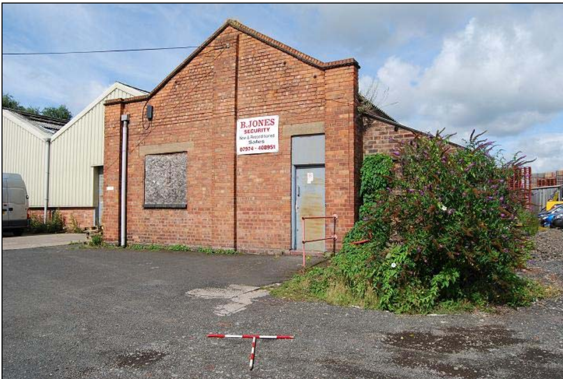
Plate 24: The mid 20 th century building (Unit 25c) south of the Pallet Return System Depot, view west
