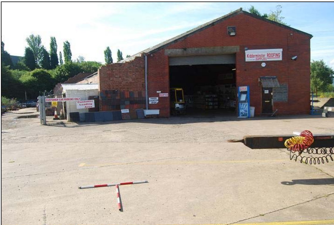
Plate 12: View of the building constructed in 1960 (Unit 23), view south
