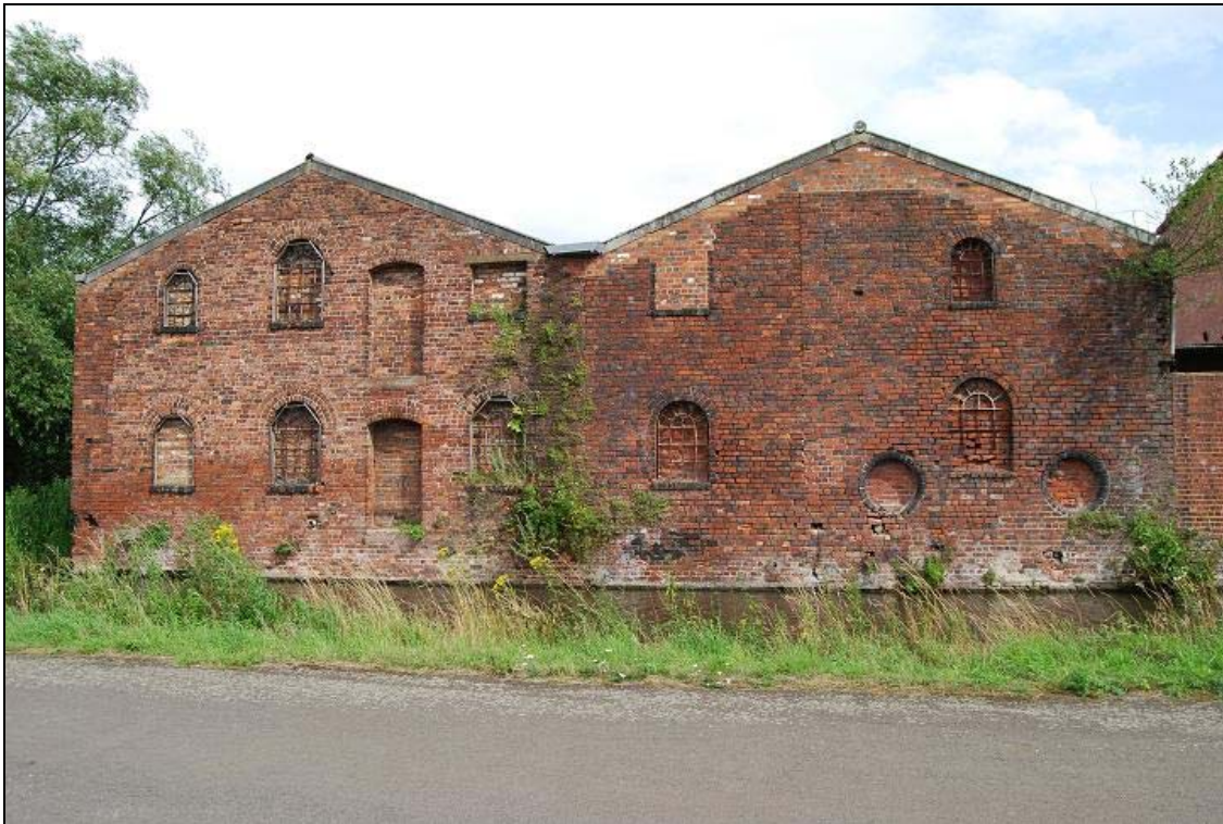
Plate 18: West elevation of the early 19 th century former corn mill (WSM 36224; see also Plate 27)
