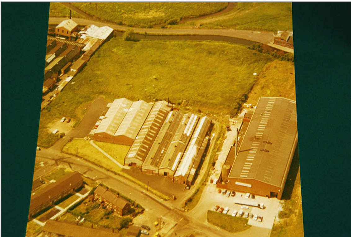
Plate 10: Aerial northwest view of the central portion of the site and the 1960s/1970s buildings, with the frontage of Stoney Lane in the foreground, 1975 (accession no 318115)
