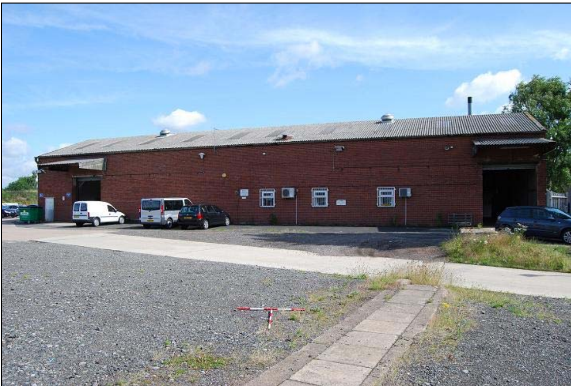
Plate 20: CMS Vauxhall preparation centre, 1970s buildings, view north
