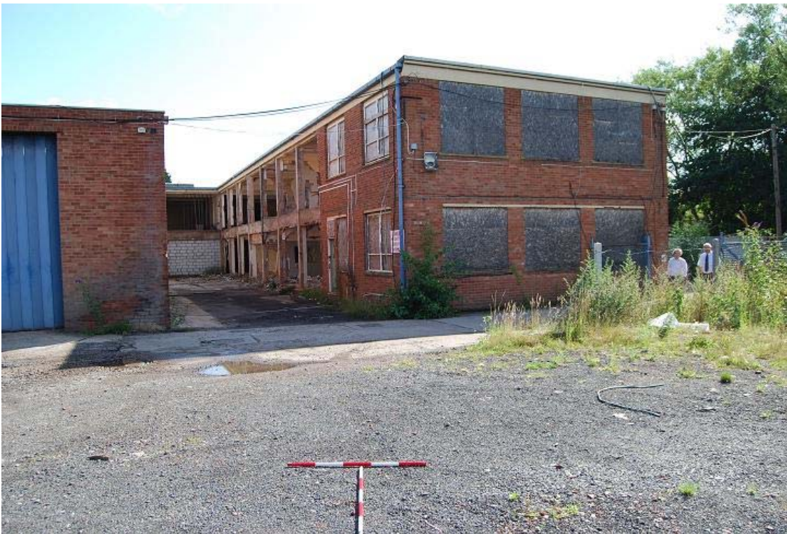
Plate 14: Northwest elevation of the 1960s carpet factory building
