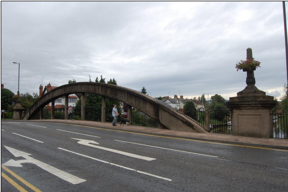
Plate 2: West arch, vertical ties, piers and the iron parapet
