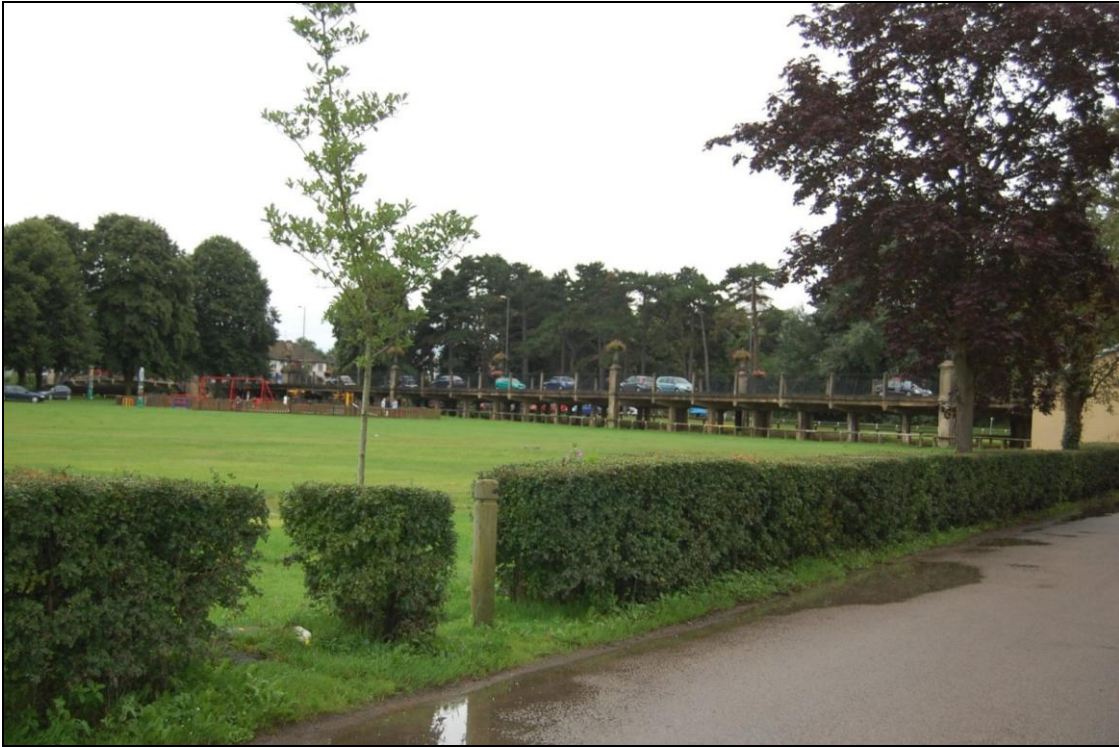
Plate 3: View north-east of the viaduct from the footpath
