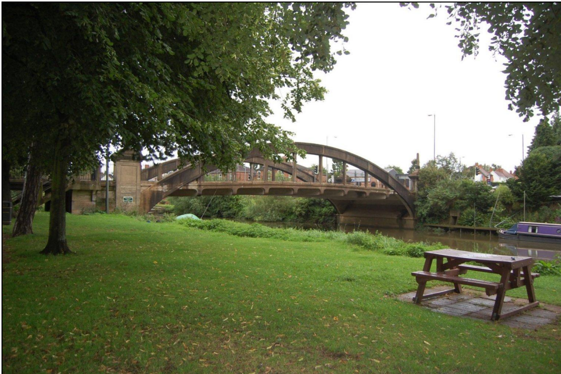
Plate 1: View north-west of the bridge from the south bank
