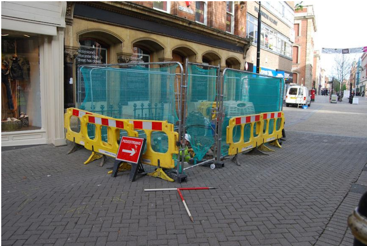
Plate 1: General view of Trench 3 from the south
