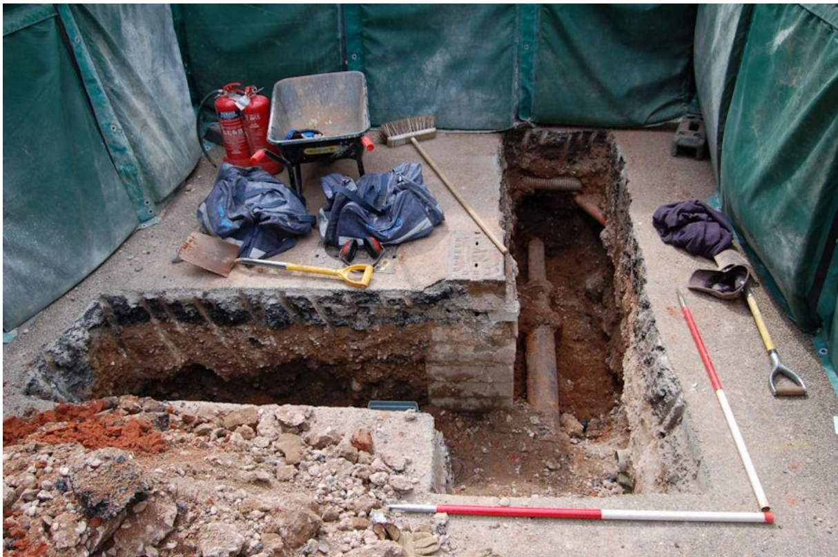
Plate 6: General view of Trench 15 from the south
