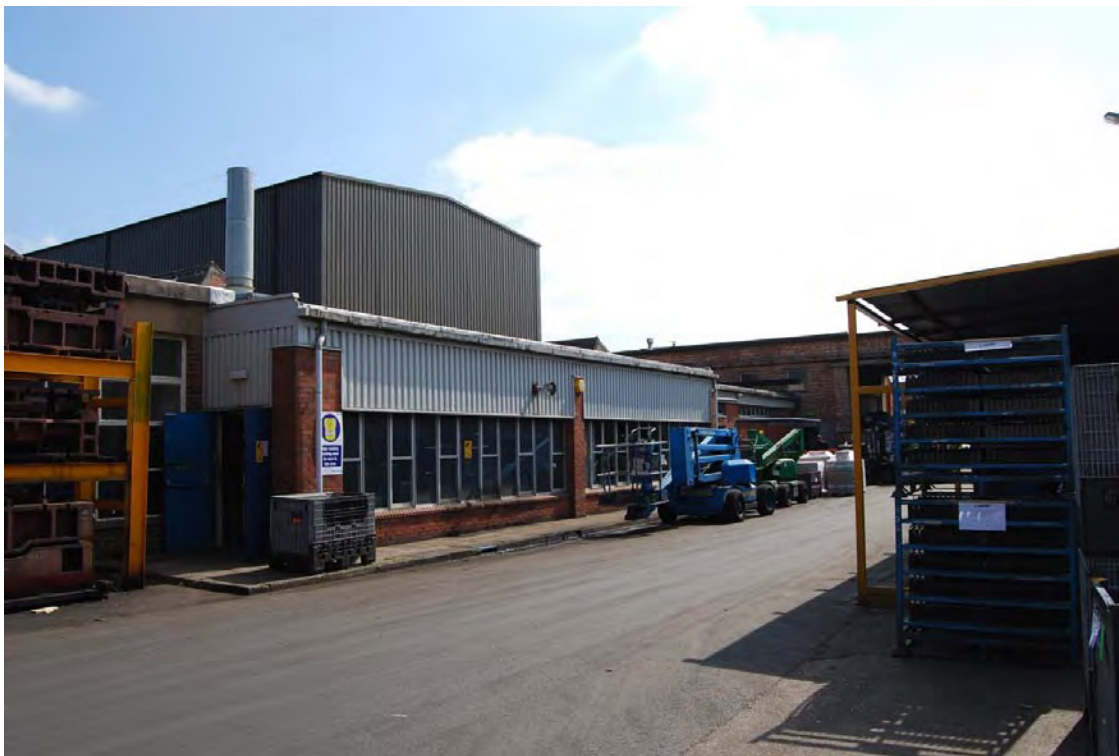
Plate 10: Buildings on west side of factory
