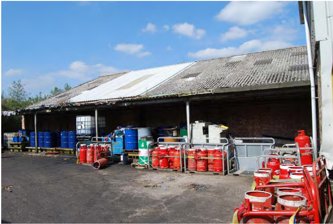
Plate 11: Building to west of factory, facing north-west
