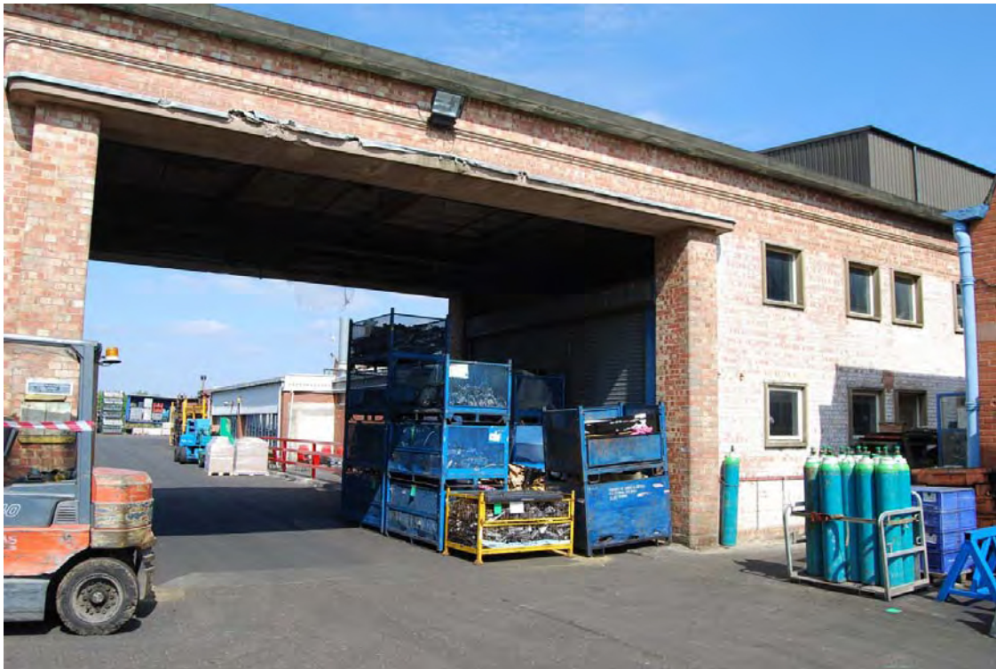
Plate 12: Building and throughway on west side of factory
