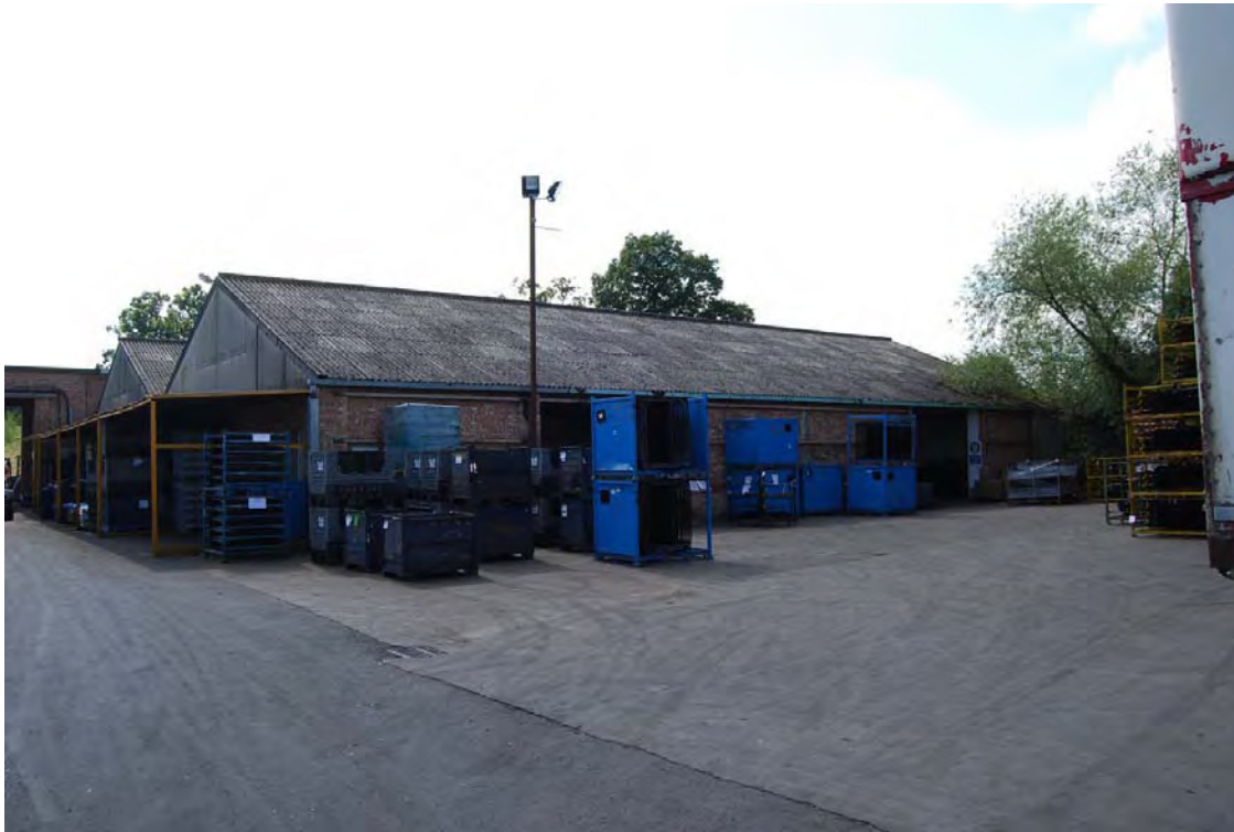
Plate 9: Building to west of factory, facing south-west
