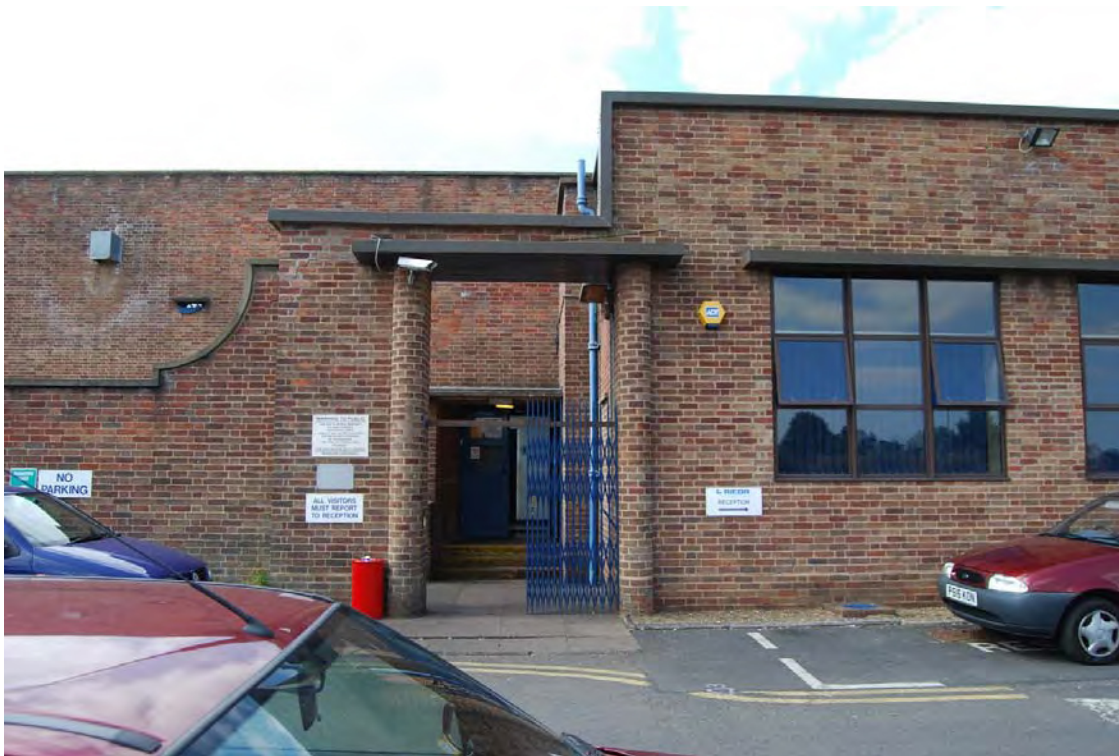
Plate 6: Entrance in south side of front elevation
