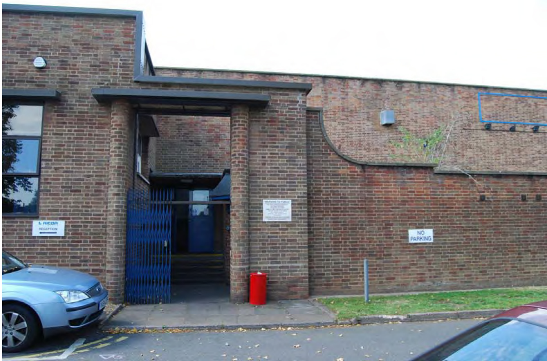
Plate 5: Entrance in north side of front elevation
