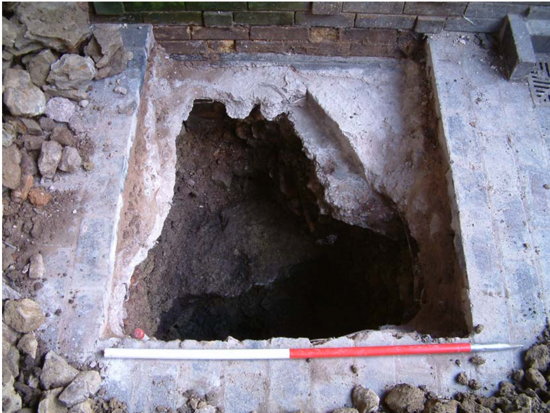
Plate 3: present brick surface, underlying concrete slabs and large concrete footing in base of excavation, facing east
