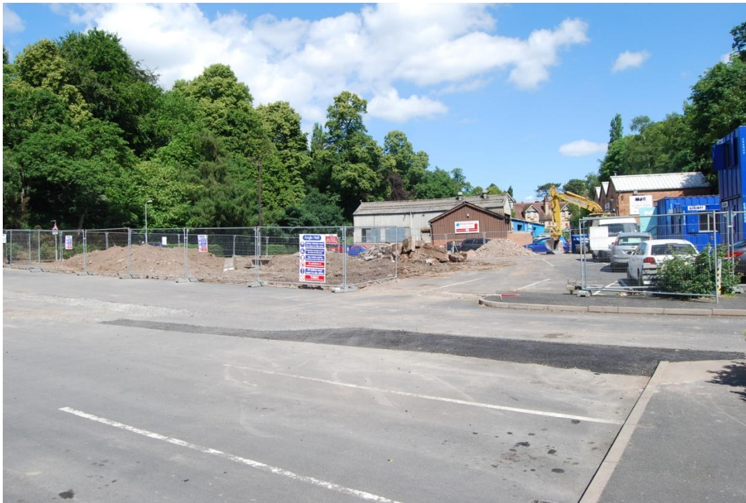
Plate 2 General view of development site, looking north-east
