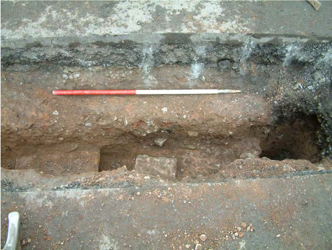
Plate 3: Trench 3, facing north. Cast iron pipes to the left and service trench to the right, the heavily truncated remains of possible sandstone structure (310) in the centre
