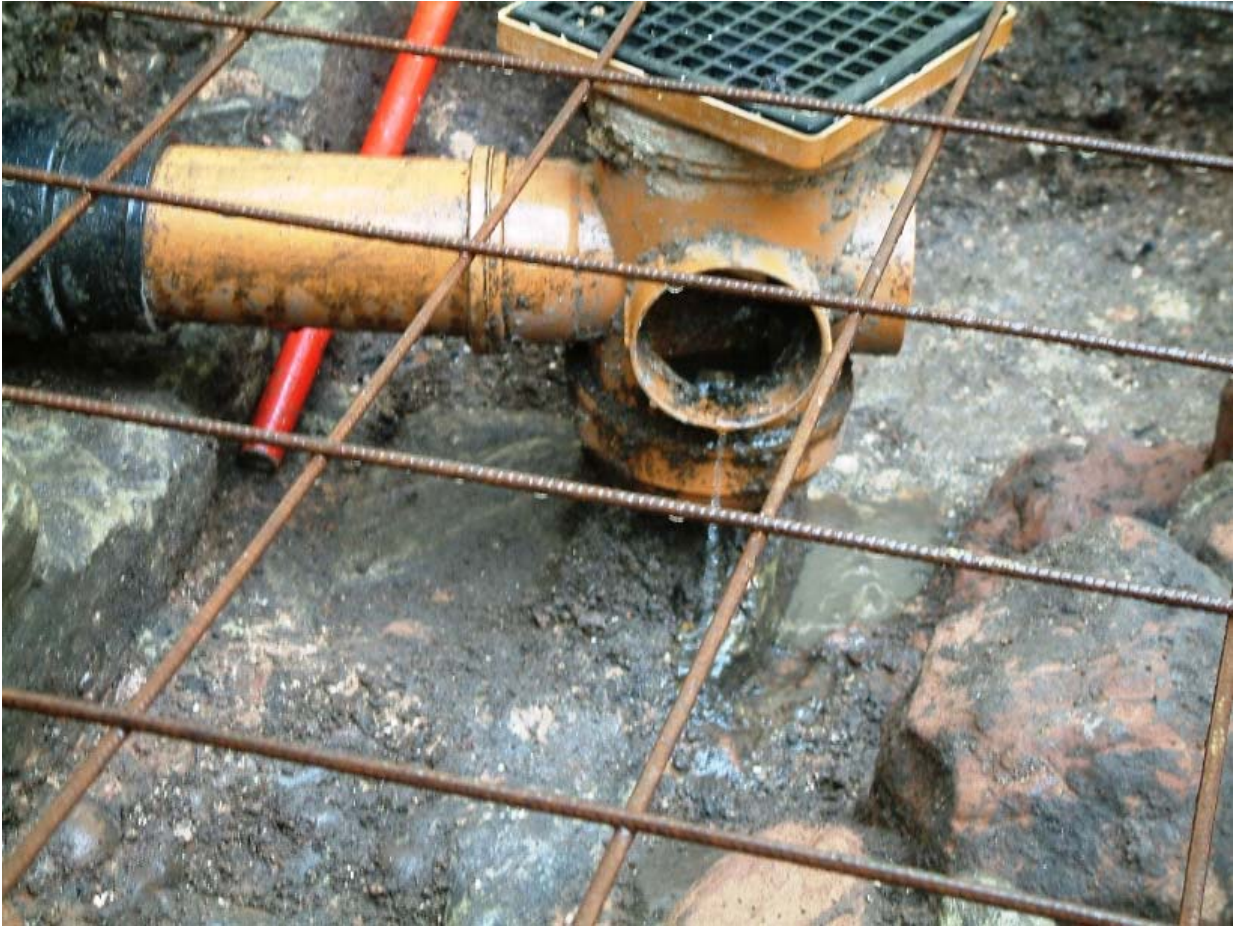
Plate 11 looking west: Test pit 3 showing uncapped end of surface drain, during light rain, discharging into archaeological deposits and against the foundations of Commandery House to the left.
