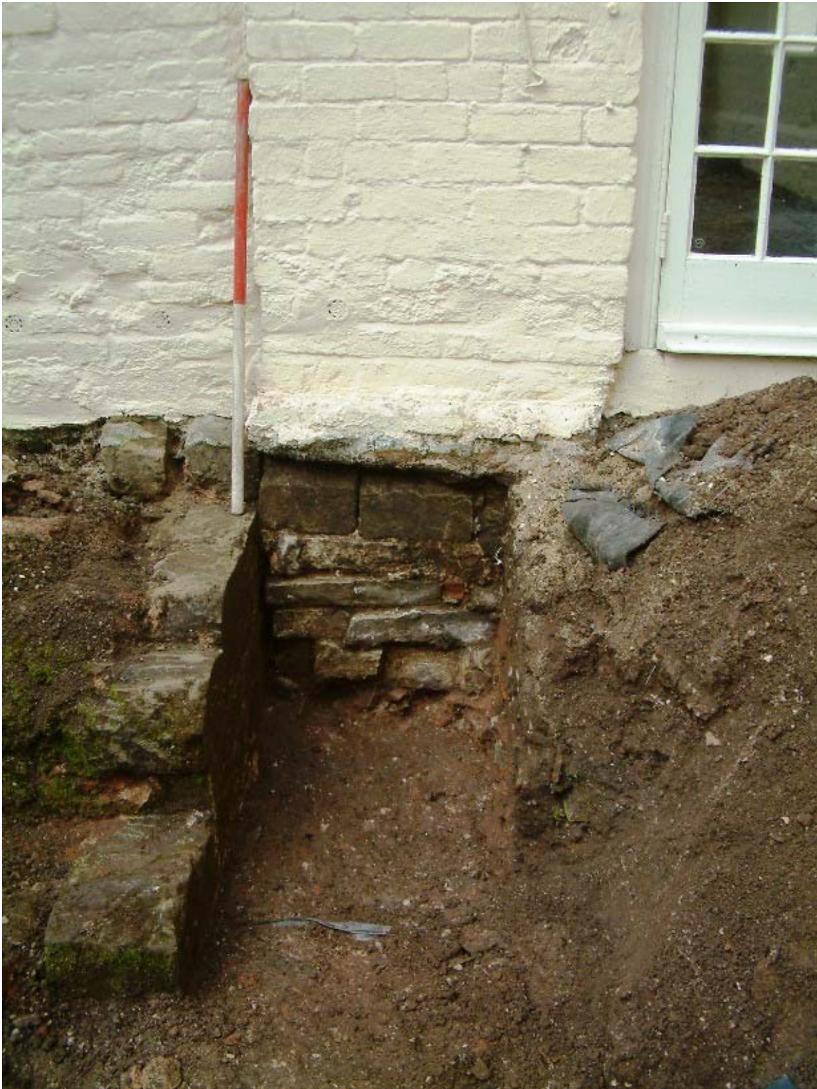
Plate 7 looking west: Test pit 2. The brick wall of the East Range extension (late 17 th century) sits directly upon the surviving chapel wall and abuts the late 15 th century East Range (at photo scale location) and continues to the left of the photograph.
