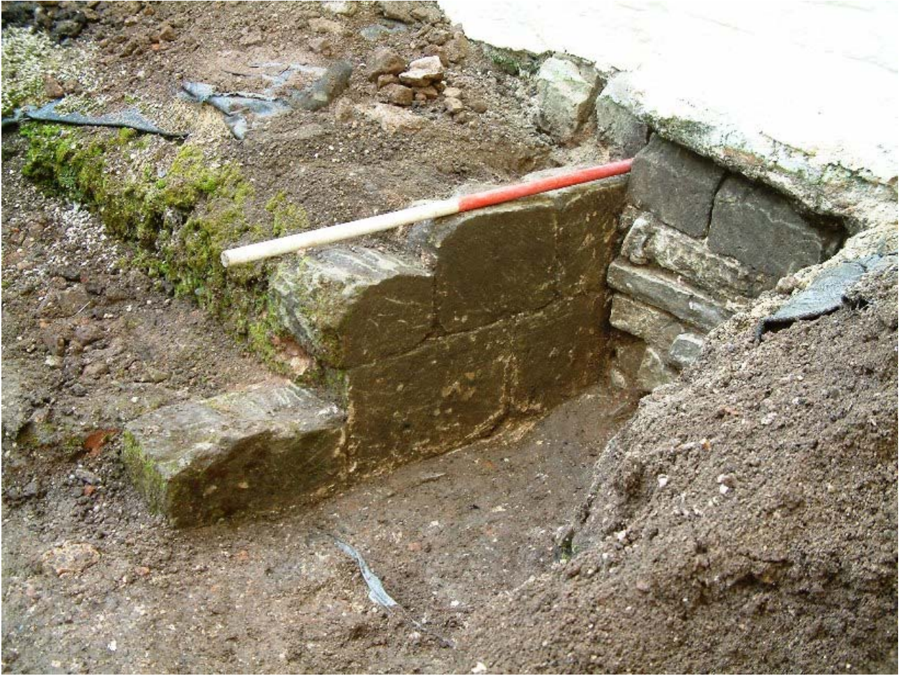
Plate 6 looking south west: Test pit 2 with exposed north wall of 13 th century chapel abutted by the exposed late 15 th century East Range foundation. The chapel wall here survives to just below the modern ground surface.
