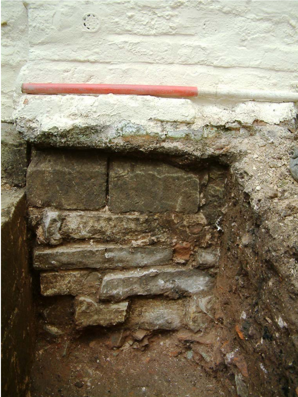
Plate 5 looking west: Test pit 2 with exposed late 15 th century East Range foundations abutting the 13 th century chapel wall to the left. The Lias foundations have settled into the pre-construction demolition layer (removed) which directly overlies a clay layer identified as part of the vestry floor. The photo clearly shows the chamfered green sandstone unitised in the final foundation coursing for the East Range overlaid by the late 17 th century brick re-facing.
