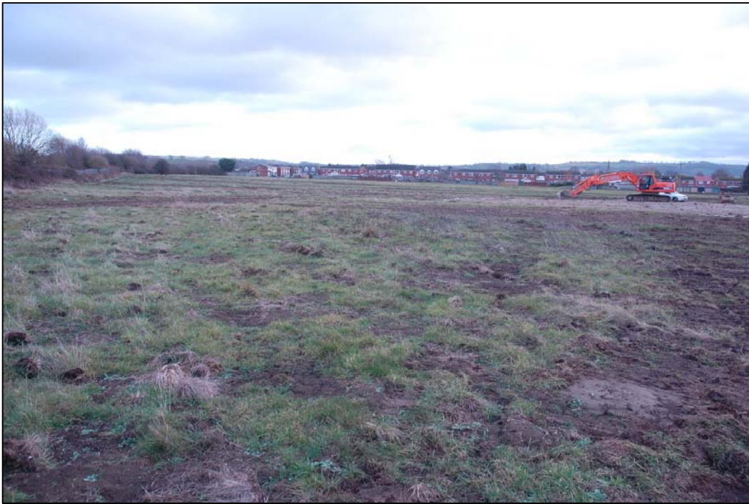
Plate 7: Backfilled trenches (Trenches 2, 3, and 4 facing south)
