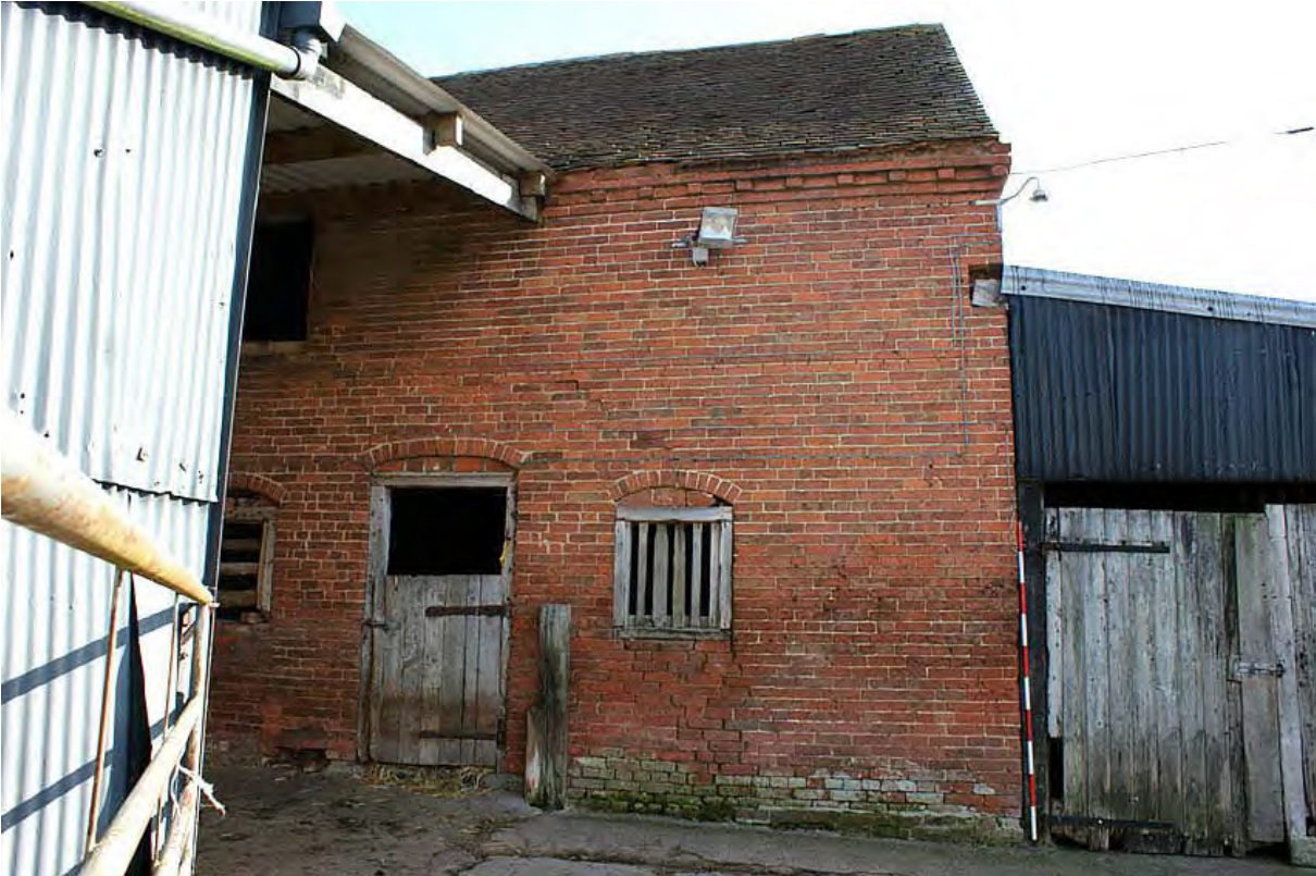
Plate 25: Building F, stable door and window, from the north west
