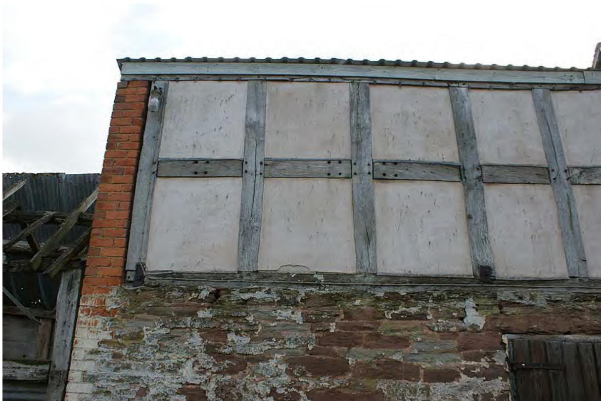
Plate 38: Building B from the north east showing re-used timbers
