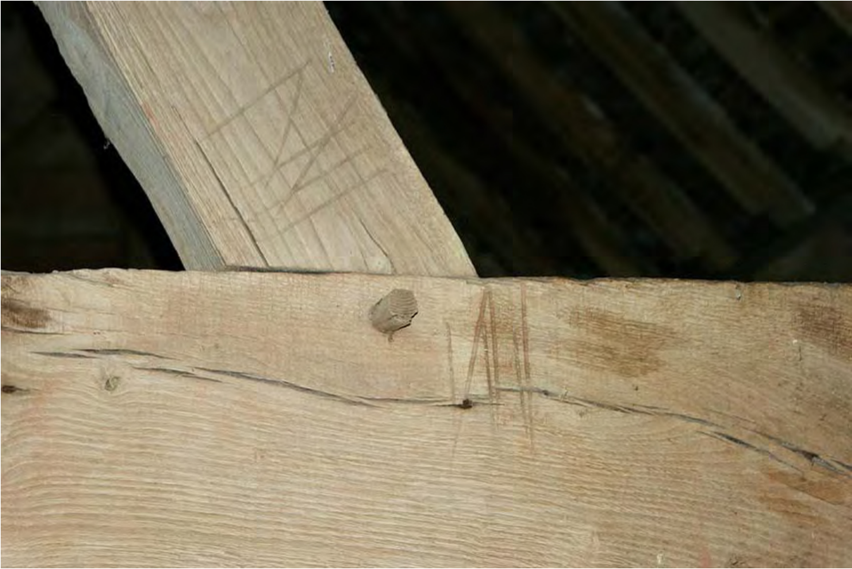
Plate 40: Carpenter's marks in Building C
