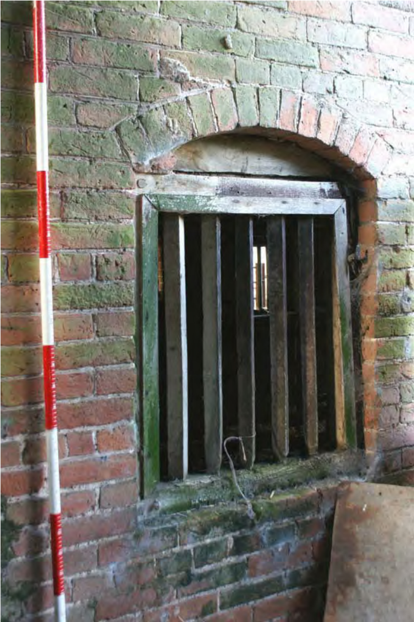
Plate 26: Building F, pegged window frame
