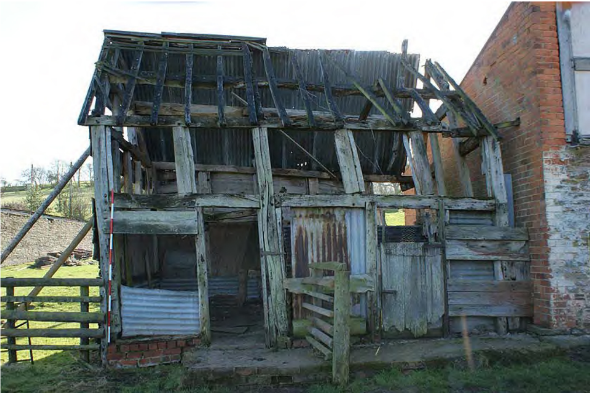
Plate 3: Building A from the north west
