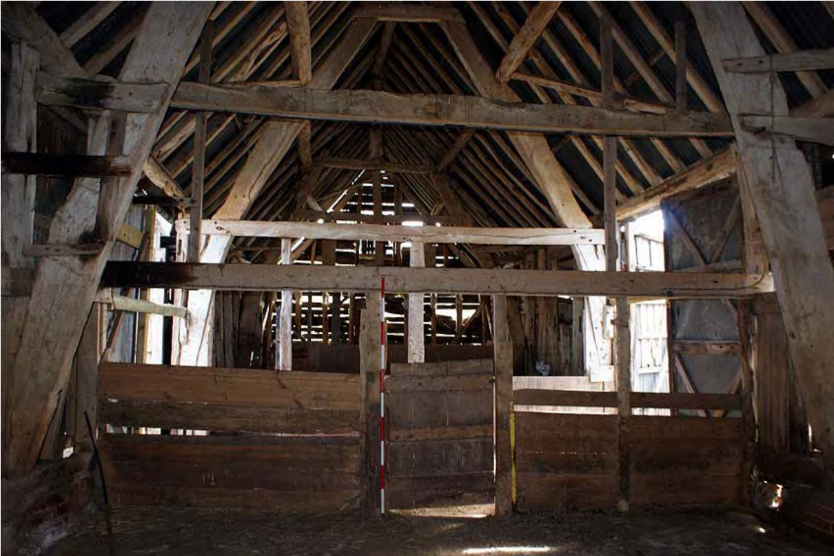
Plate 14: Building G interior showing cruck blade pairs
