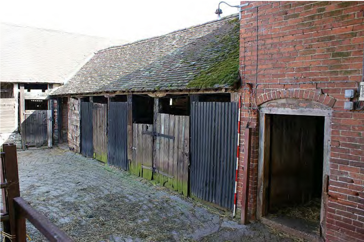
Plate 7: Building E from the west
