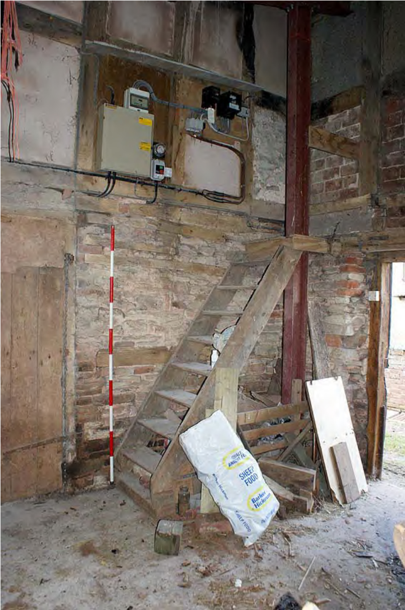
Plate 20: Building B interior stairs
