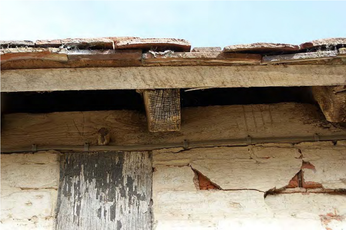
Plate 41: Carpenter's marks on wall plate of Buildings C and D
