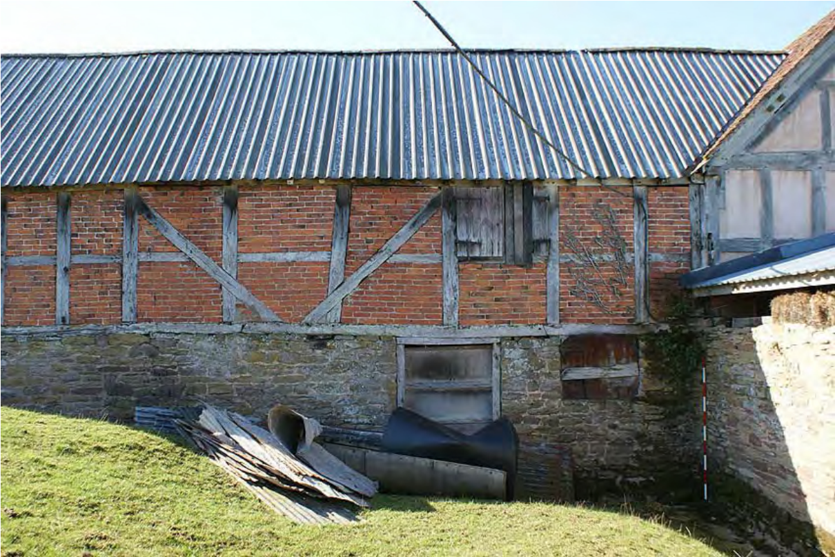
Plate 5: Building C from the north east
