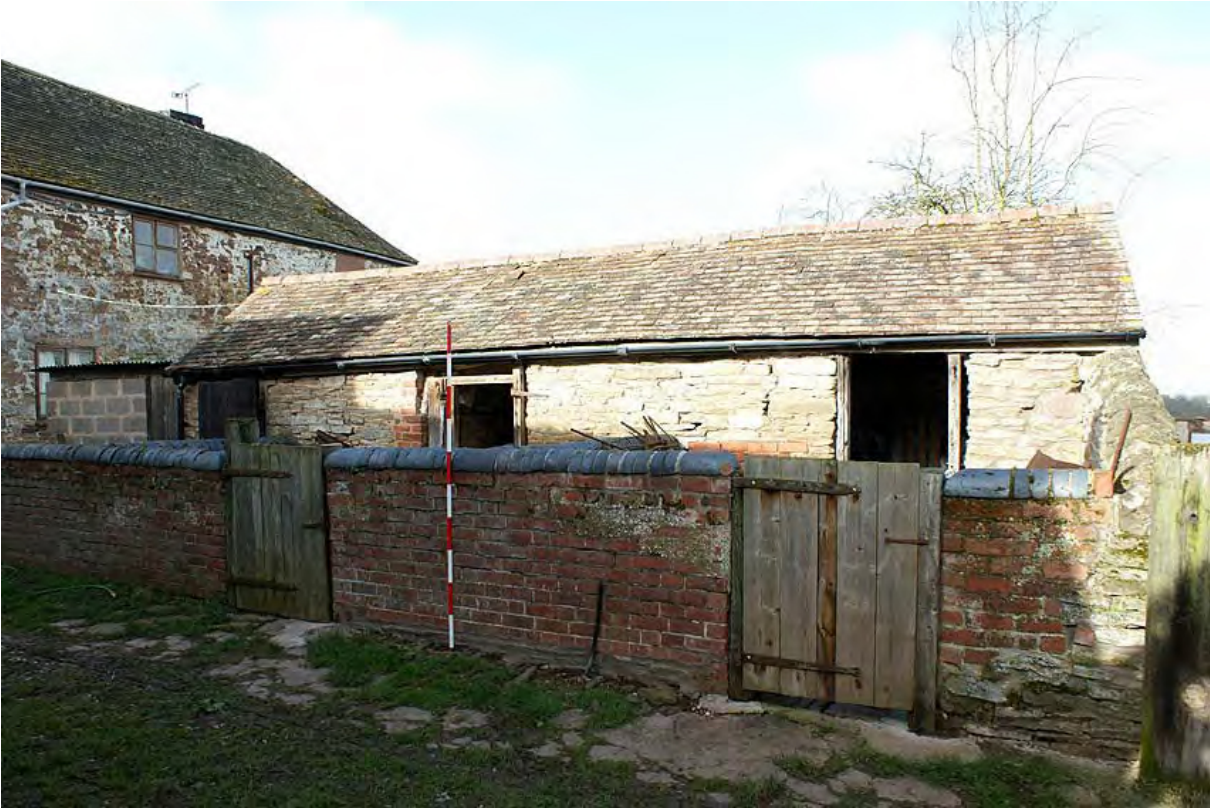
Plate 10: Building H from the south east
