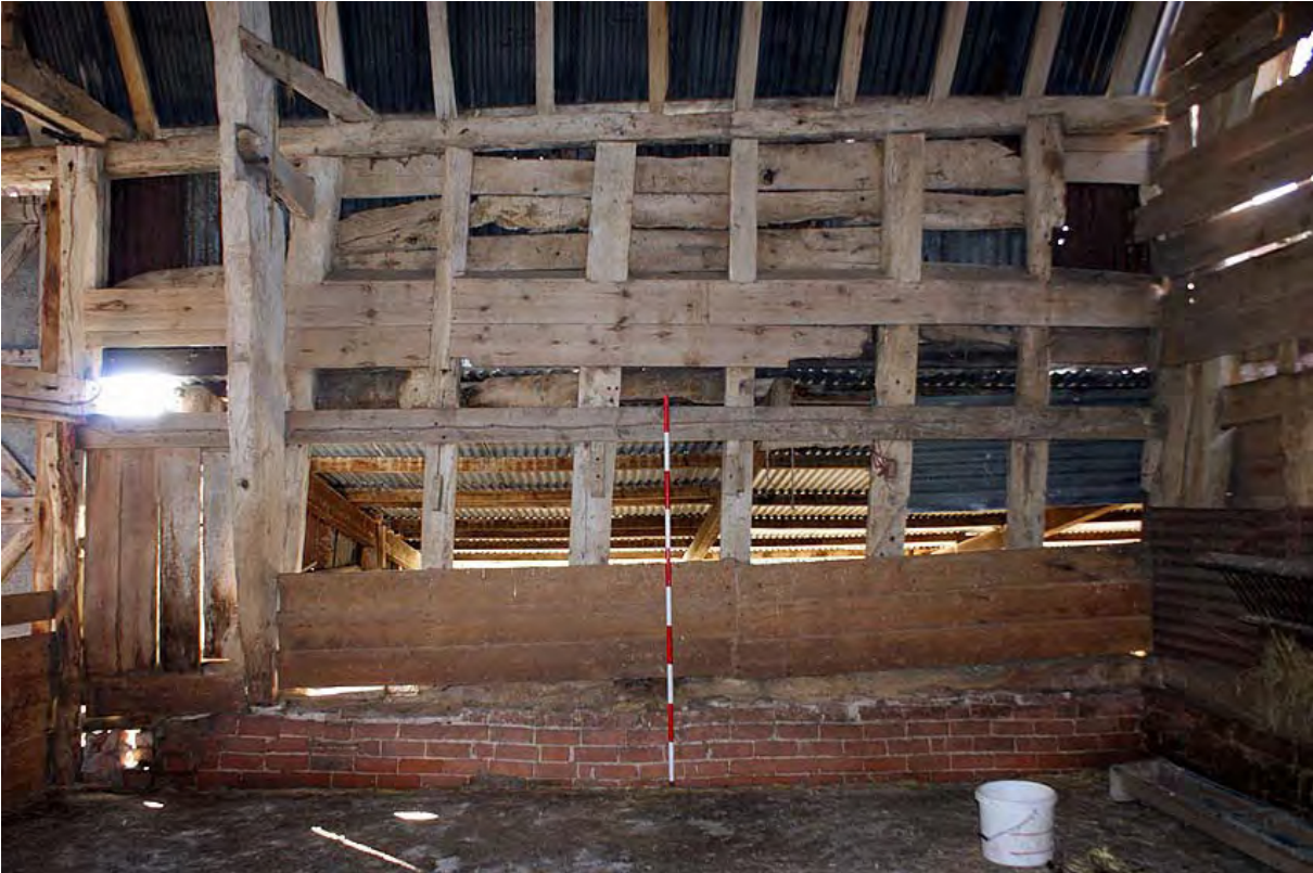
Plate 15: Building G side wall panels
