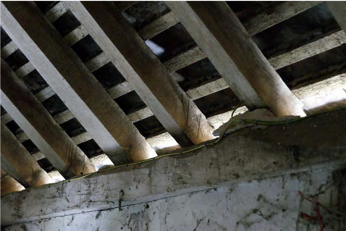
Plate 42: Carpenter's marks on rafters of Buildings C and D
