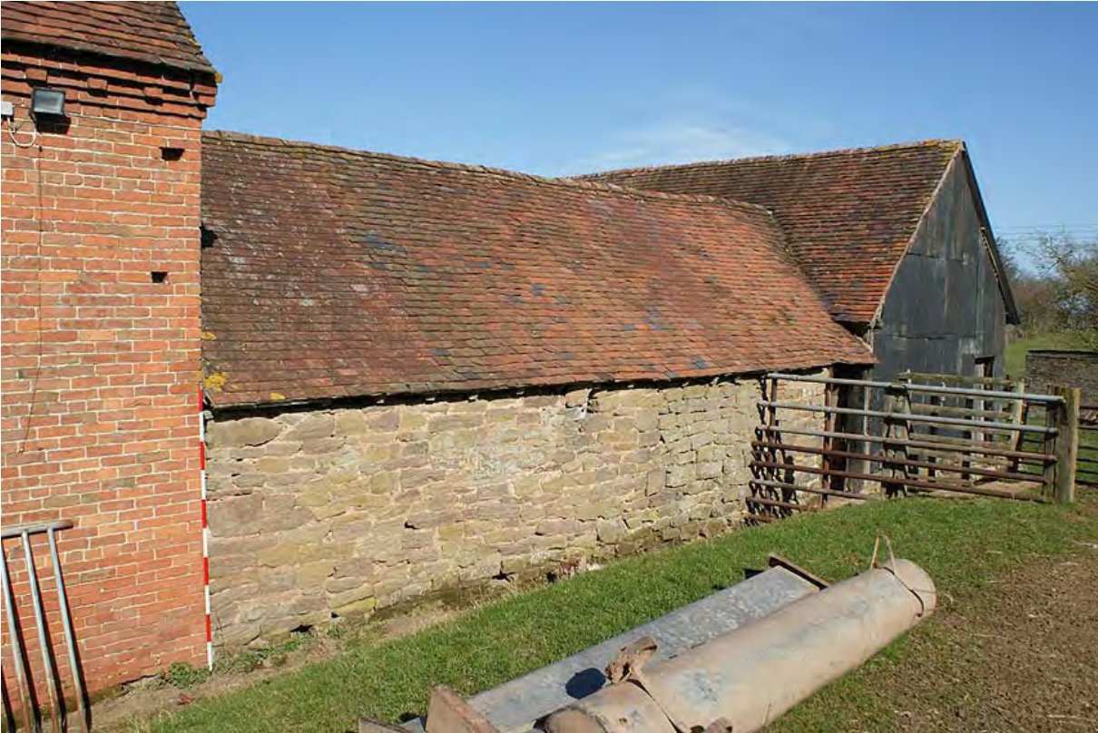
Plate 31: Building E rear wall from the south
