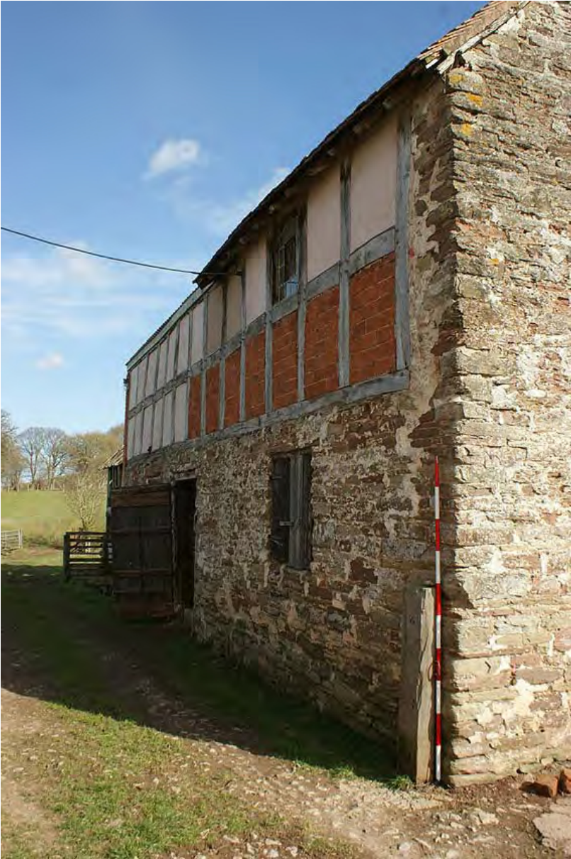
Plate 4: Building B from the west
