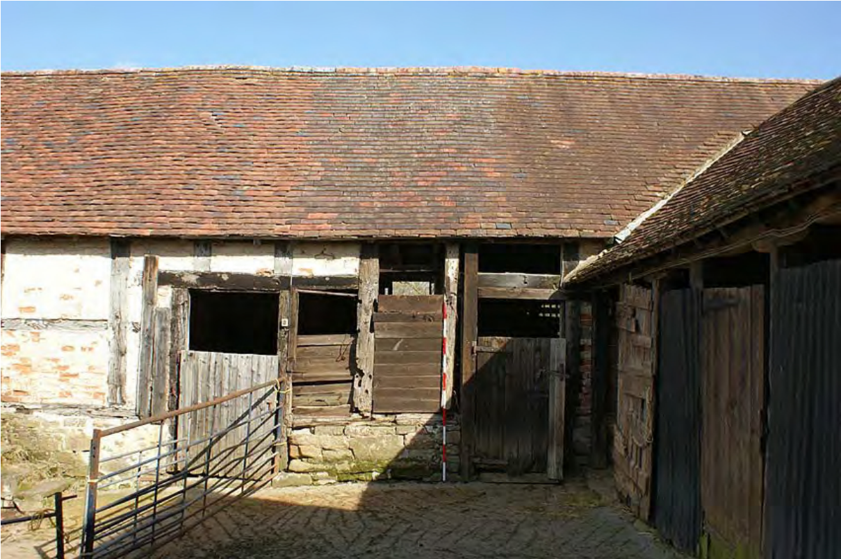
Plate 23: Building D from the south west
