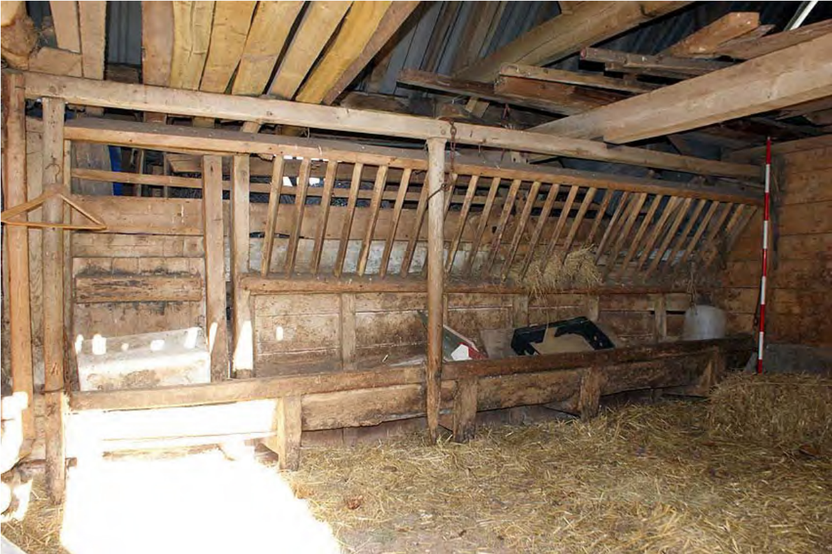
Plate 35: Building D, trough and hay rack
