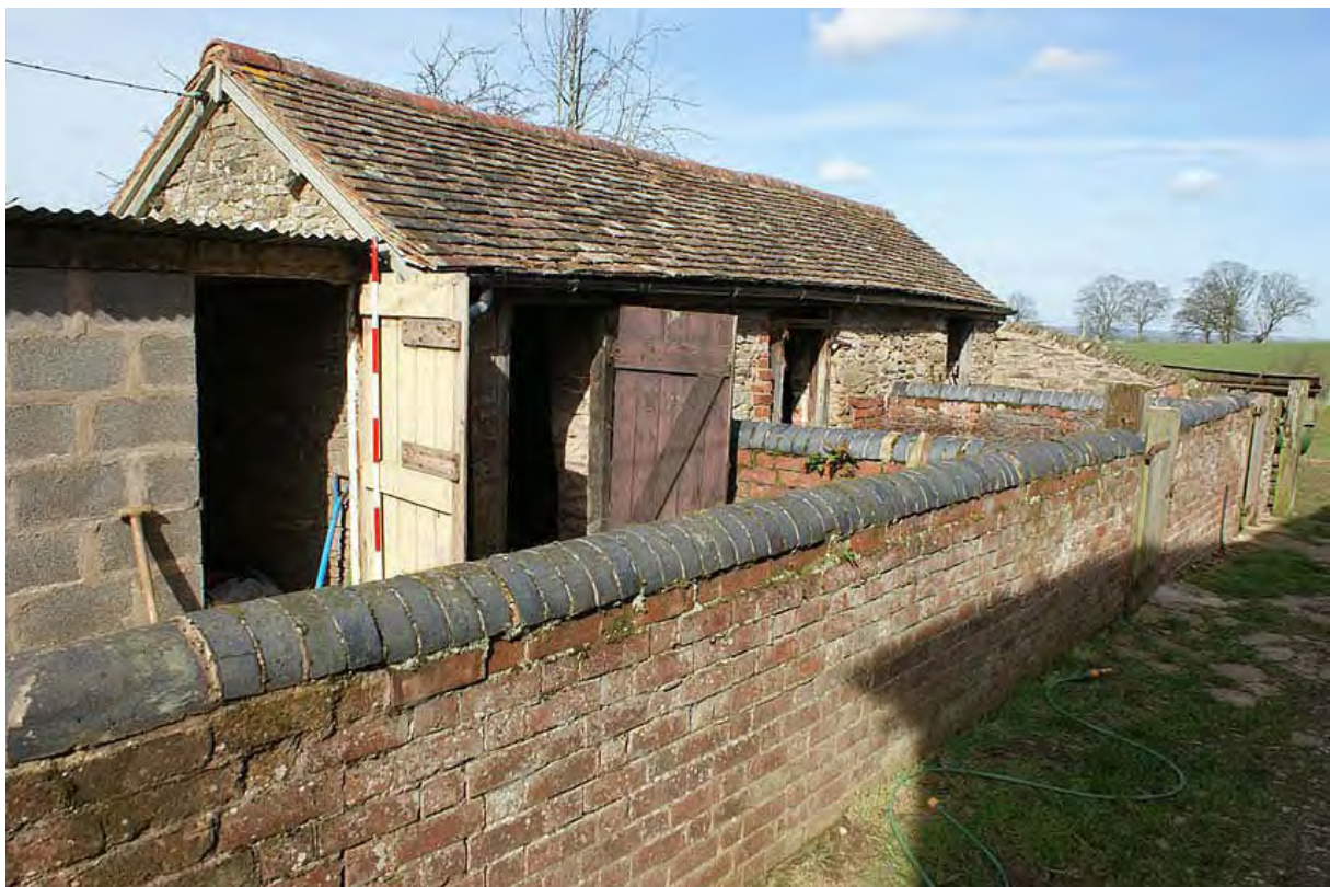
Plate 28: Building H, pigsty, from the south west
