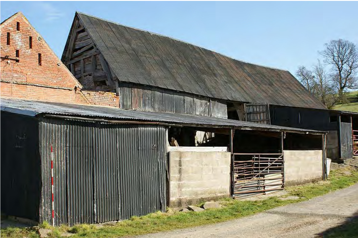
Plate 9: Building G from the north west
