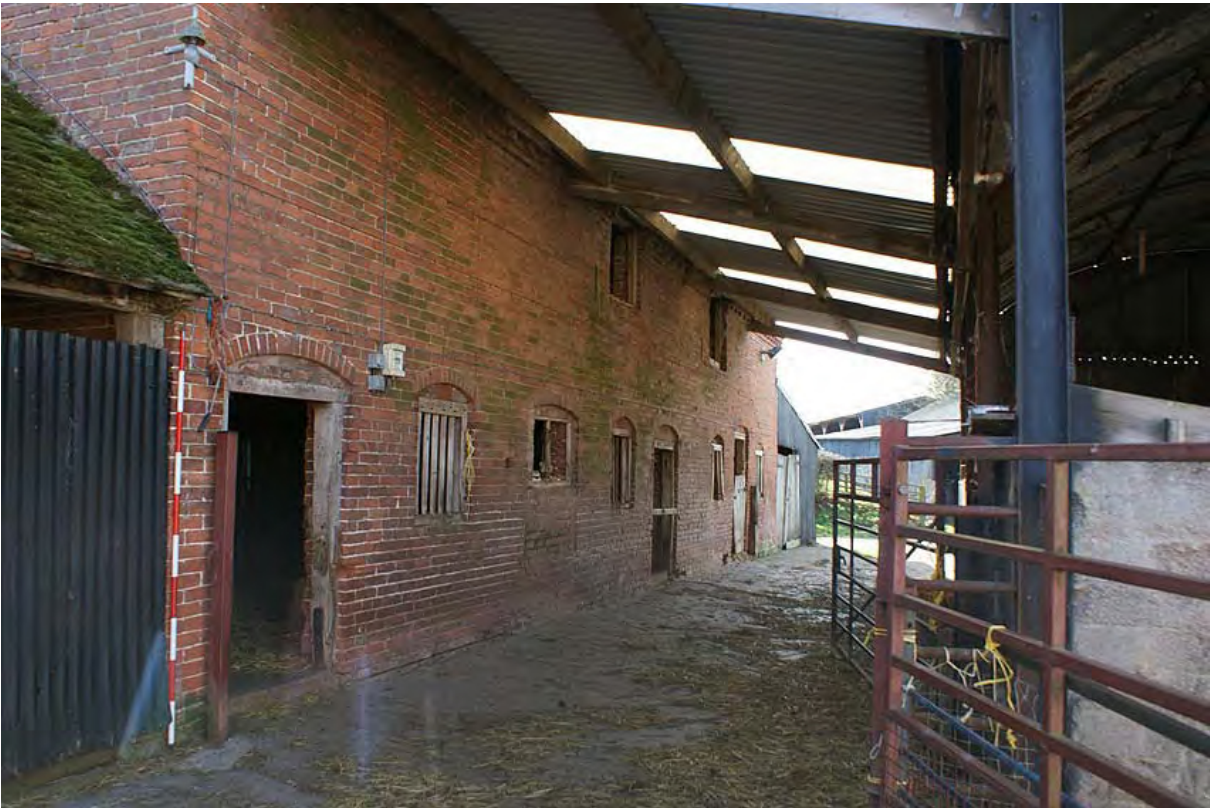
Plate 8: Building F from the north east
