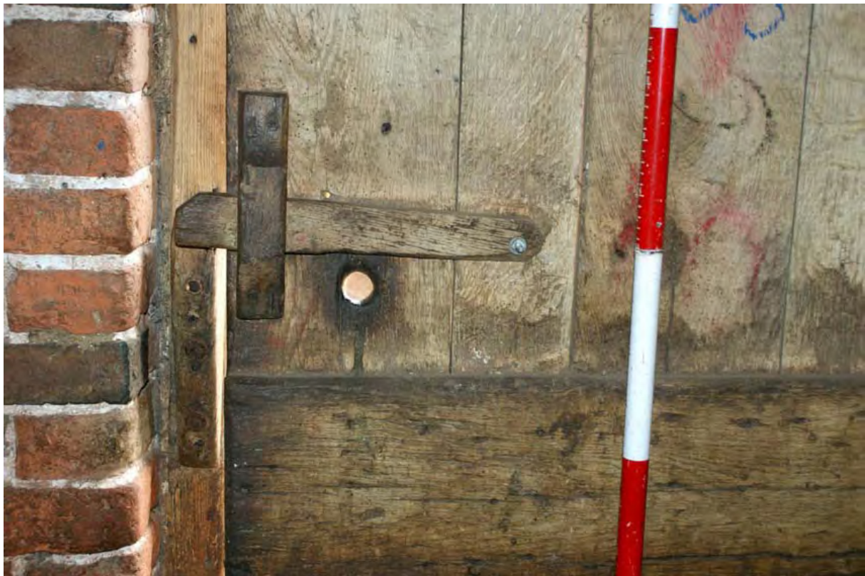
Plate 27: Building F, door latch and latch fastener
