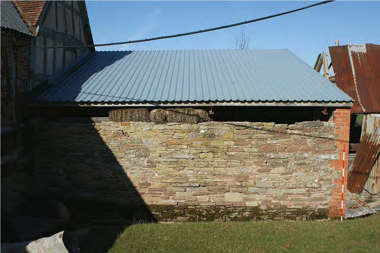
Plate 39: Building B from the south east showing single pitch roof
