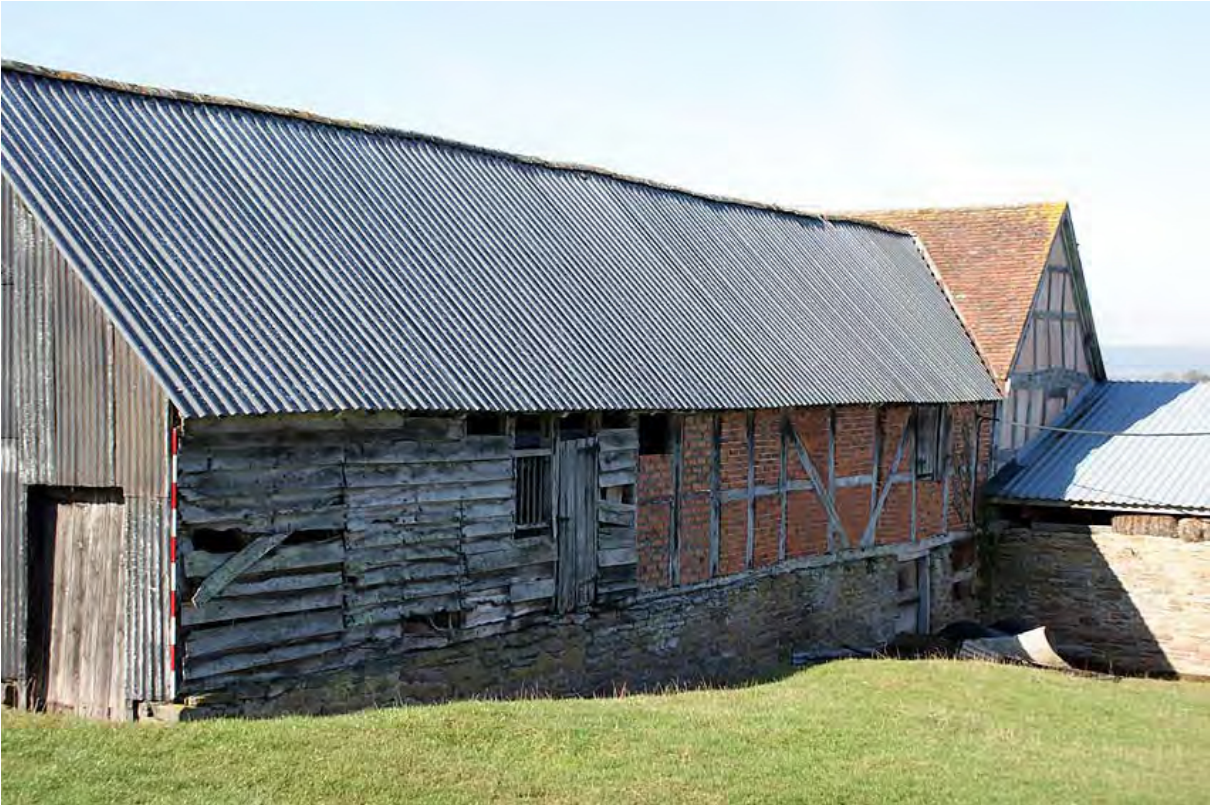
Plate 21: Buildings D, C and B from the south east
