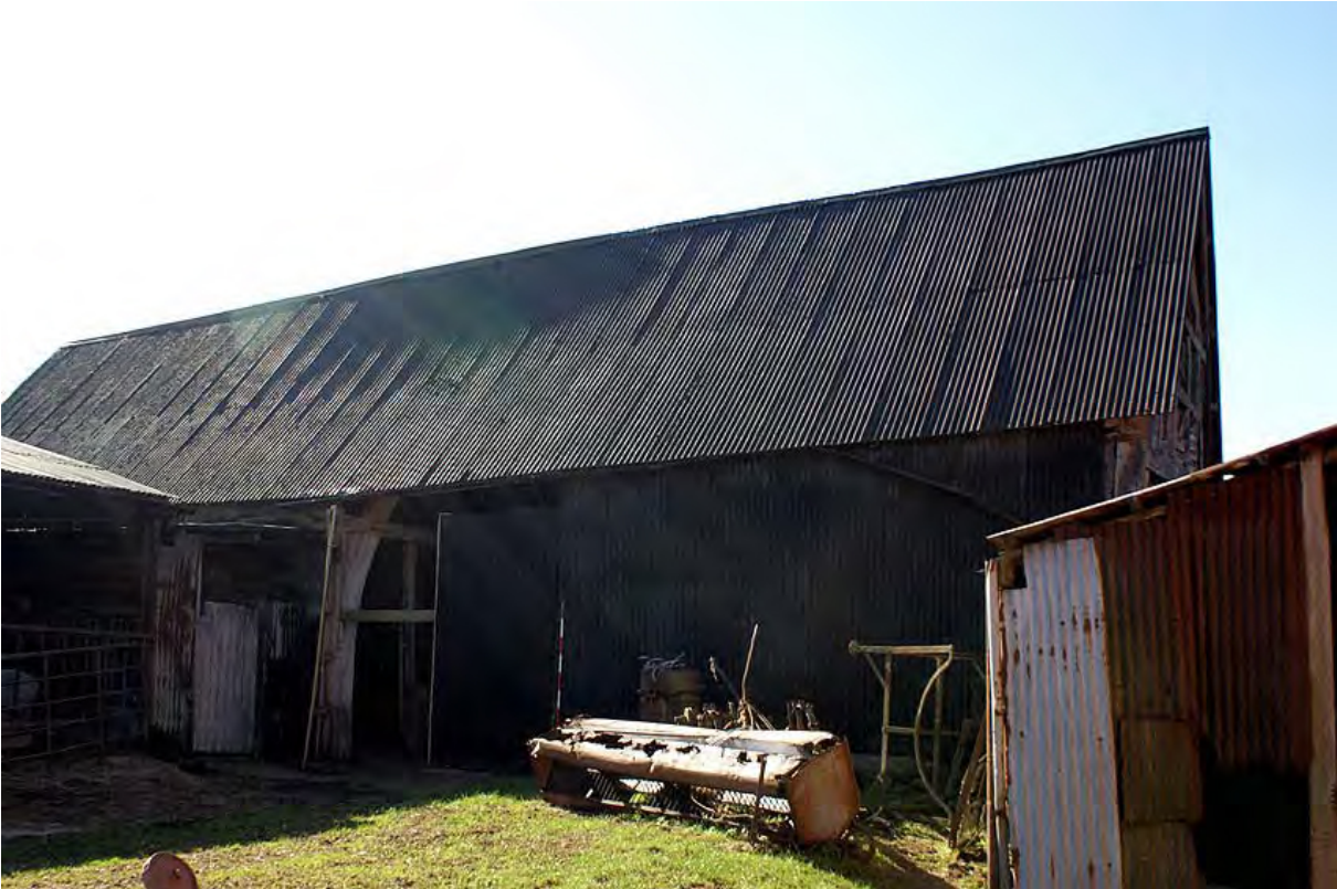
Plate 13: Building G from the north east
