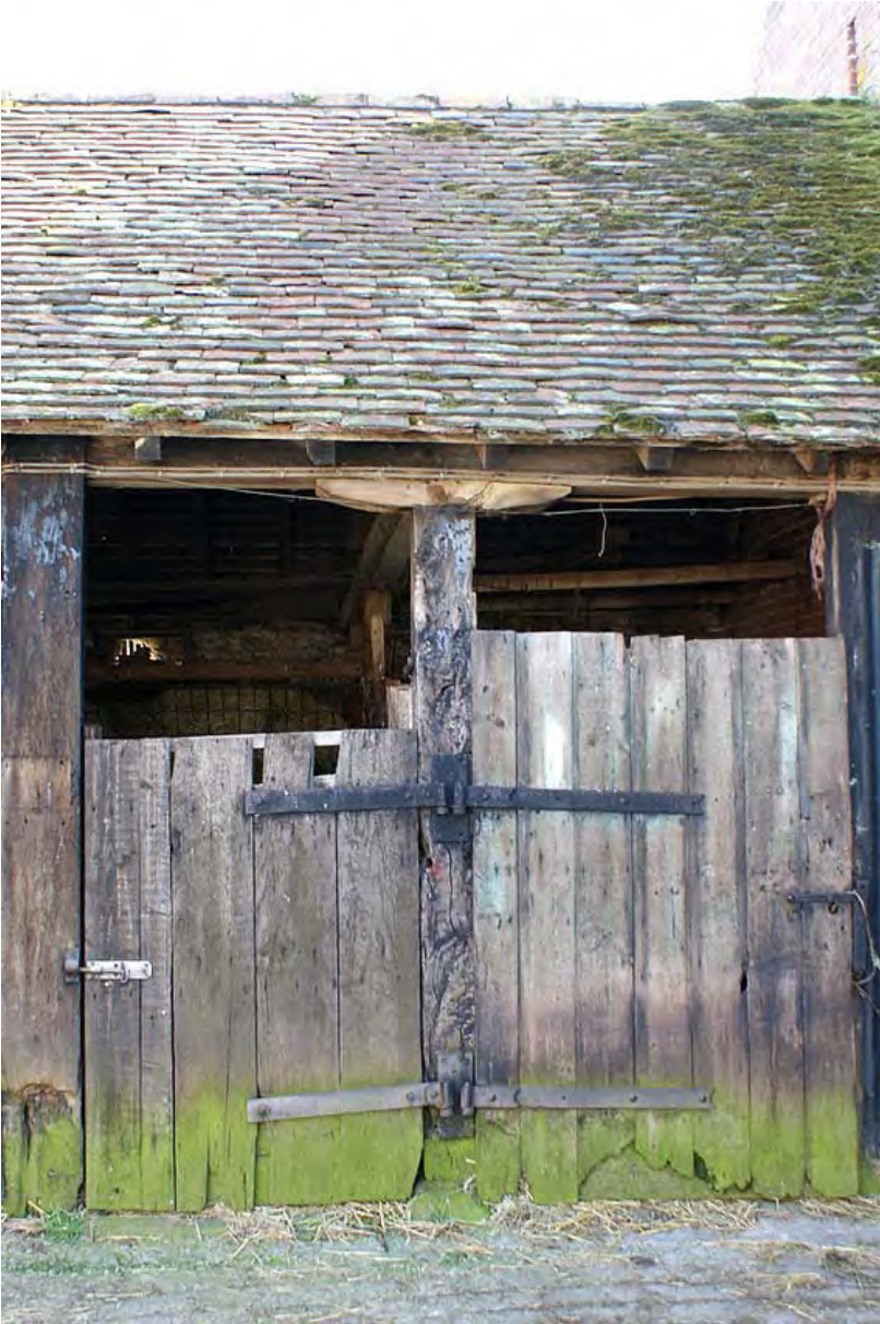
Plate 32: Building E, shelter shed post from the north west
