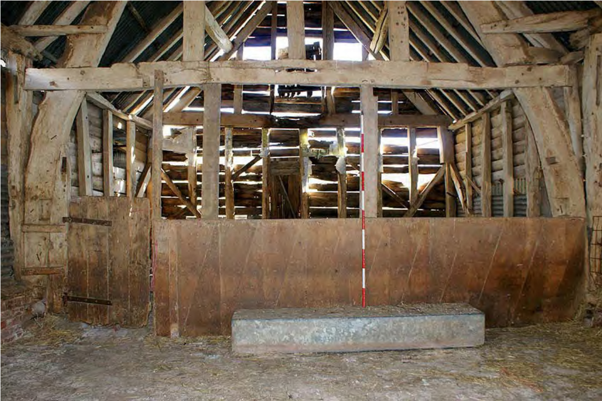
Plate 12: Building G cruck blades showing elements of re-use
