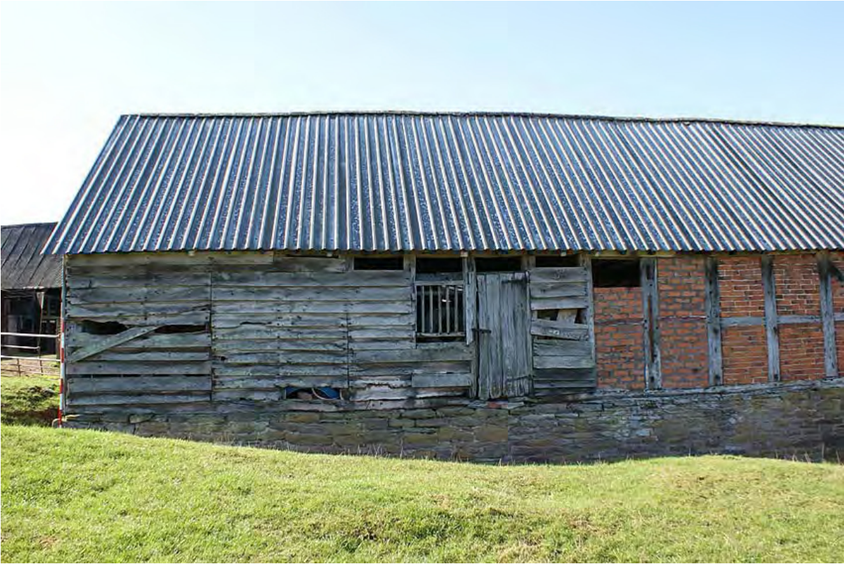
Plate 6: Building D from the north east
