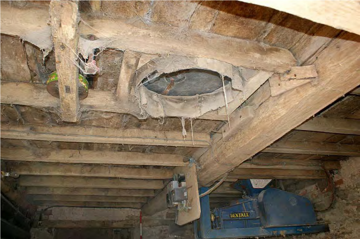
Plate 19: Building B lower ground floor, grain hole
