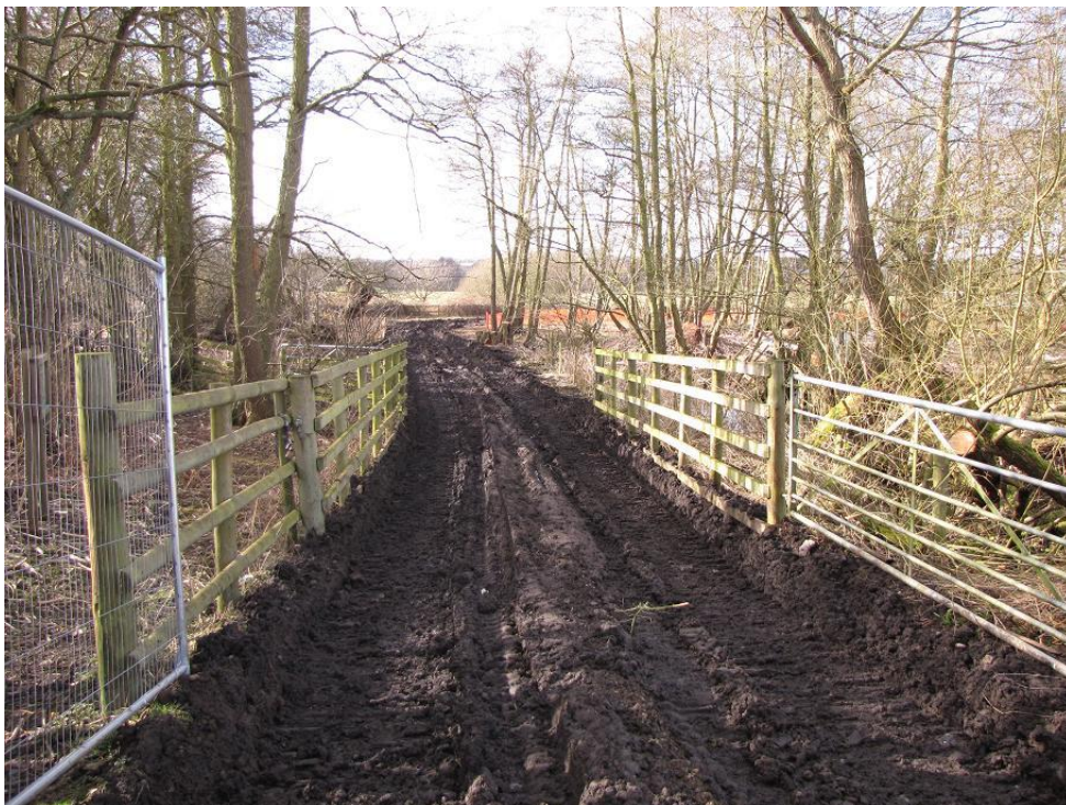
Plate 6 Southern Access road (Trench 4); looking west
