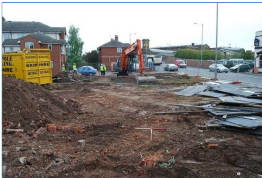
Plate 1 The site overall during initial ground reduction looking north-west
