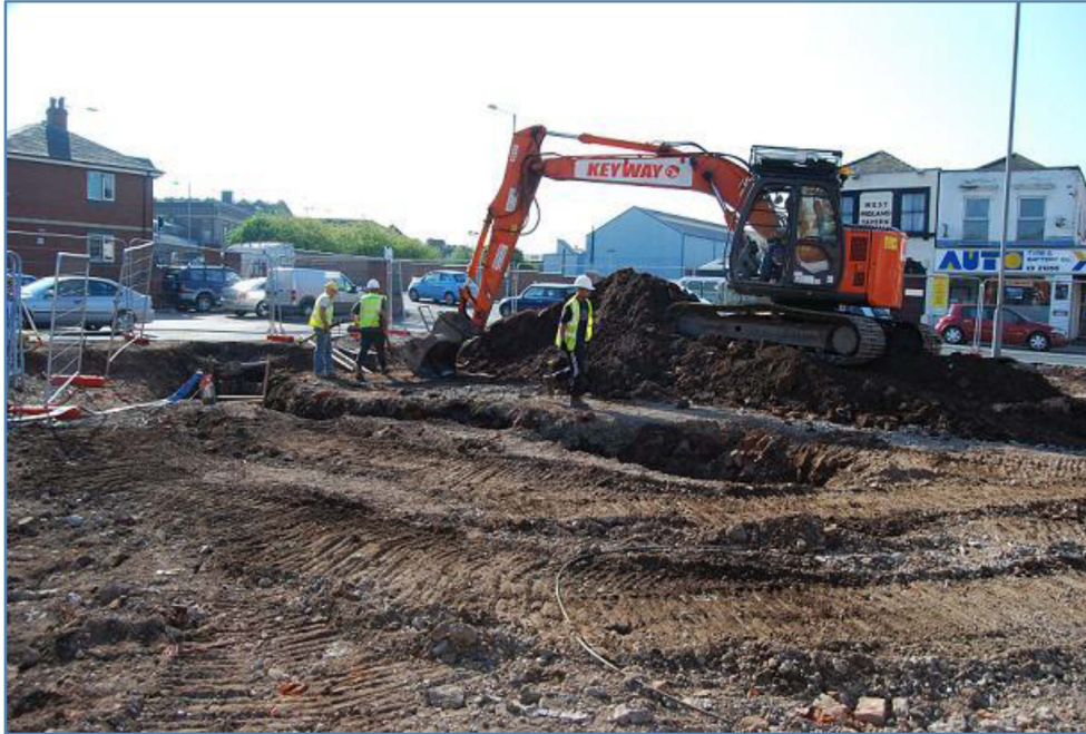
Plate 7 The drainage trench (Trench 2) after excavation, looking south-east
