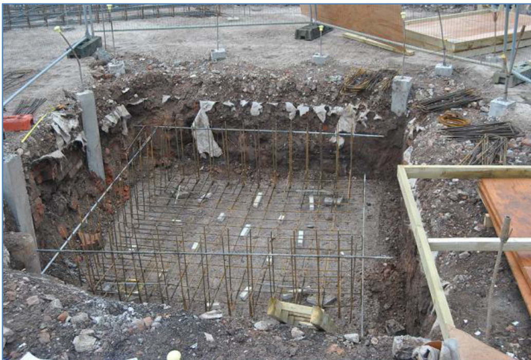
Plate 12 The lift shaft (Trench 3) looking north-west
