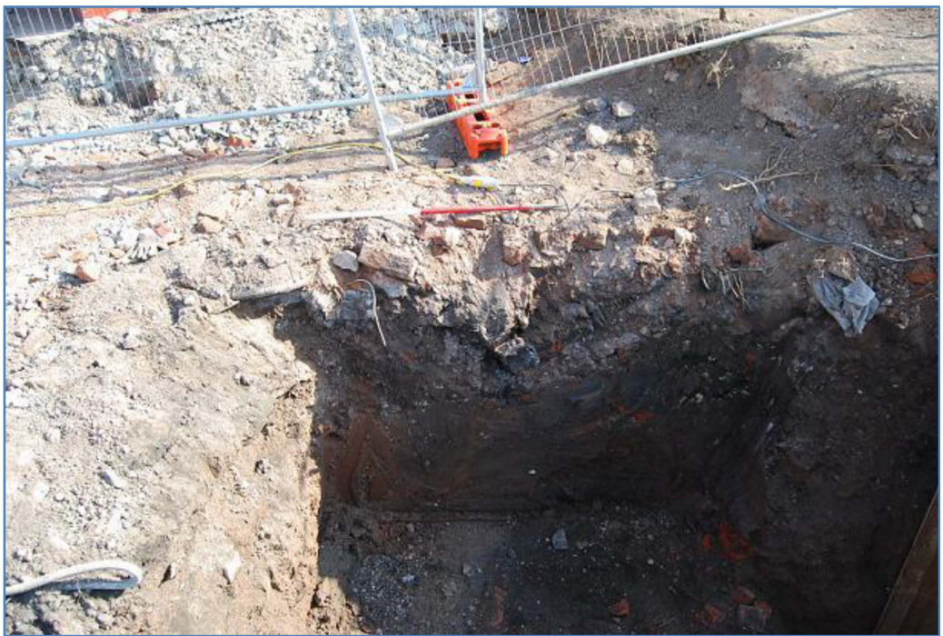
Plate 10 South facing section of eastern manhole of Trench 2
