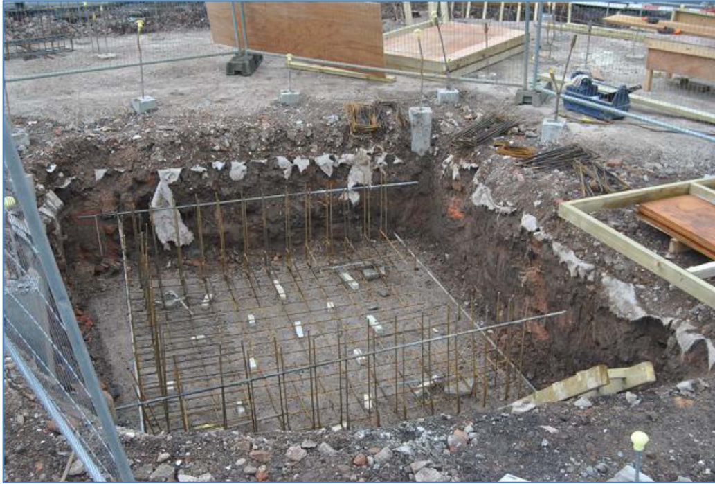
Plate 11 General shot of lift shaft (Trench 3) looking west
