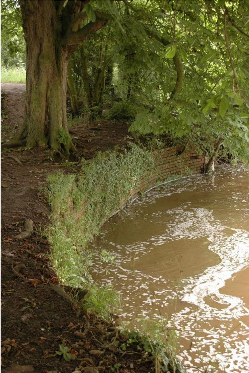
Plate 6 The bowl below Mill Weir, looking south
