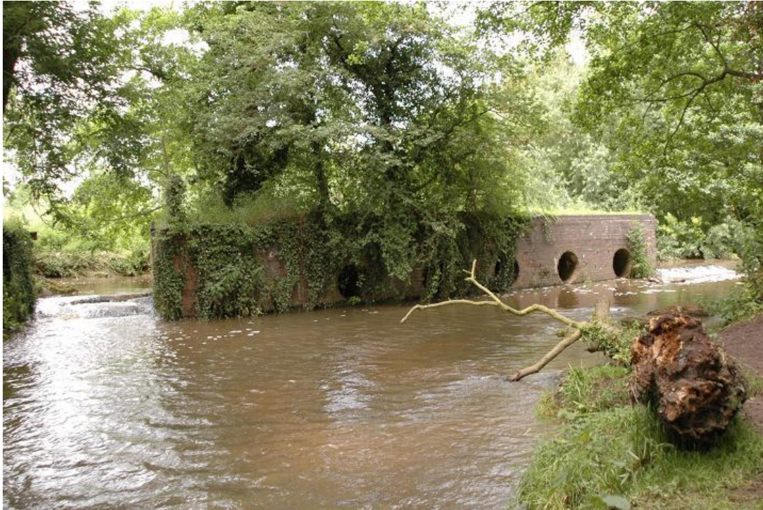
Plate 1 Five Tunnels Weir from the south-west
