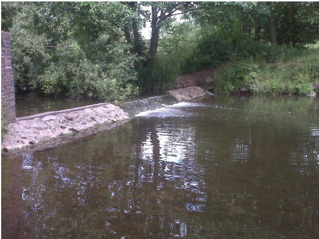
Plate 2 The east side of Five Tunnels Weir, from the south-west
