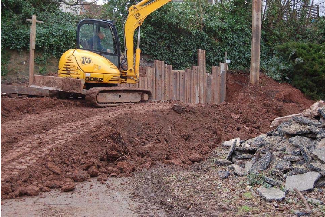
Plate 1: Installing the shoring in trench 1 to retain bank.
