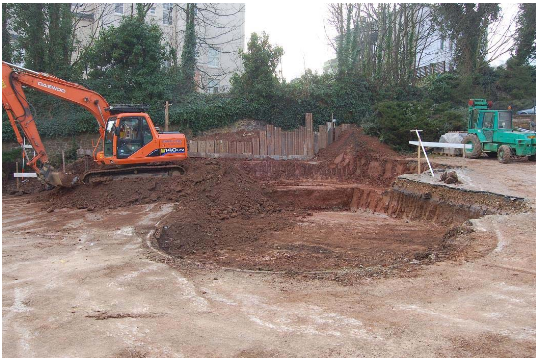
Plate 2: General shot showing the stripping of trench 2
