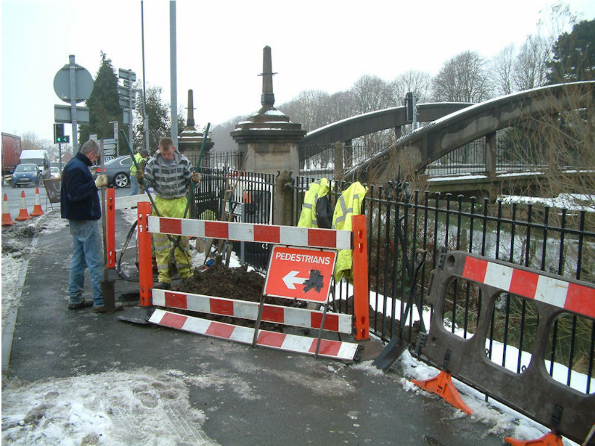
Plate 4, General location of Trench 2 during excavation, view west
