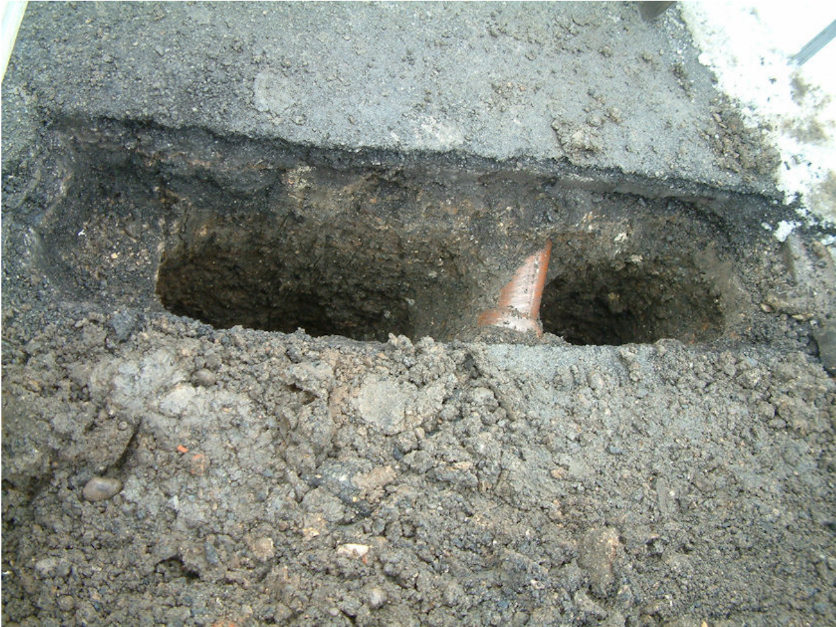
Plate 5 Trench 2 showing tarmac with modern disturbance beneath, view north
