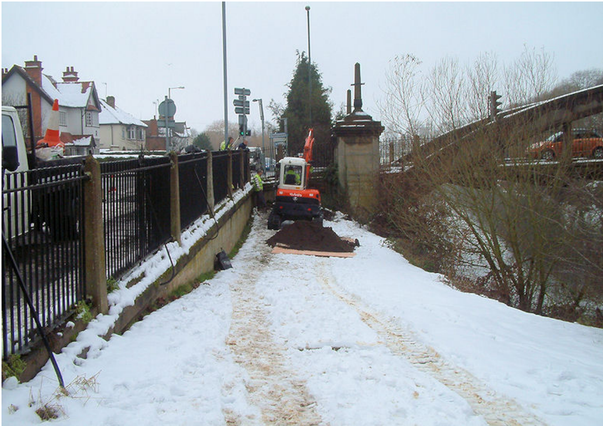
Plate 7, Excavation of Trench 3, with Abbey Bridge in the background, view west
