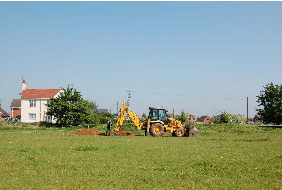
Plate 1 Excavation of Trench 2, facing north.
