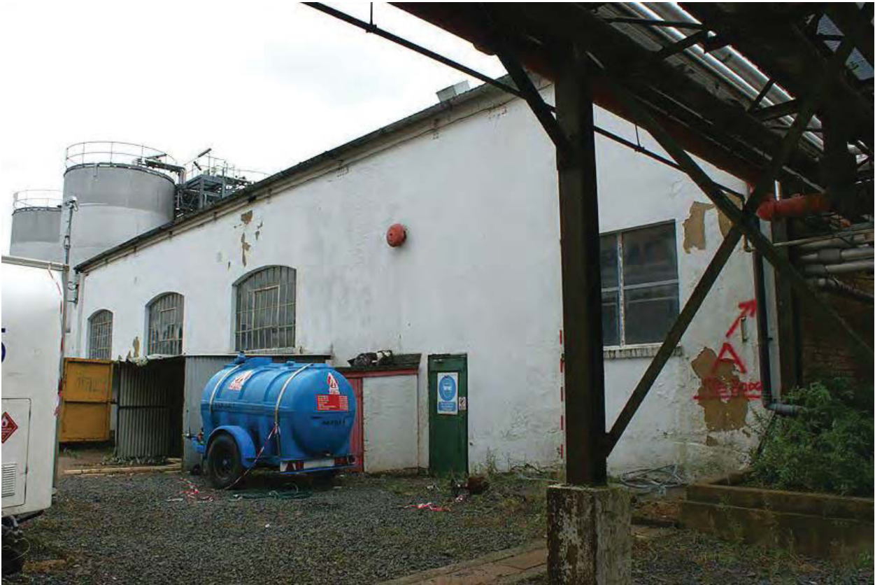
Plate 7: Building B north west elevation
