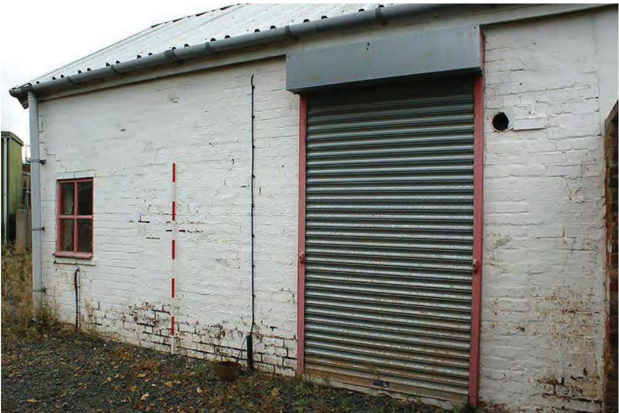
Plate 2: Building A north east elevation
