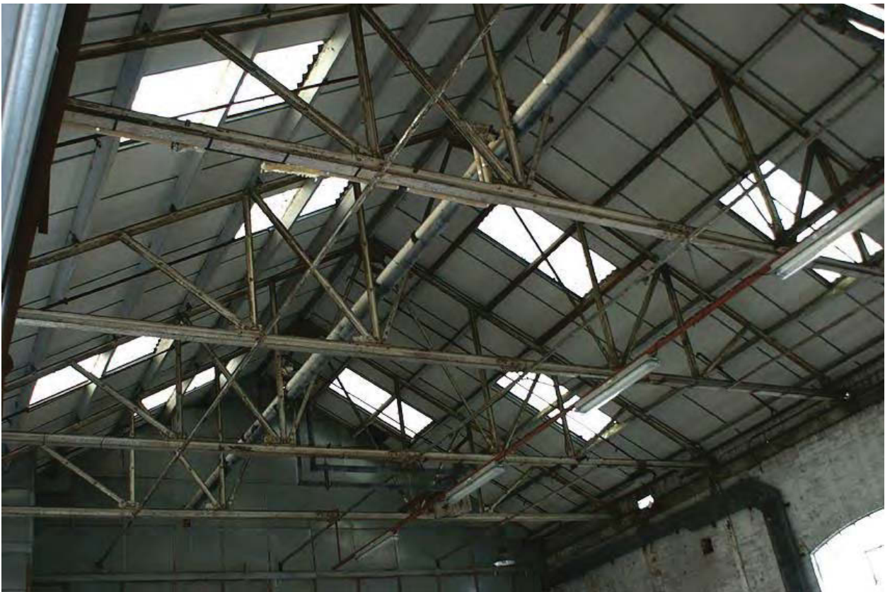
Plate 10: Building B metal trusses
