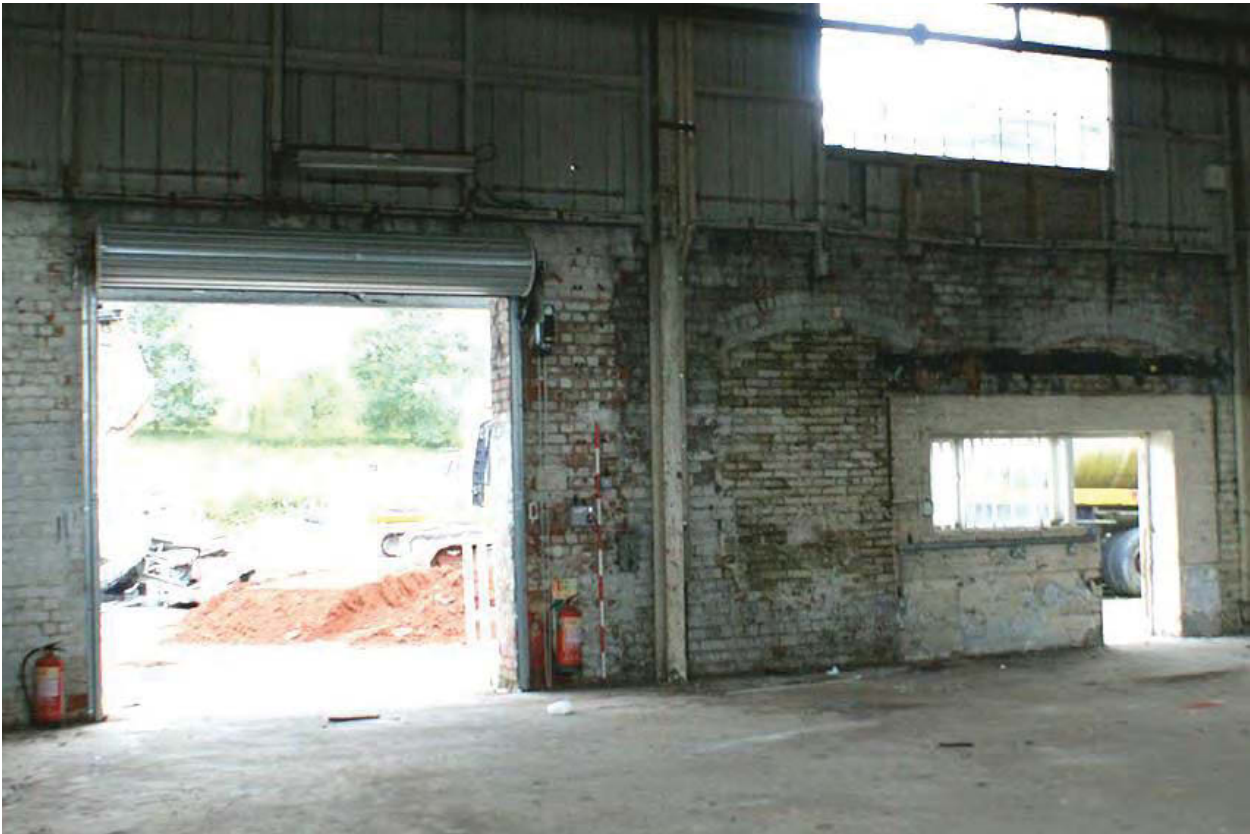
Plate 23: Building B, south east elevation showing inserted openings and blocked windows
