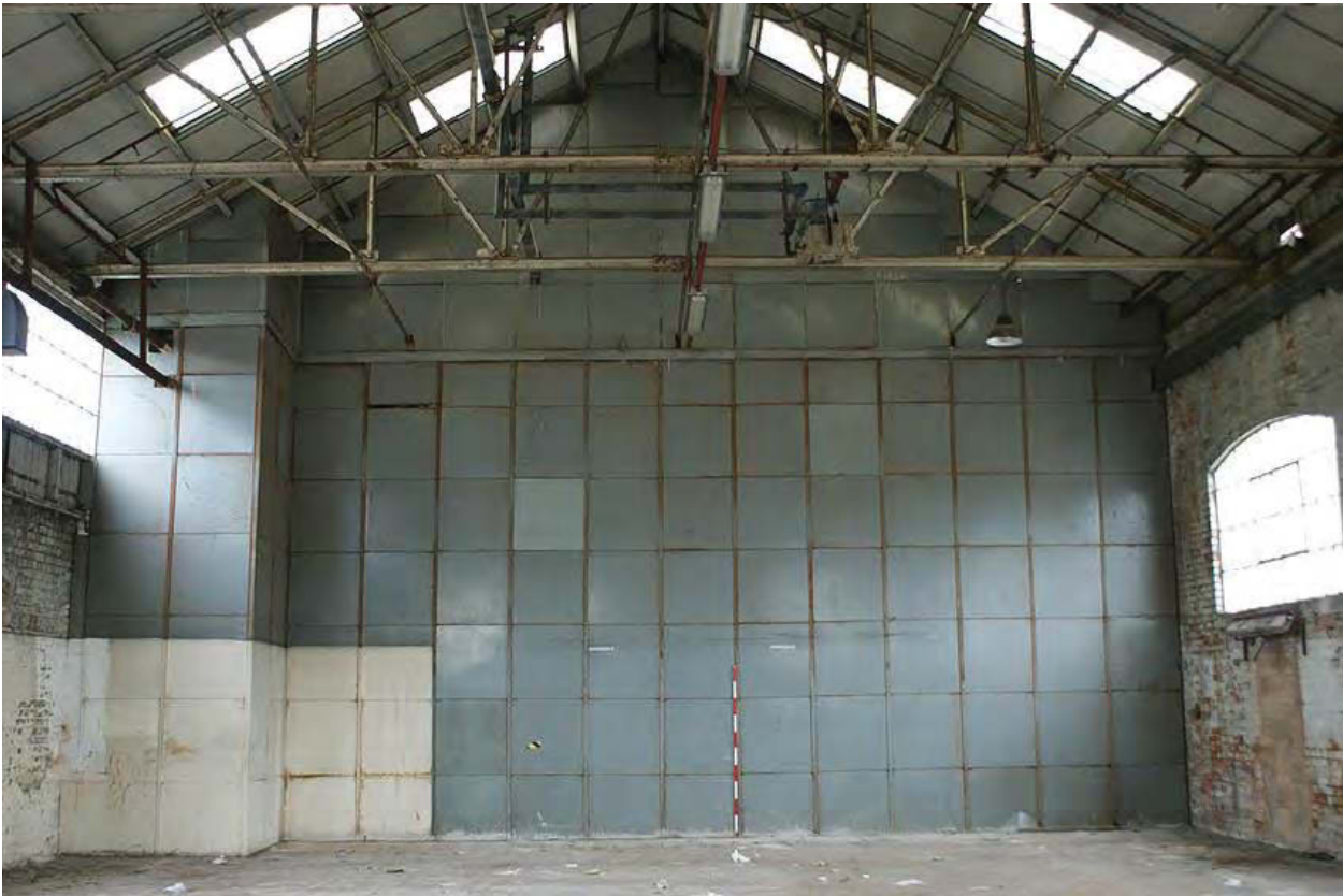
Plate 20: Building B, inserted metal partition
