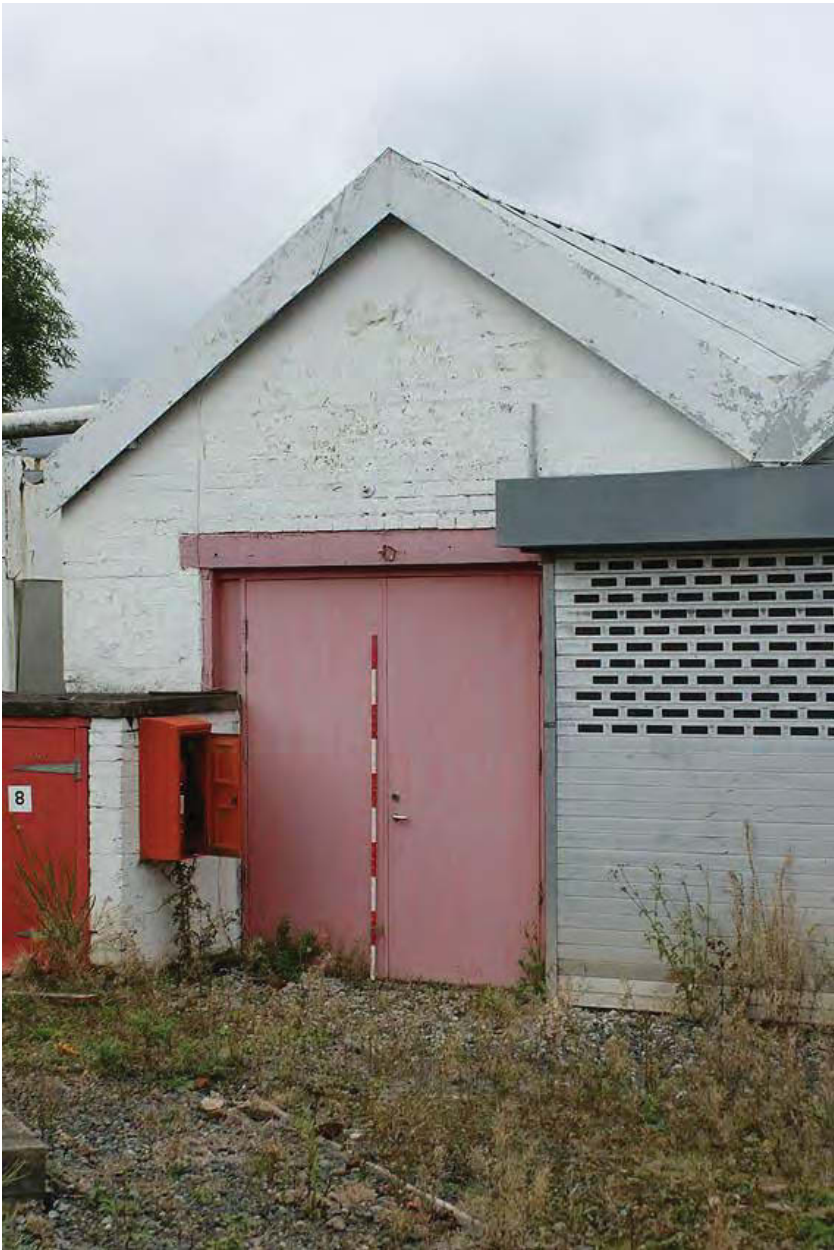
Plate 19: Exterior of Building A, south east elevation inserted doors
