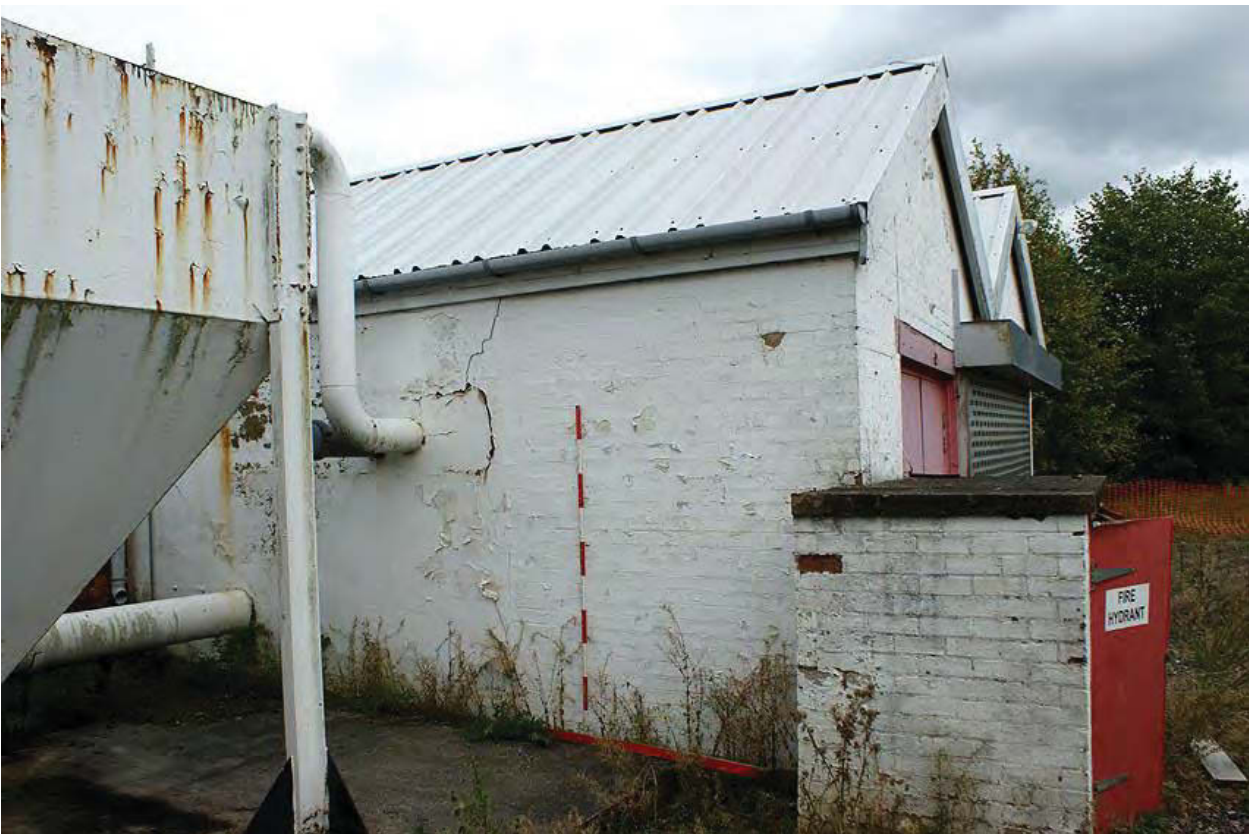
Plate 4: Building A south west elevation
