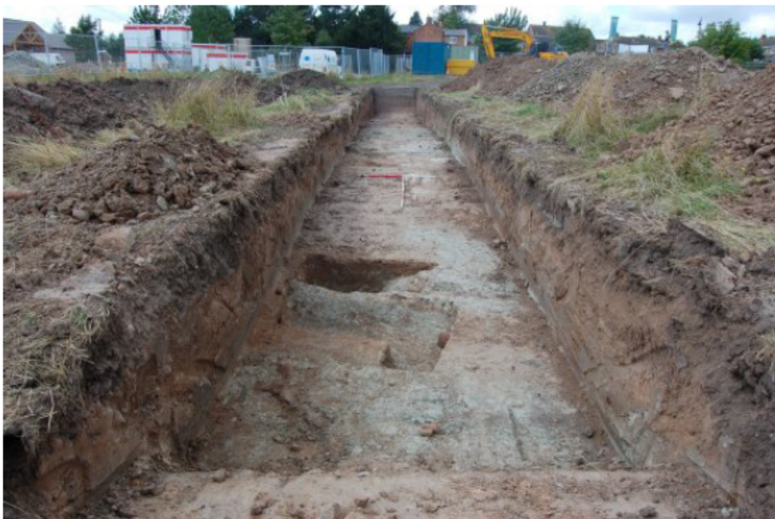
Plate 18: Trench 12, general view. (Facing west)
