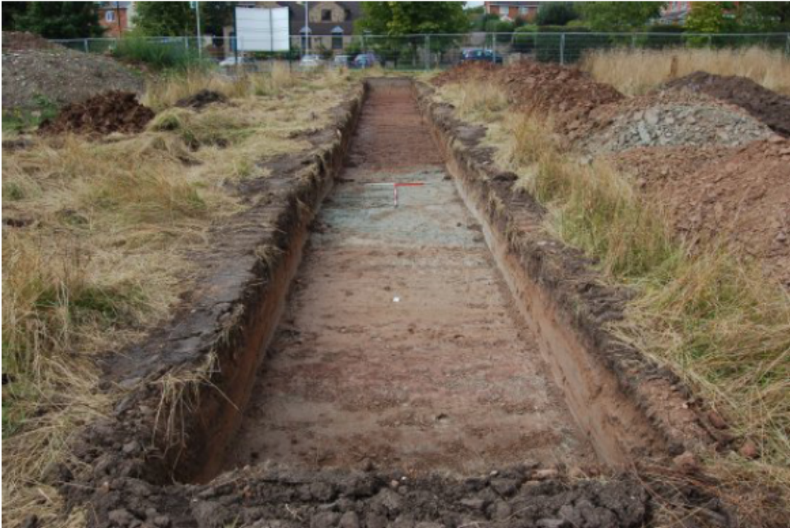
Plate 9: Trench 8, general pre-excavation view. (Facing west)
