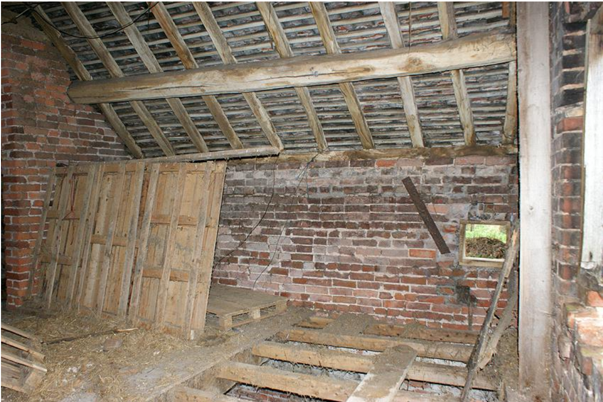
Plate 13: Upper floor of Building 1
