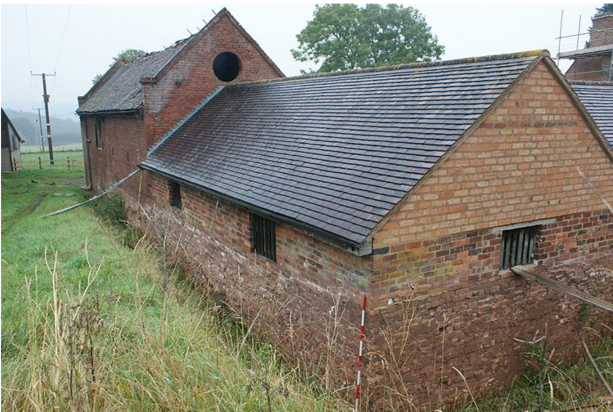
Plate 8: Building 2 from the north west
