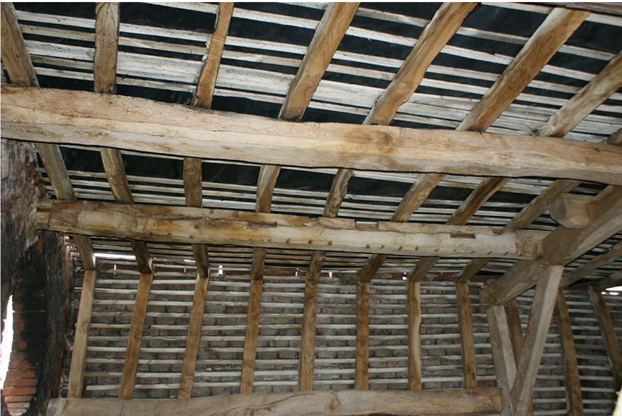
Plate 11: Reused timber in the roof of Building 1
