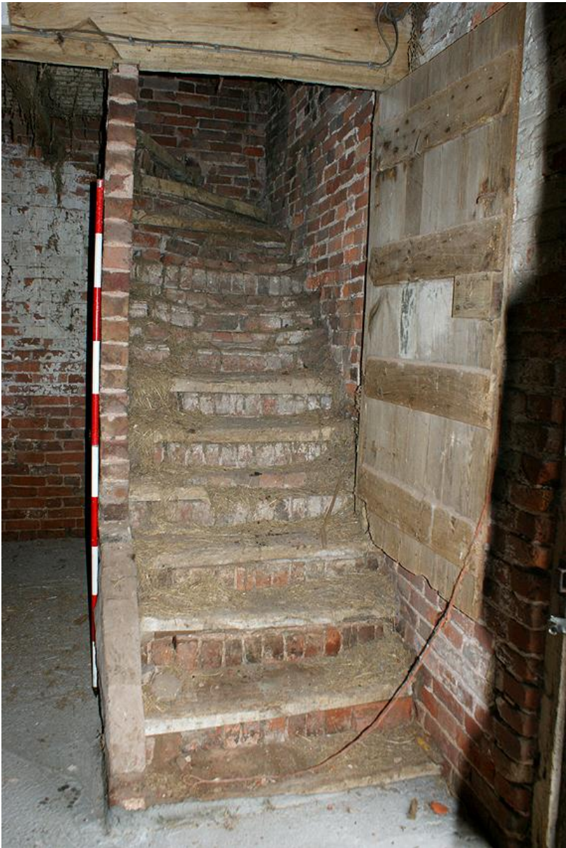
Plate 12: Staircase to first floor in Building 1
