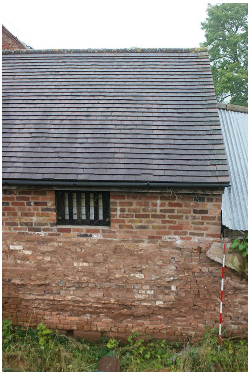
Plate 9: North wall of Building 2 showing reused sandstone
