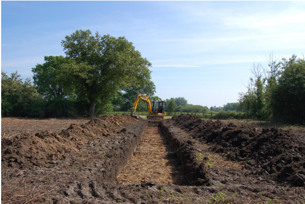
Plate 1: General view of the trench, facing east
