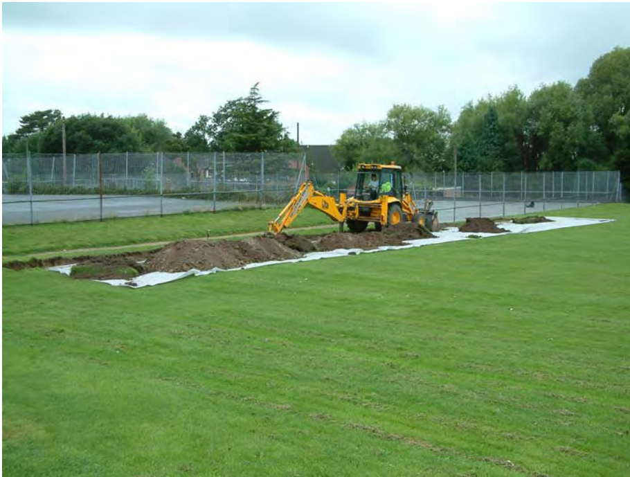
Plate 3: Trench 2, machine excavation in progress, view north-west
