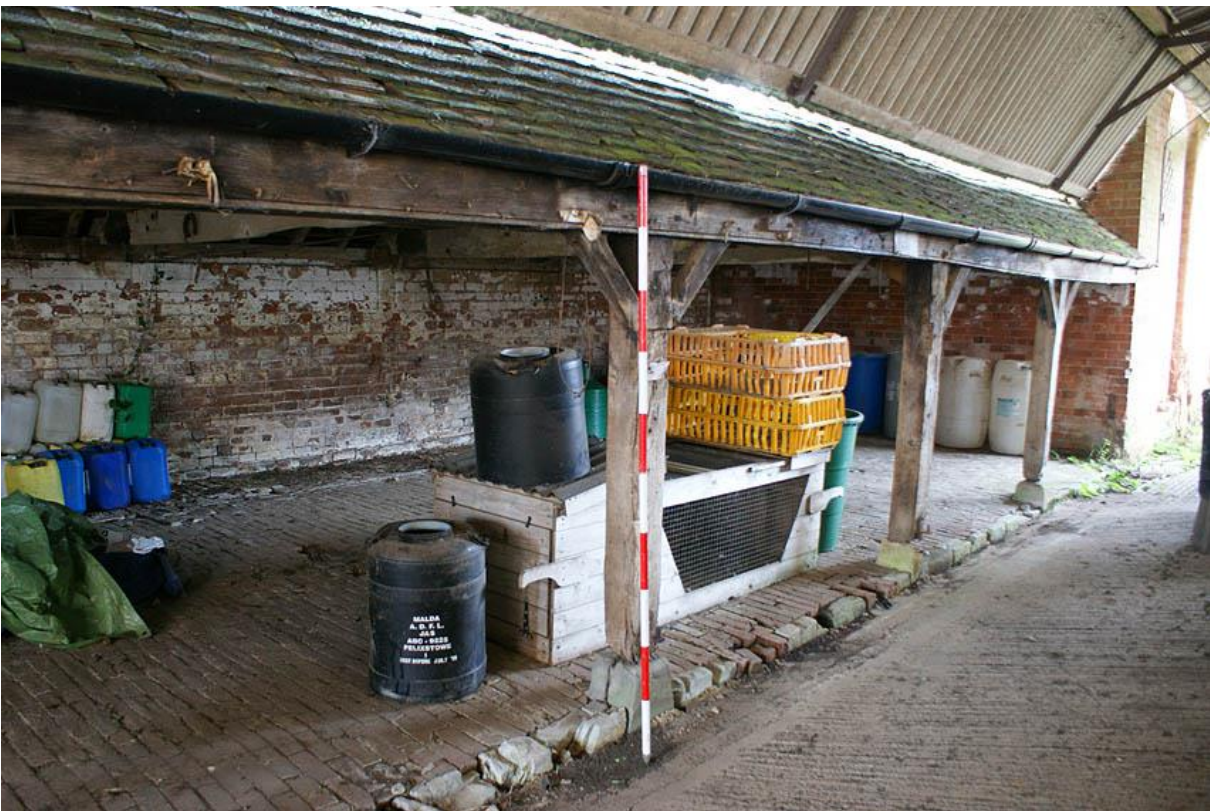
Plate 2: Unit 1 shelter shed from the south east
