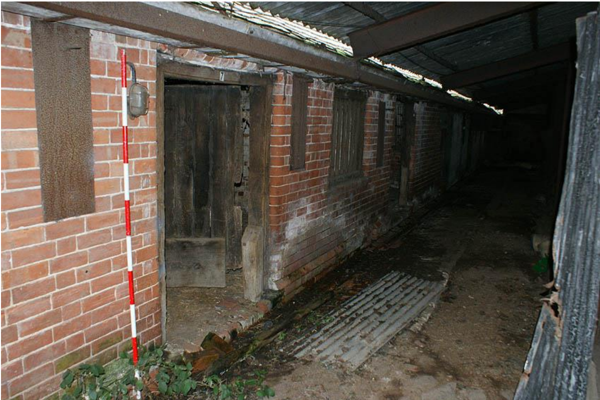
Plate 5: Unit 1 stables from the west
