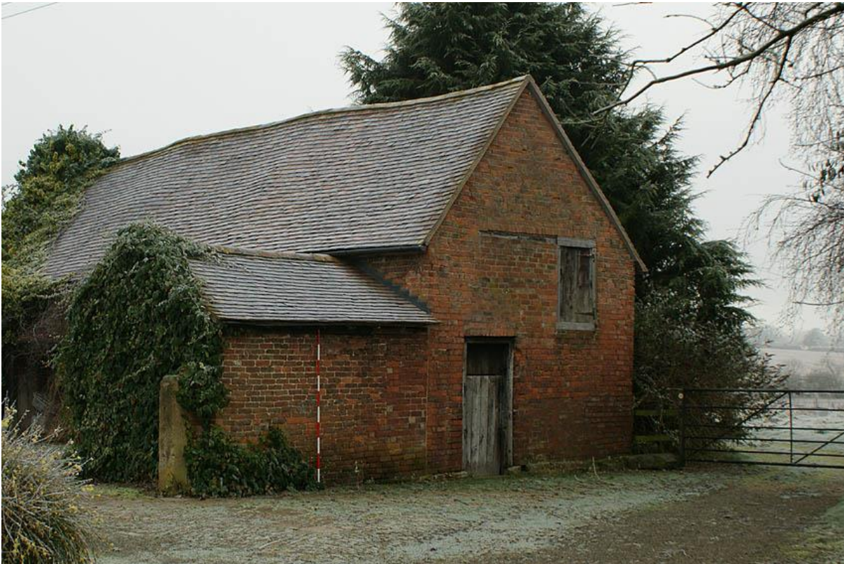
Plate 14: Unit 6 timber frame structure showing brick extensions and possible 17 th century brick wall on the left
