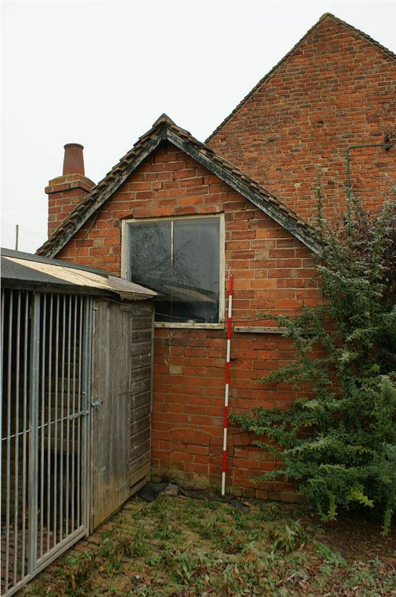
Plate 10: Units 3 and 4 farmhouse hen house extension
