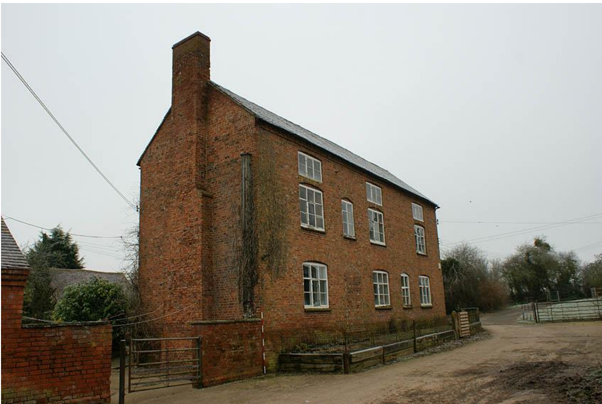
Plate 8: Units 3 and 4 farmhouse from the east
