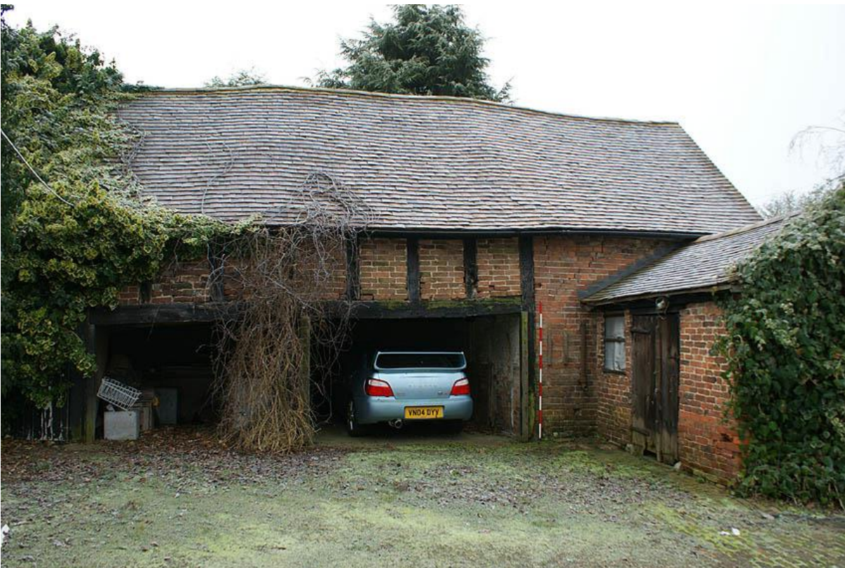
Plate 13: Unit 6 timber frame structure from the north east
