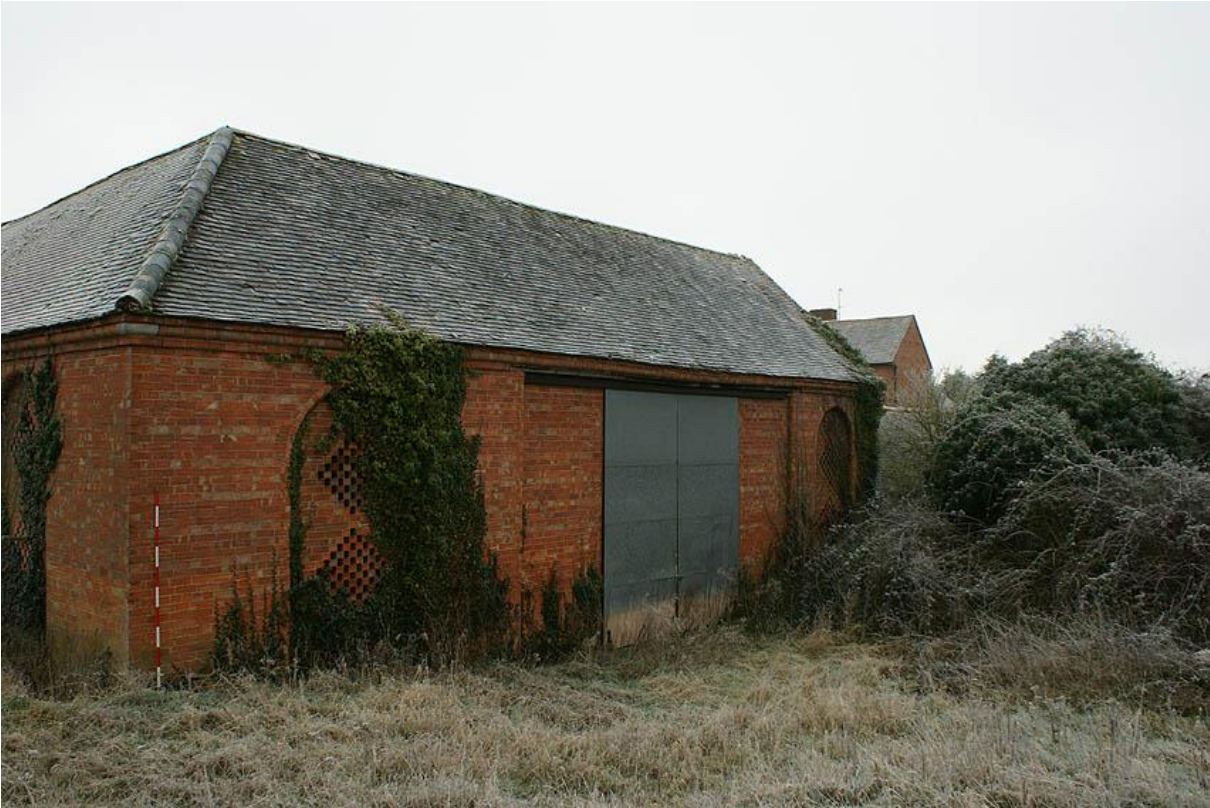
Plate 3: Unit 1 threshing barn from the north west
